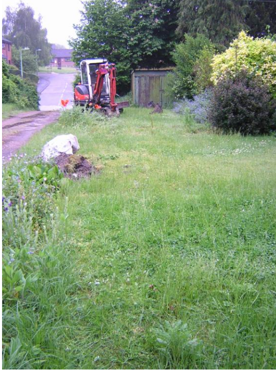
Plate 1. Pre-excavation TR1 , from the north-west
