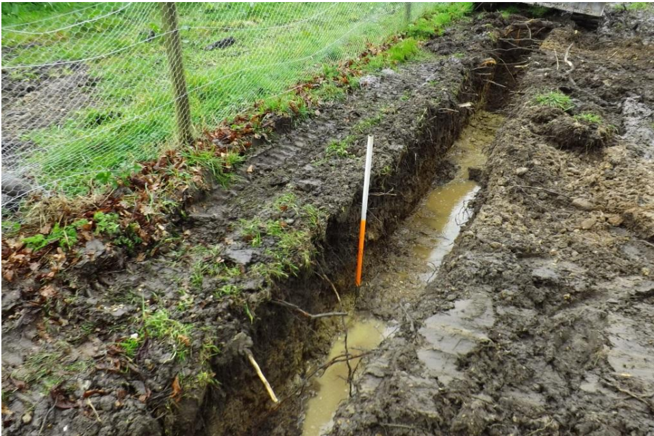
Plate 2. Section of french drain trench, looking south-east
