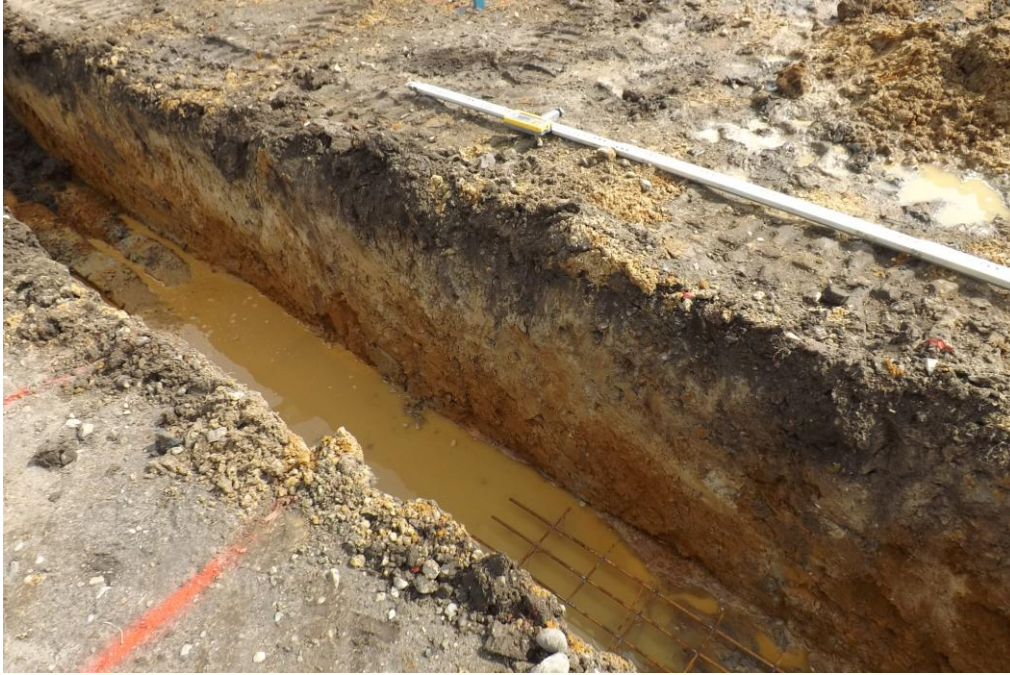
Plate 7. Section of footings trench (plot 2), from the south-west
