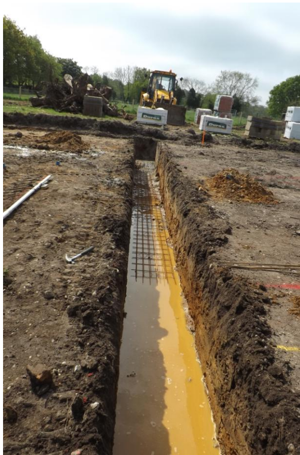
Plate 8. Footings trench (plot 2) from the north
