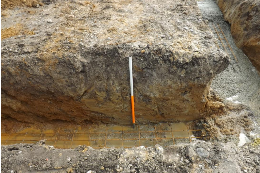
Plate 5. Section of footings trench, plot 1, from south
