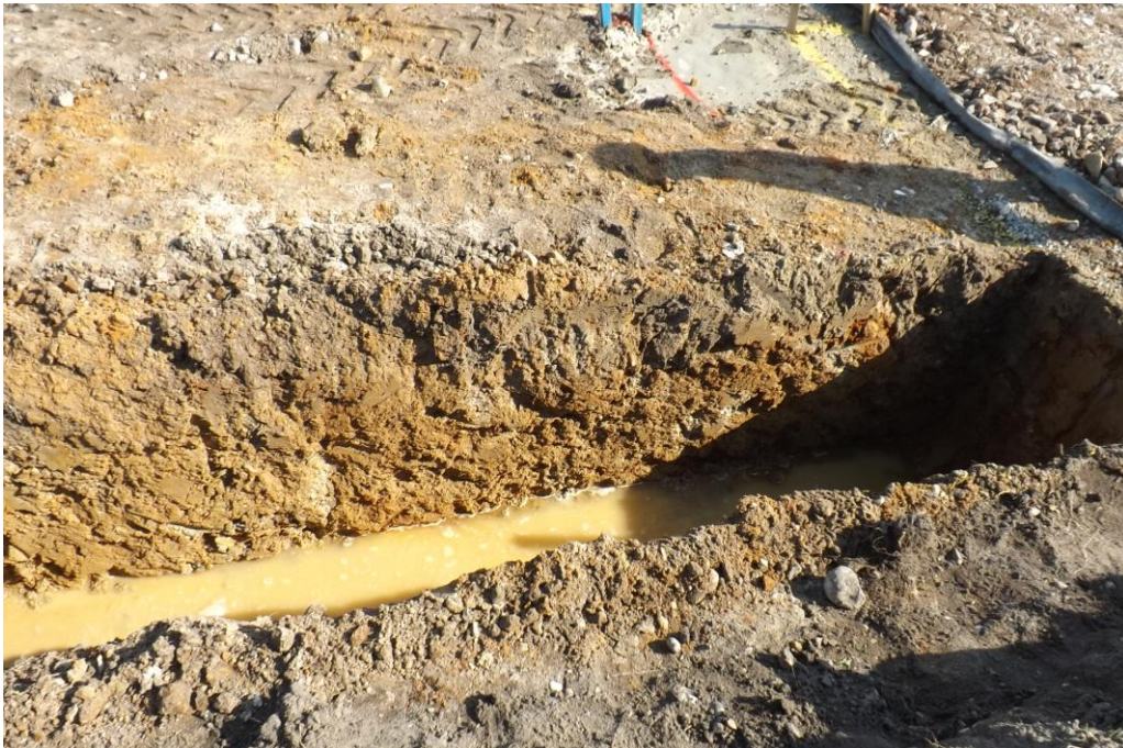
Plate 4. Section of footings trench, plot 1, from the west
