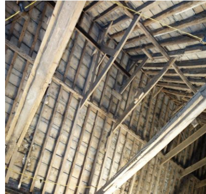
Plates 17 & 18 Roof bracket assemblies for hoists
