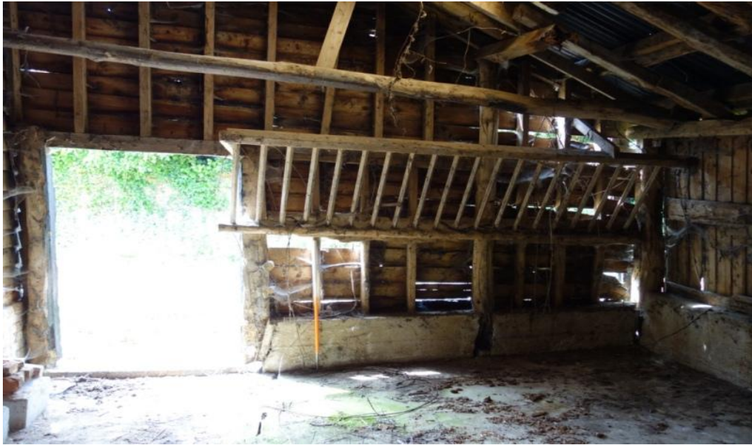
Plate 32. Lean-to detail used as a stable showing the wooden feeding rack from the north-east
