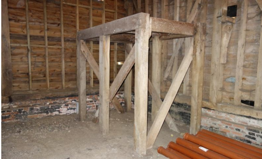
Plate 22. Wooden cradle to support a tank or hopper
