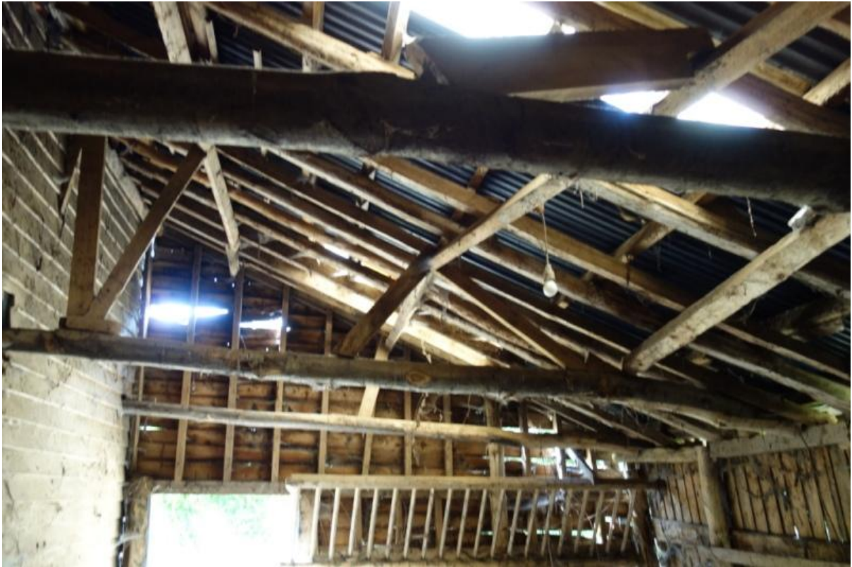
Plate 34. roof detail of lean-to (stable) from the north
