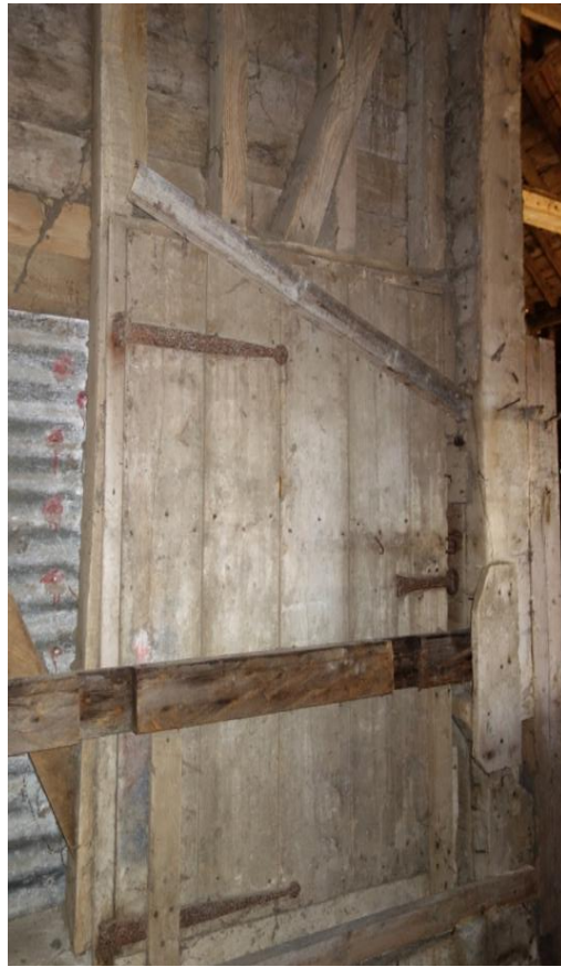
Plate 26. Door detail to side of porch from the south-west
