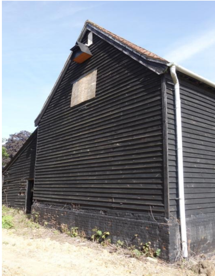
Plate 3. Barn gable end wall from the south
