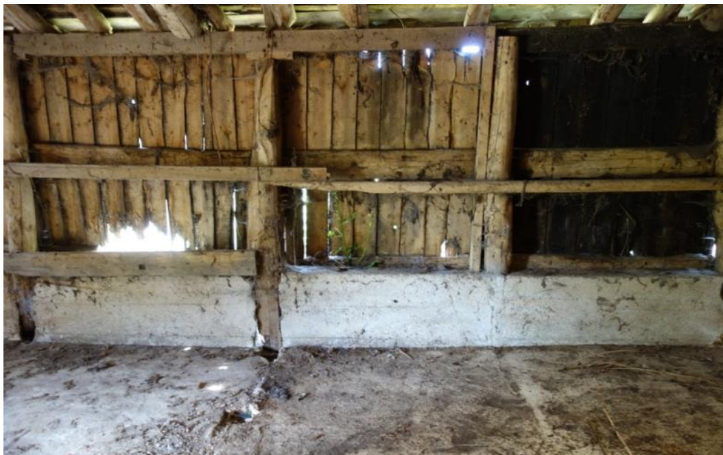
Plate 33. Tethering rail to west-facing elevation wall of lean-to
