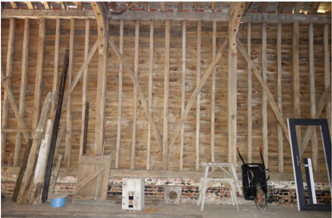
Plate 21. Studwork detail rear elevation wall from the north-west
