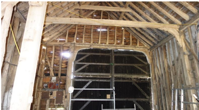
Plate 24. Roof detail of porch, vertical
