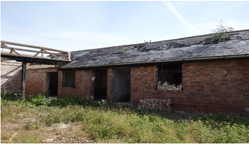
Plate 9. Stables from the south-west
