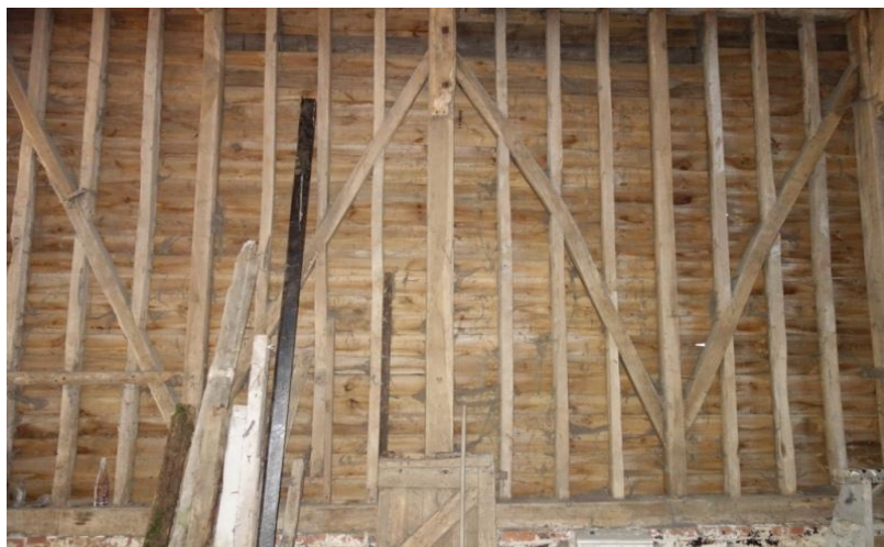
Plate 29. Detail of studwork to rear wall from the west
