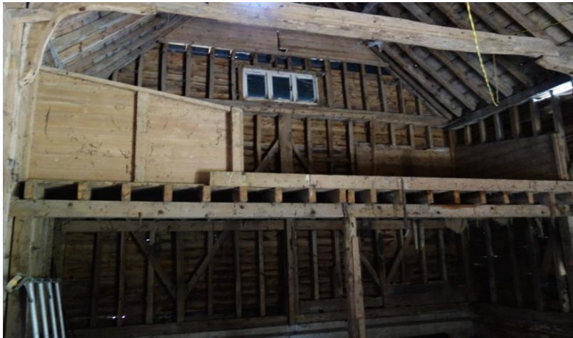
Plate 28. Hay loft from the south-west
