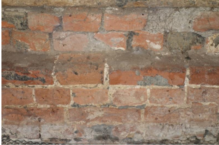
Plate 27. Brick plinth detail to north-east corner of barn
