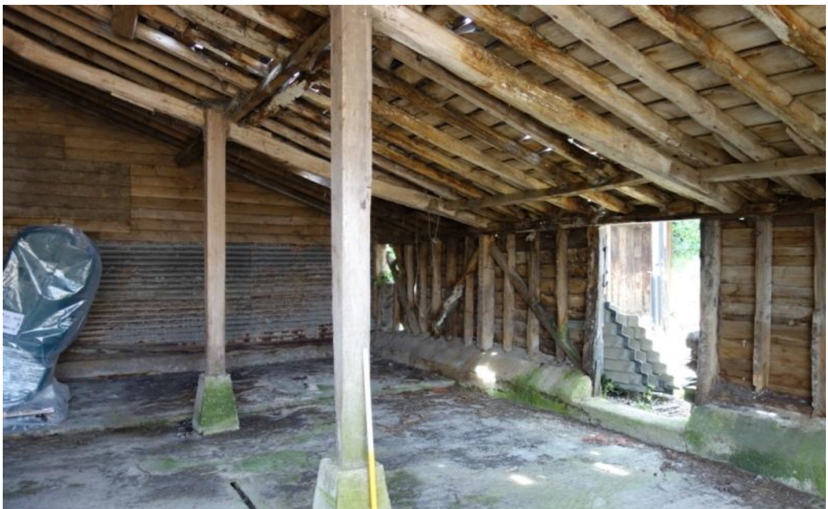
Plate 35. Interior view of northern lean-to (storage room)
