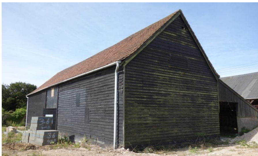
Plate 7. Barn exterior from the north-east
