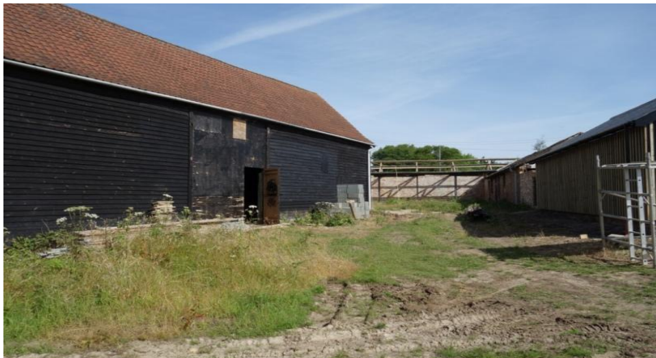
Plate 2. Stables exterior from the south
