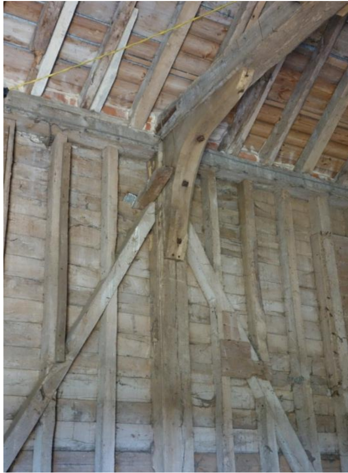
Plate 14. Bolted knee brace detail from the south-east
