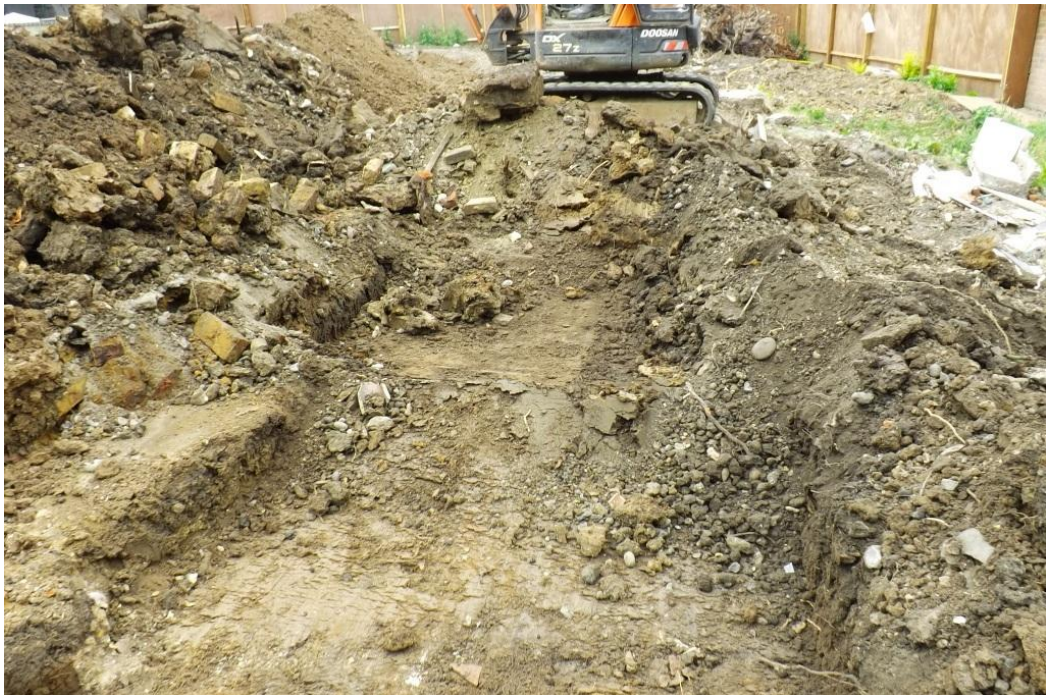
Plate 9. Trench 2 in progress showing over burden of demolition material
