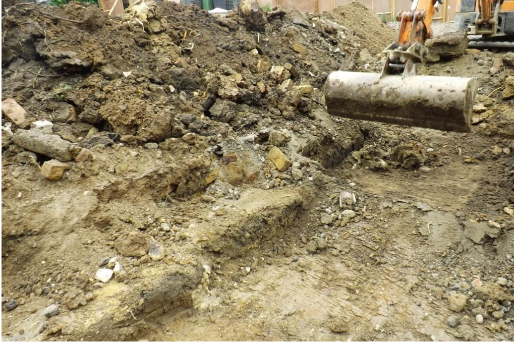
Plate 8. Trench 2 in progress showing over burden of demolition material
