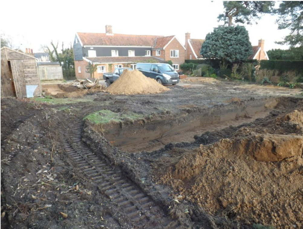
Plate 5. Post-excavation of site, from the south-west
