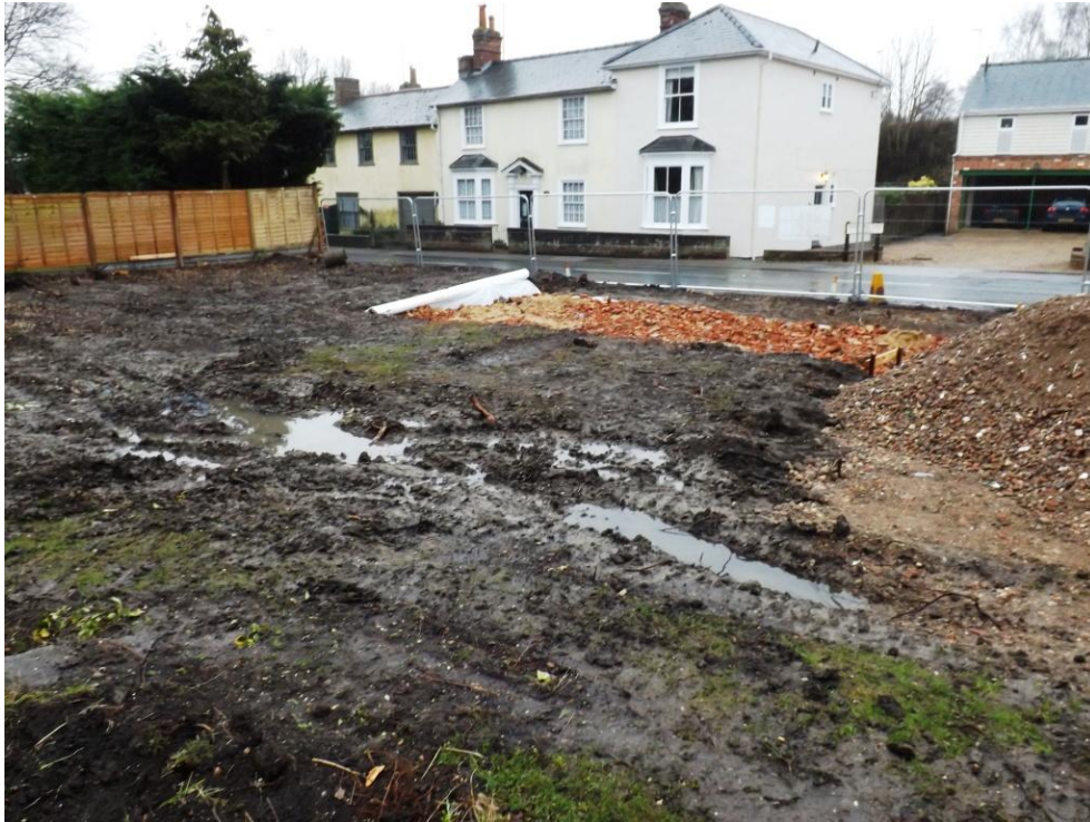
Plate 1. Pre-excavation of site, from the north-west
