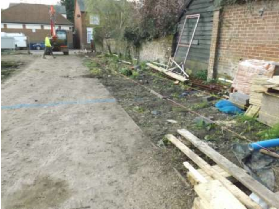
Plate 1. Pre-excavation from the north
