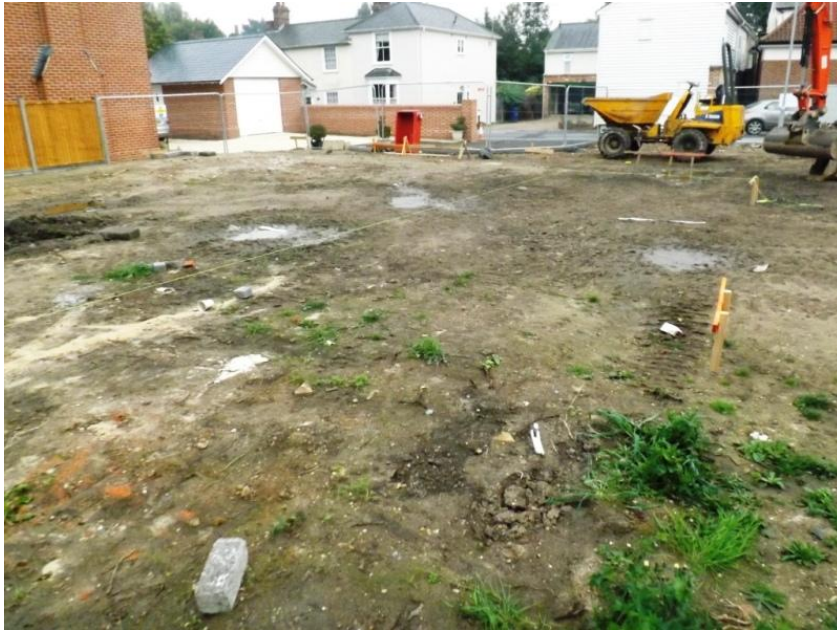
Plate 1. Pre-excavation of site
