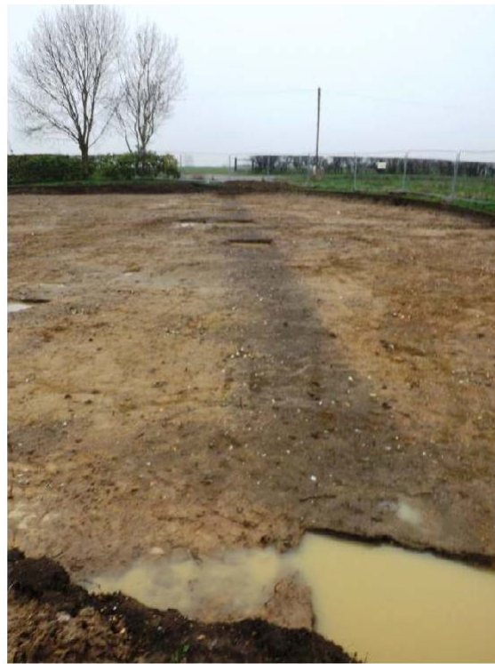
Figure 67. General view of building internal structure and boundary ditch from the south
