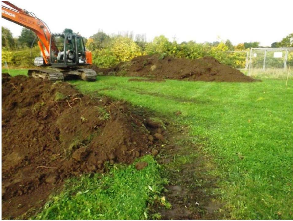
Figure 20. Pre-excavation, general view
