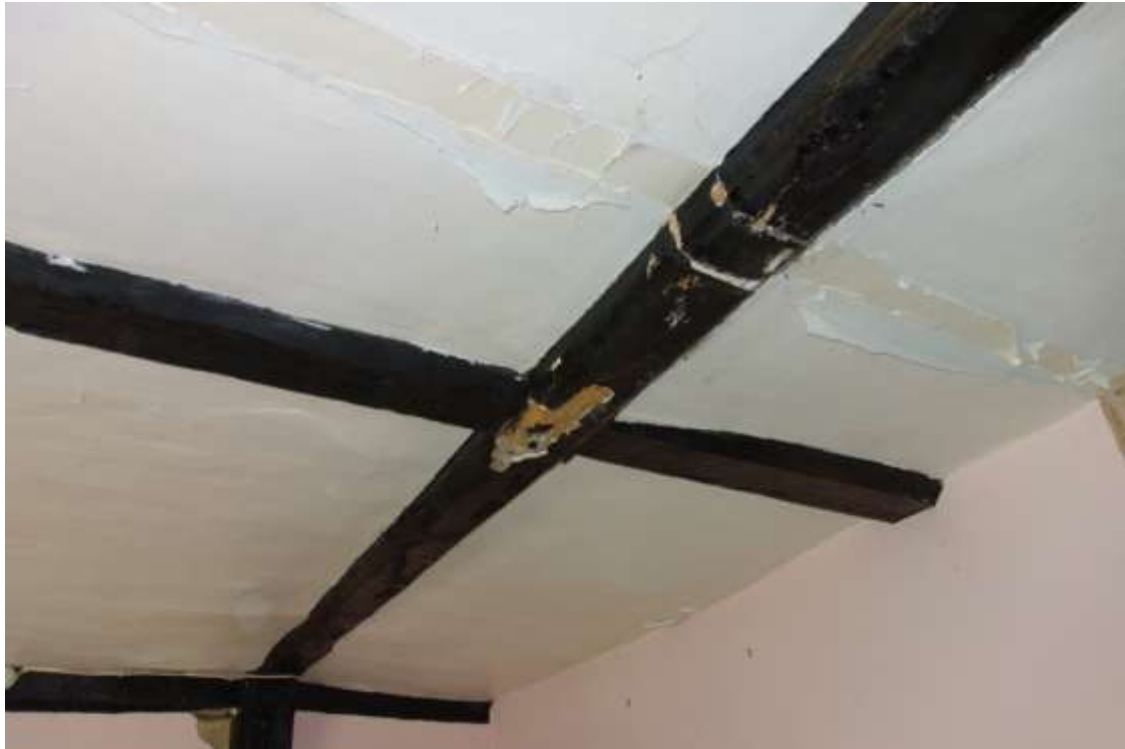
Plate 31. First floor cross-wing ceiling joist detail
