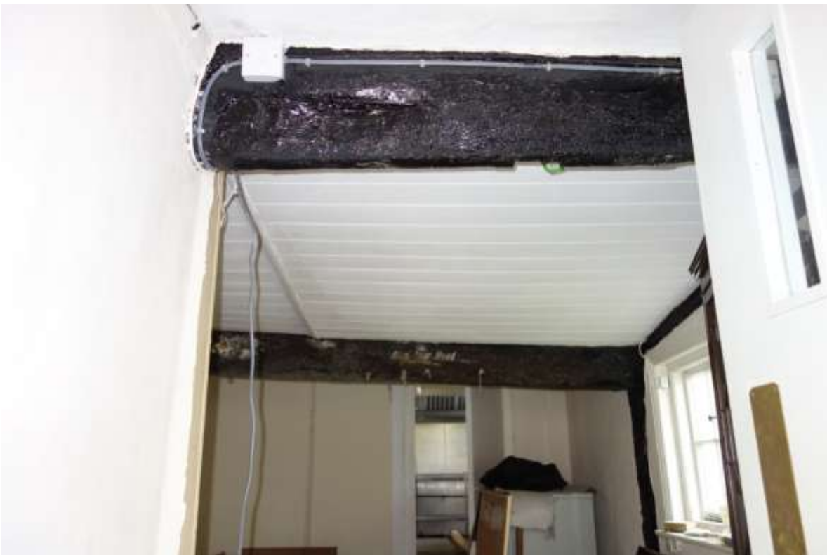
Plate 16. Joists in cell 1, phase 1 ground floor
