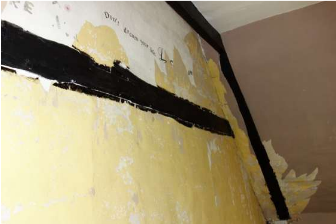
Plate 33. Partition wall of sub-divided room, first floor with tie-beam to roof truss over hall/lounge
