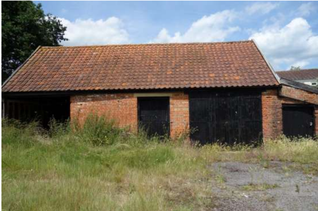
Plate 39. Nineteenth century cart shed from the south
