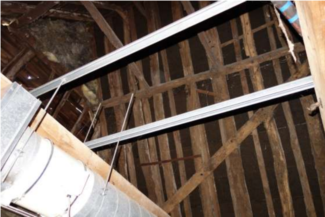
Plate 37. Roof detail over hall/lounge showing plain butt purlin and wind brace arrangement (late 17th century work)
