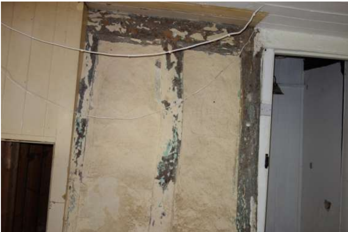
Plate 20. Exposed studwork detail to base of staircase in phase 1
