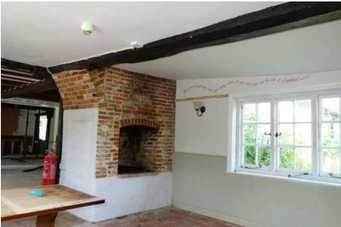
Plate 17. Fireplace/oven in phase 2, cell 2 (lounge), showing late Tudor brickwork, altered in the 18th century (note the dome-shape of the oven in the brickwork now filled in above the arch)
