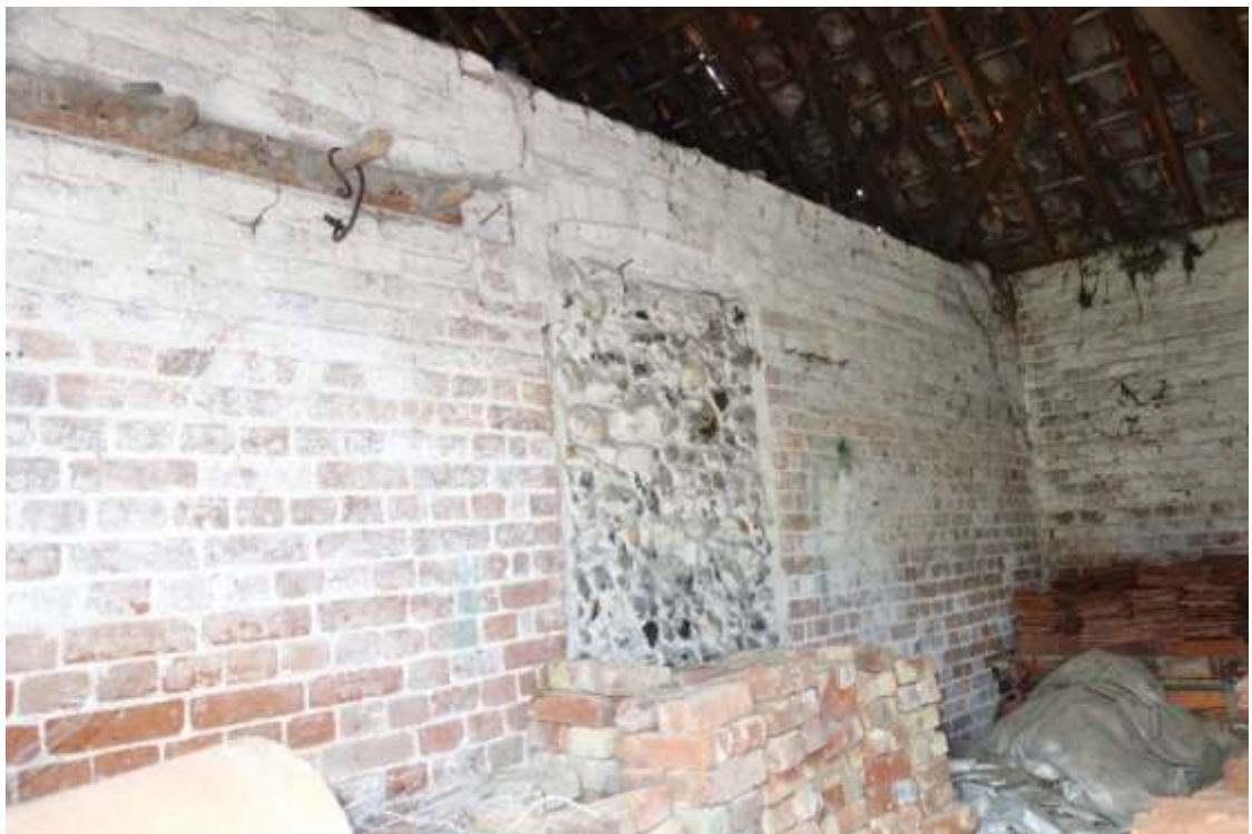
Plate 42. Blocked off doorway from open cell to central cell, note the wooden tack hook to the upper left
