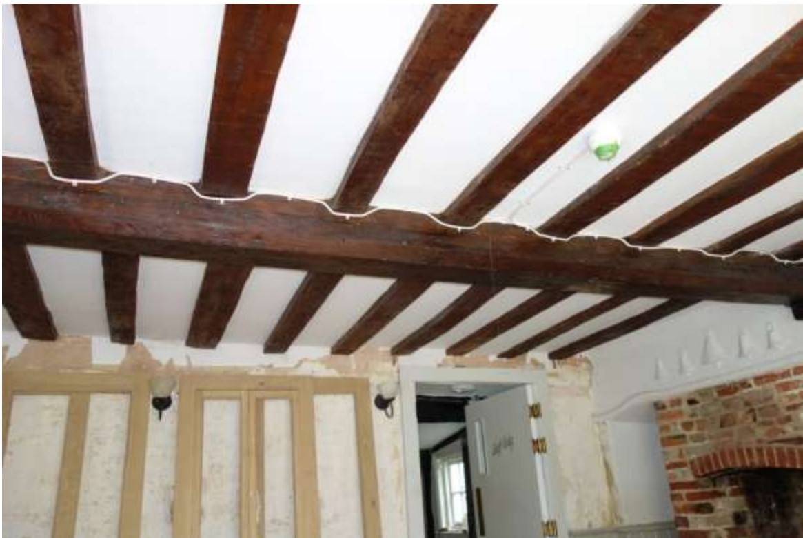
Plate 12. Joist detail in ground floor cross-wing
