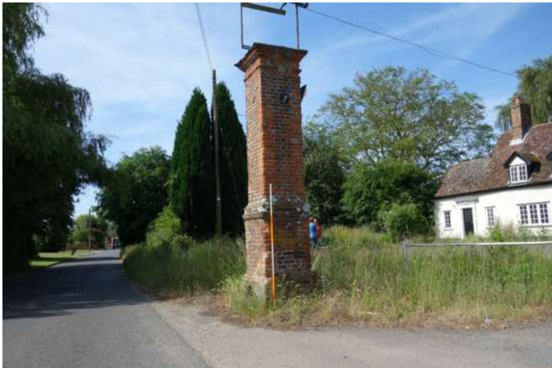
Plate 2. The Inn sign pillar, from the north
