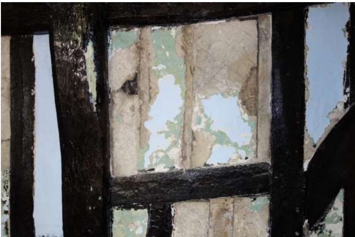
Plate 25. Studwork detail 15th/16th work, with mullion window of early type in ophase 1, first floor
