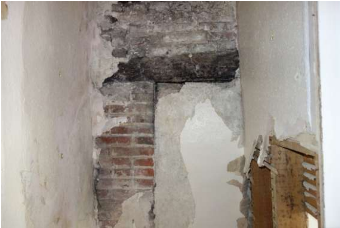
Plate 27. First floor, inserted fireplace into phase 2 stack, looking north
