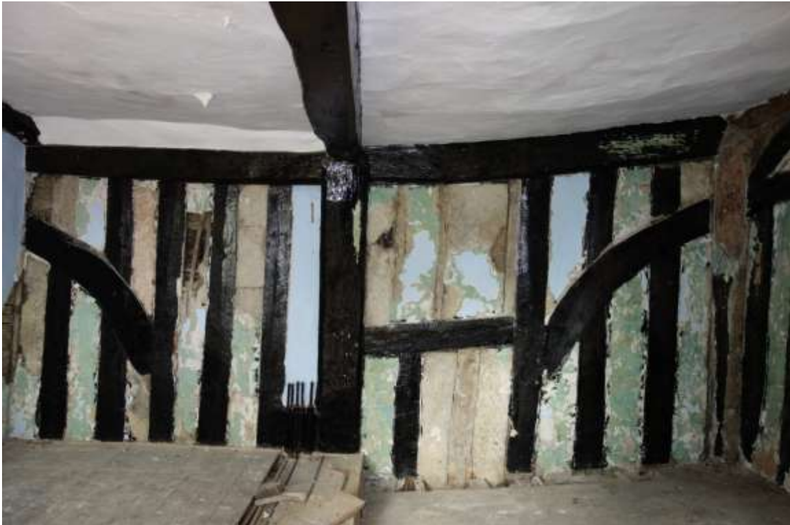
Plate 25. Studwork detail 15th/16th work, with mullion window of early type in ophase 1, first floor
