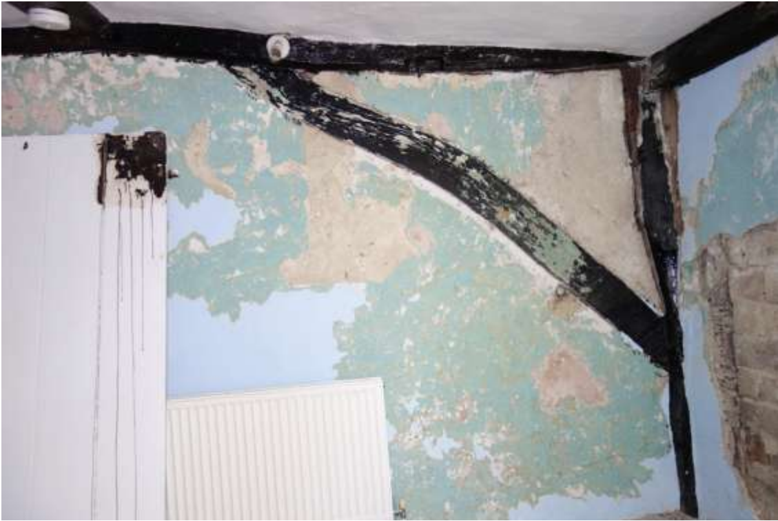
Plate 23. Arch brace, otherside of door (unchanged) in first floor of phase 1
