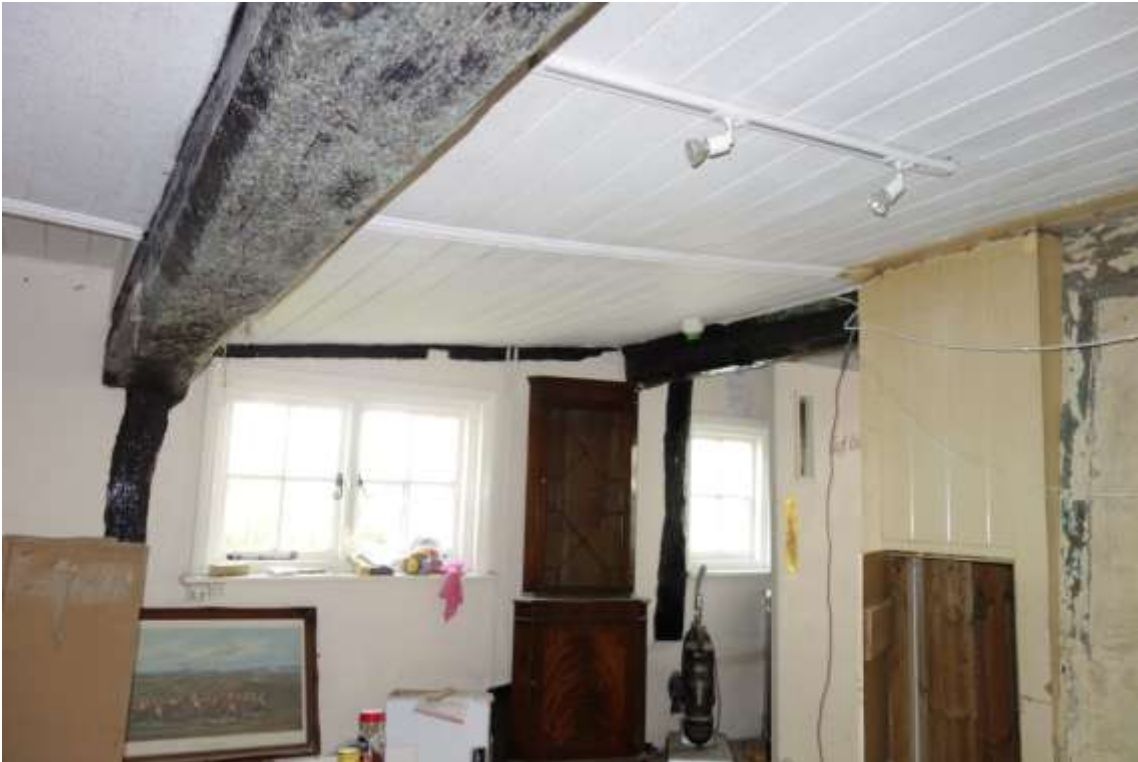
Plate 19. Interior view of phase 1, cell 1 ground floor
