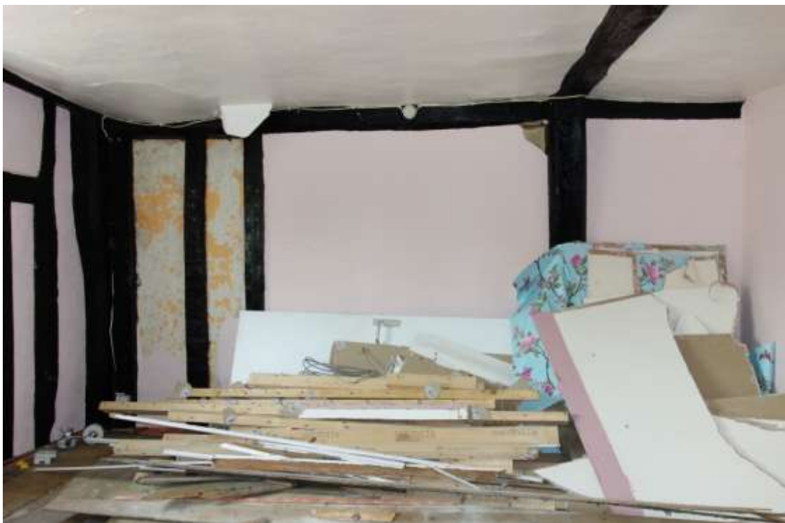
Plate 30. General view of first floor in cross-wing, from the north
