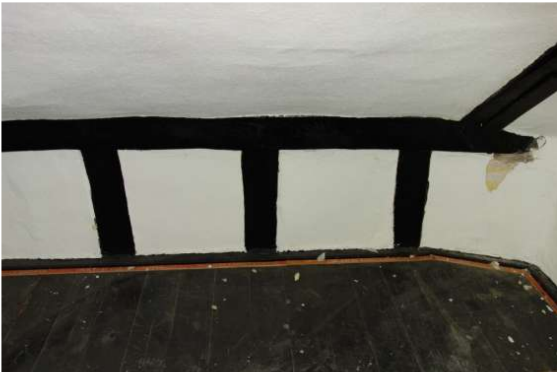
Plate 33. Partition wall of sub-divided room, first floor with tie-beam to roof truss over hall/lounge
