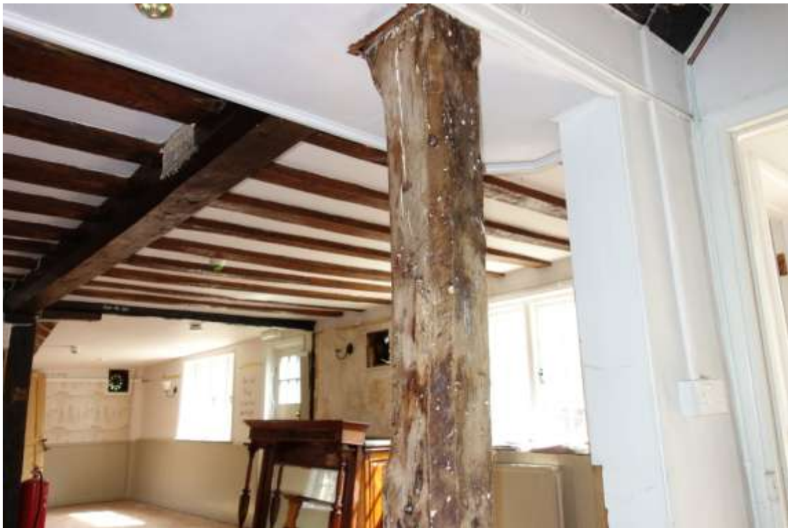
Plate 14. Chamfered post , single survivor of end wall of hall/lounge
