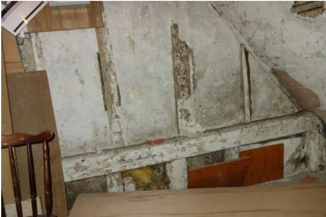
Plate 35. Wall plate and corner post to hall/lounge on first floor, looking west
