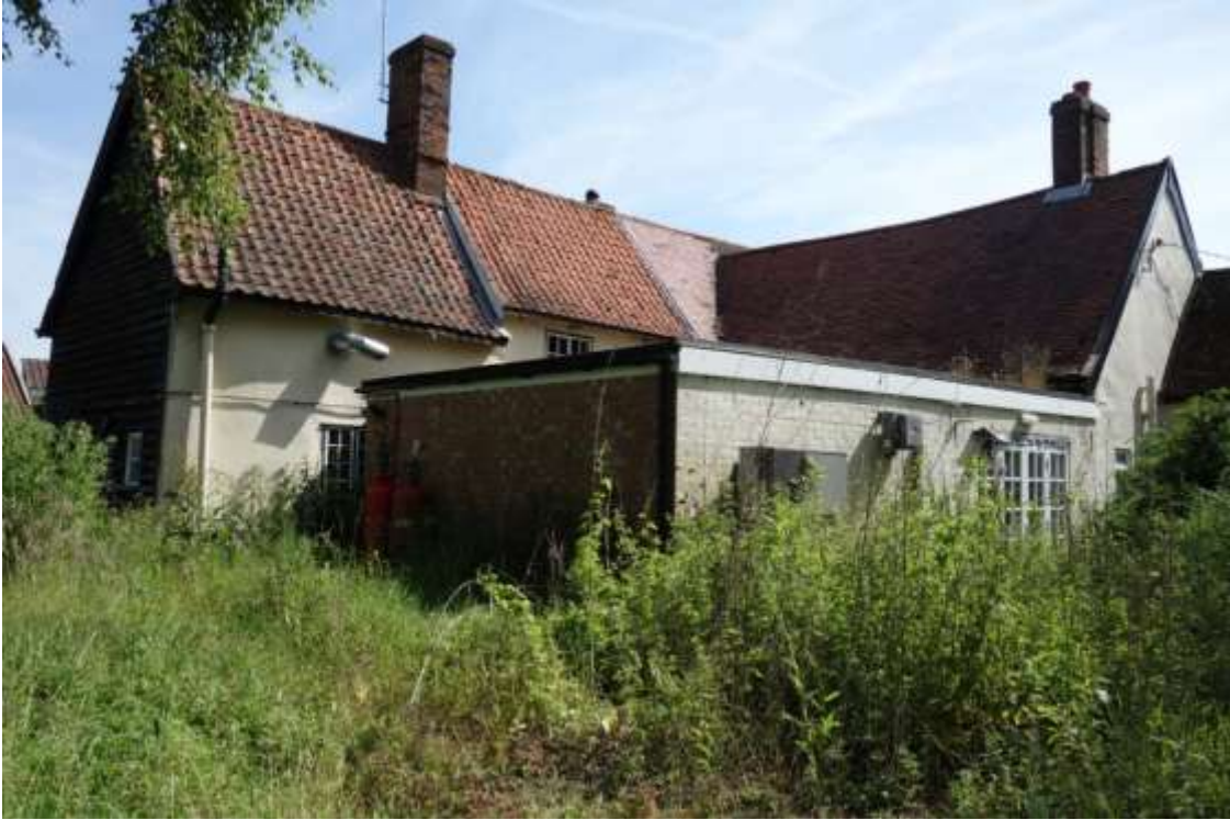
Plate 7. Rear and side view of Inn, from the south-west
