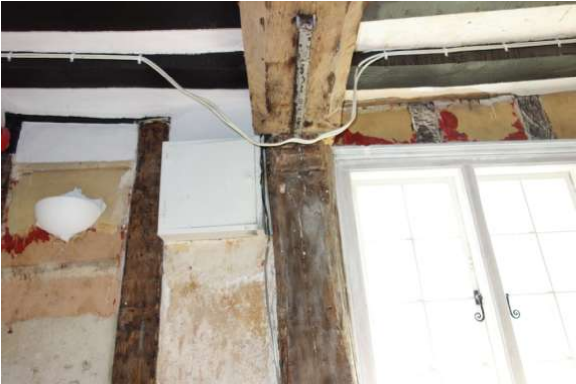
Plate 11. Ogee moulding at top of principal storey post
