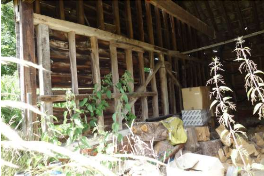
Plate 41. Cart shed bay interior studwork
