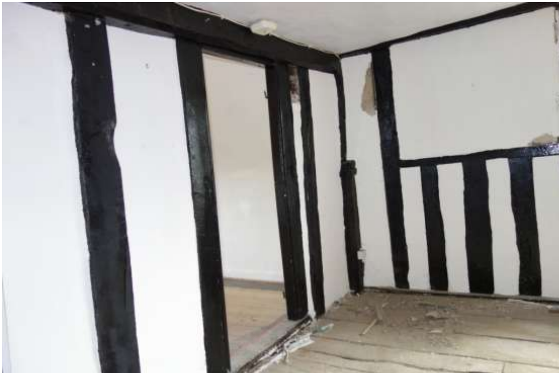
Plate 28. Studwork detail in first floor crosswing to northern range
