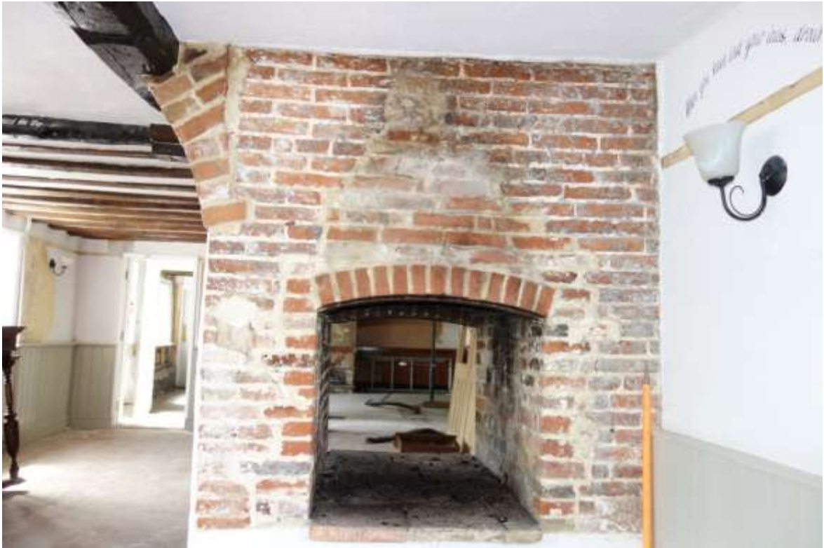
Plate 17. Fireplace/oven in phase 2, cell 2 (lounge), showing late Tudor brickwork, altered in the 18th century (note the dome-shape of the oven in the brickwork now filled in above the arch)
