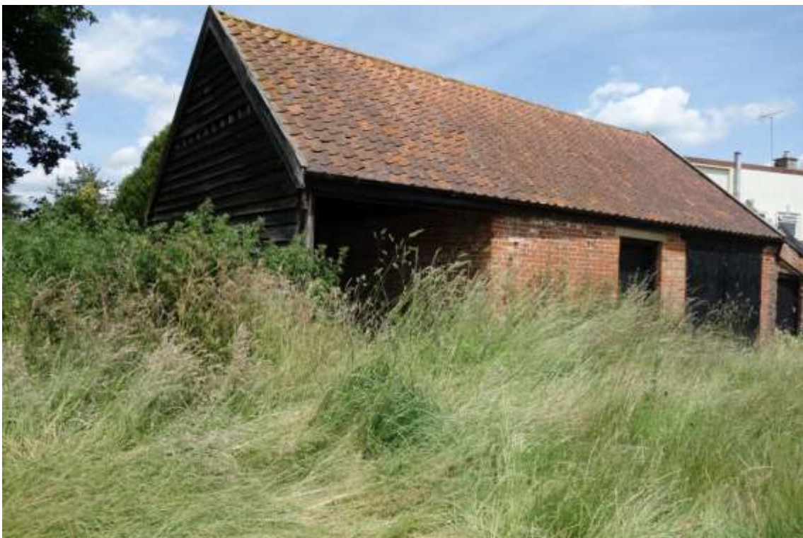
Plate 40. Nineteenth century cart shed from the south-west
