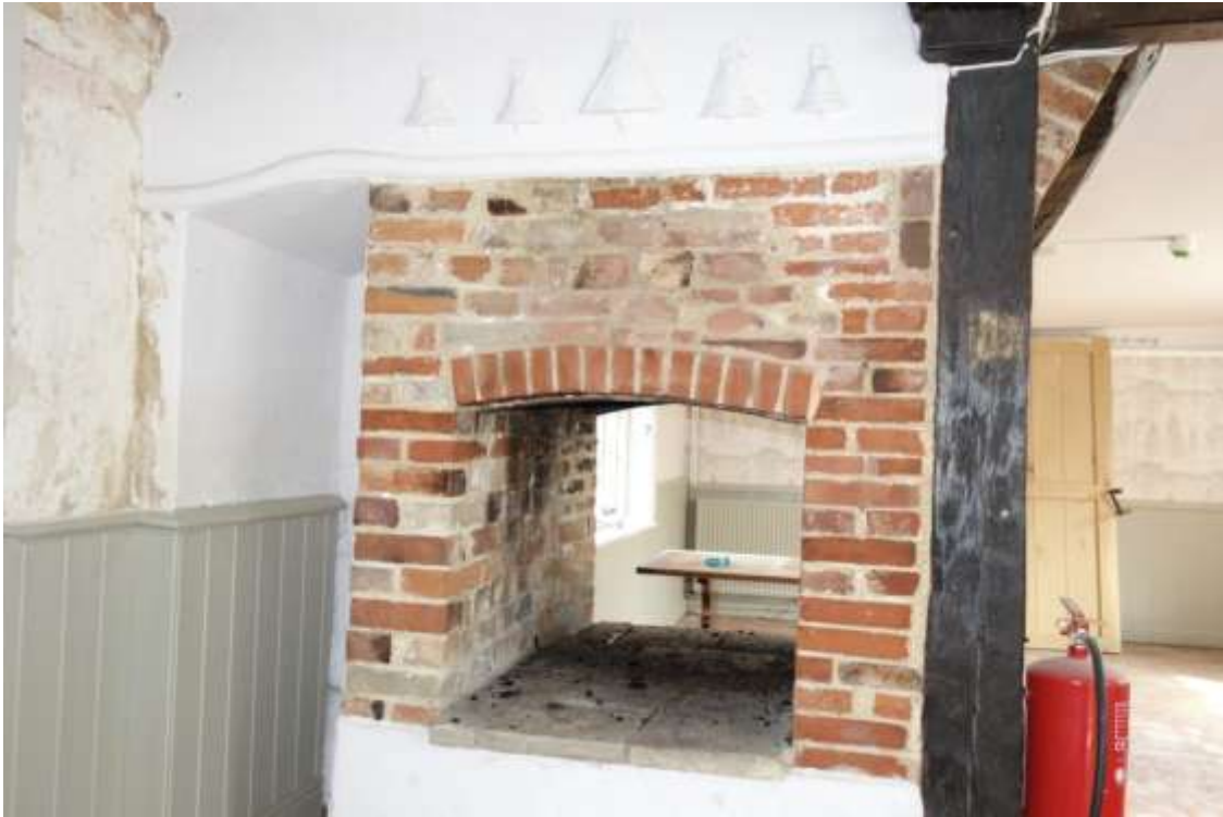
Plate 13. Late 16th fireplace/oven, altered in the 18th century in the northern range
