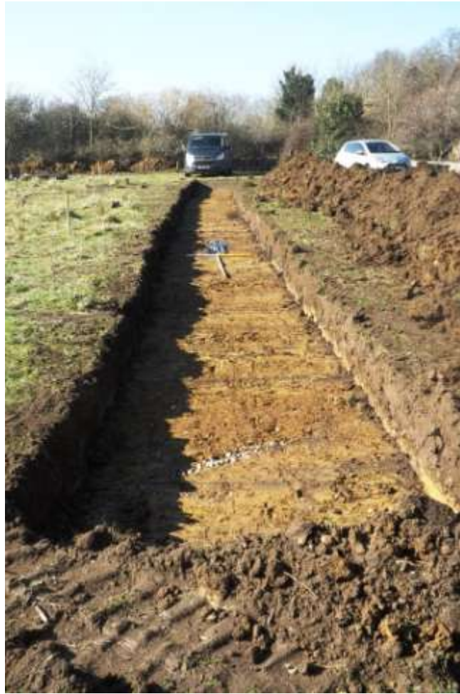
Plate 9. Trench 5, from the east
