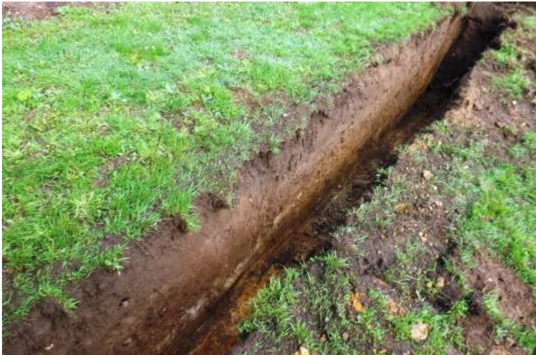
Plate 2. Footings trench, general view
