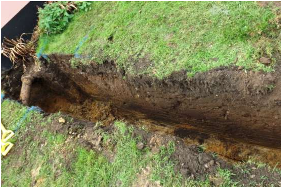
Plate 4. Footings trench, general veiw
