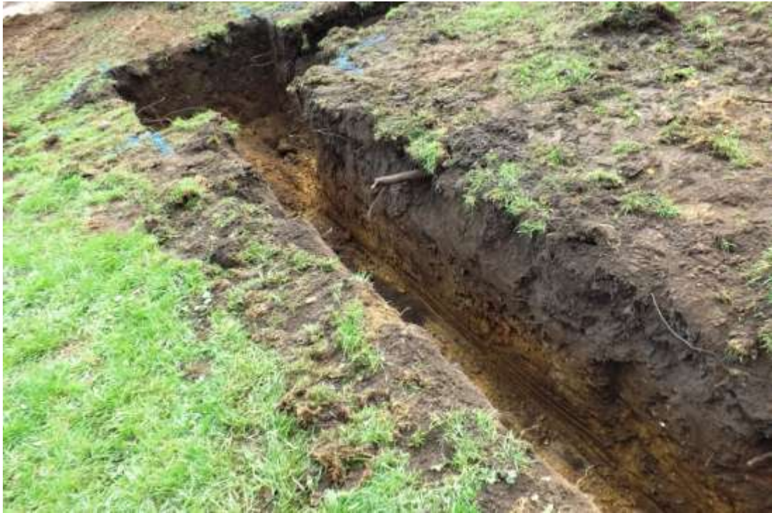
Plate 5. Footings trench, general veiw
