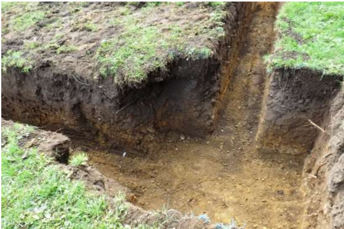
Plate 6. Footings trench, general veiw
