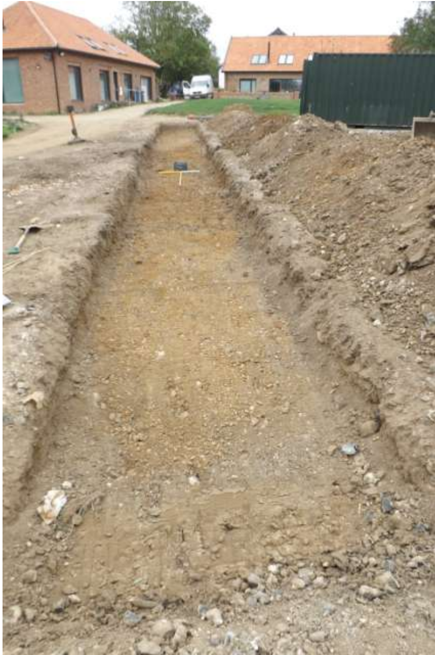
Plate 13. Trench 1. post-excavation, looking north-west
