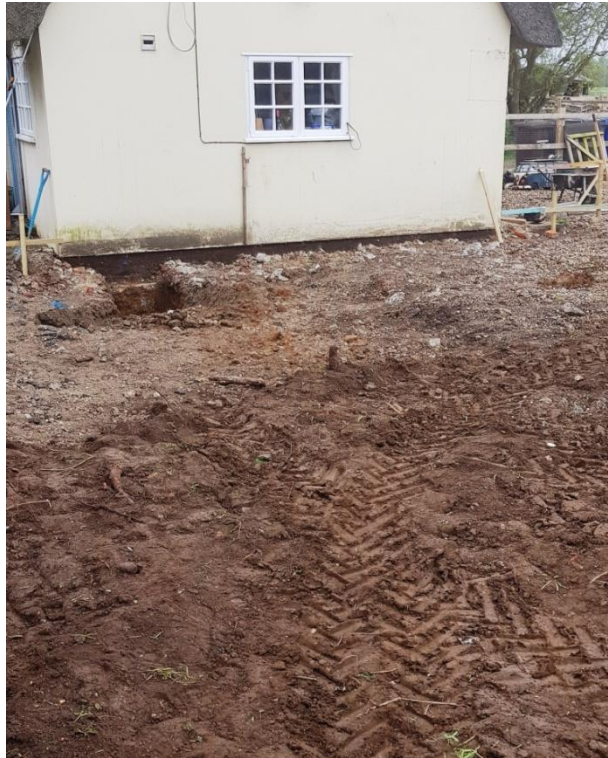
Plate 1. Pre-excavation, from the north-east
