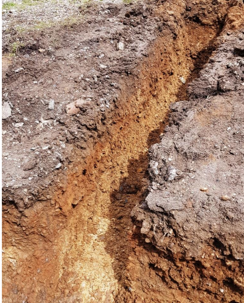
Plate 5. General view of footings trench
