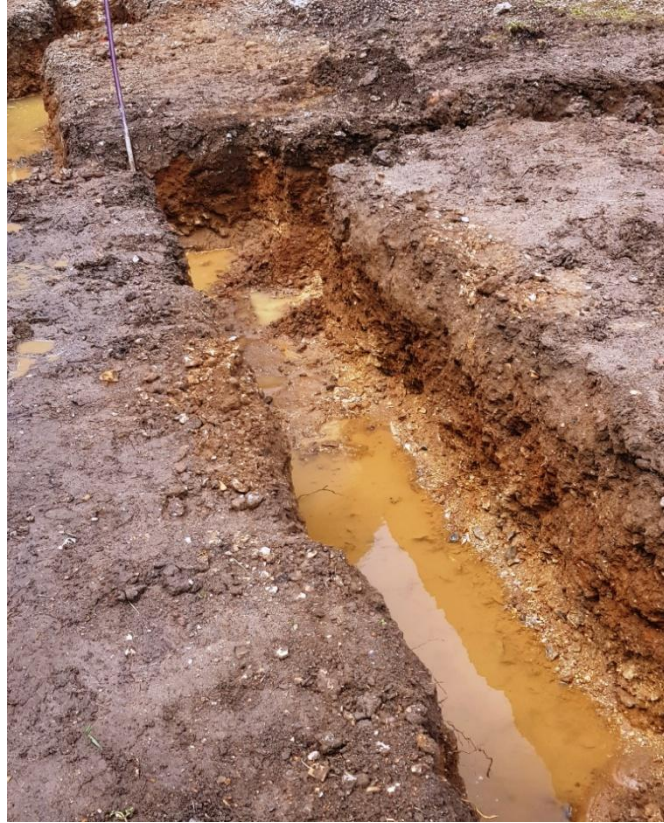
Plate 3. General view of footings trench showing made-up deposit
