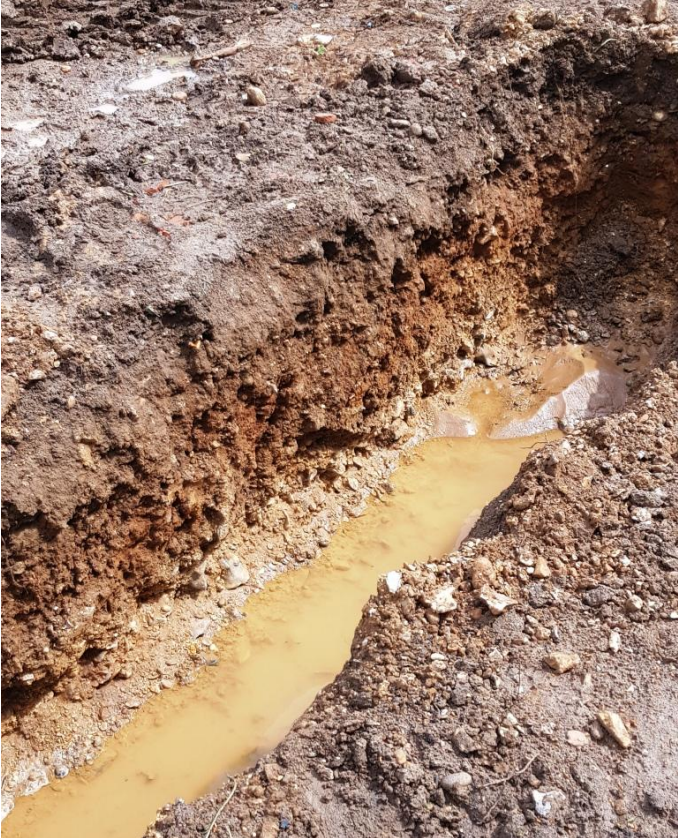
Plate 4. General view of footings trench
