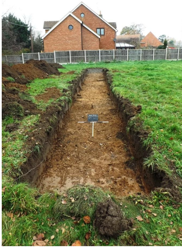
Plate 6. Trench 1, post-excitation, looking north-west
