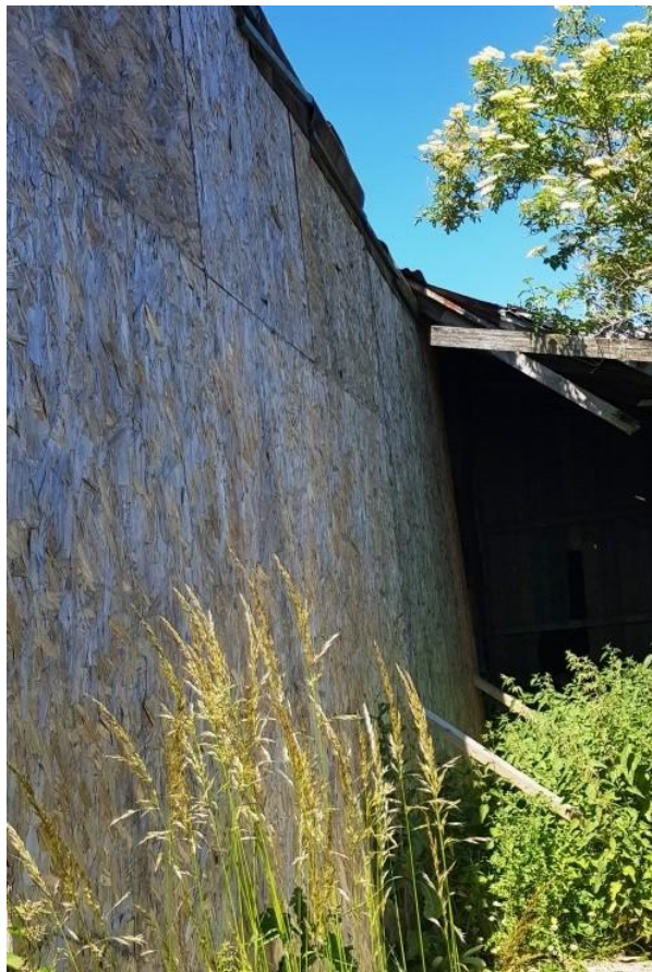
Plate 39. Rear elevation of cow house (now boarded up)
