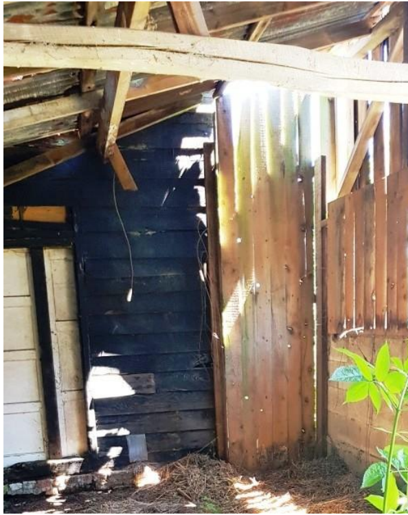
Plate 38. Interior of breeze-block-built extension to cow house
