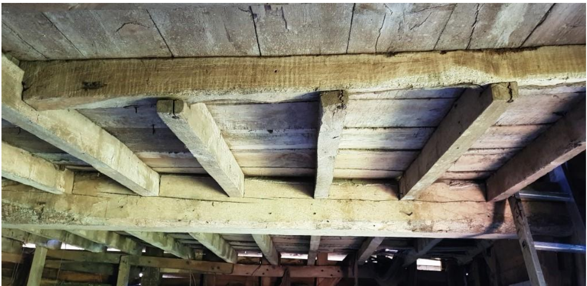
Plate 32. Blocked-off original access hatch to hayloft in northern cell
