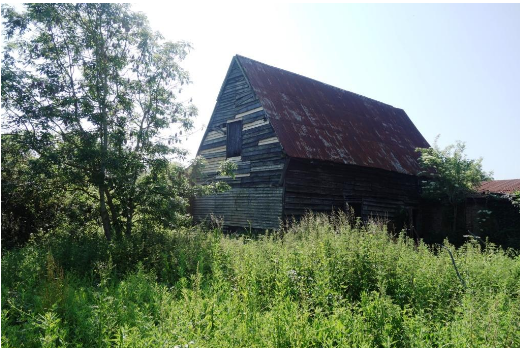
Plate 2. Barn, gable end, north-facing
