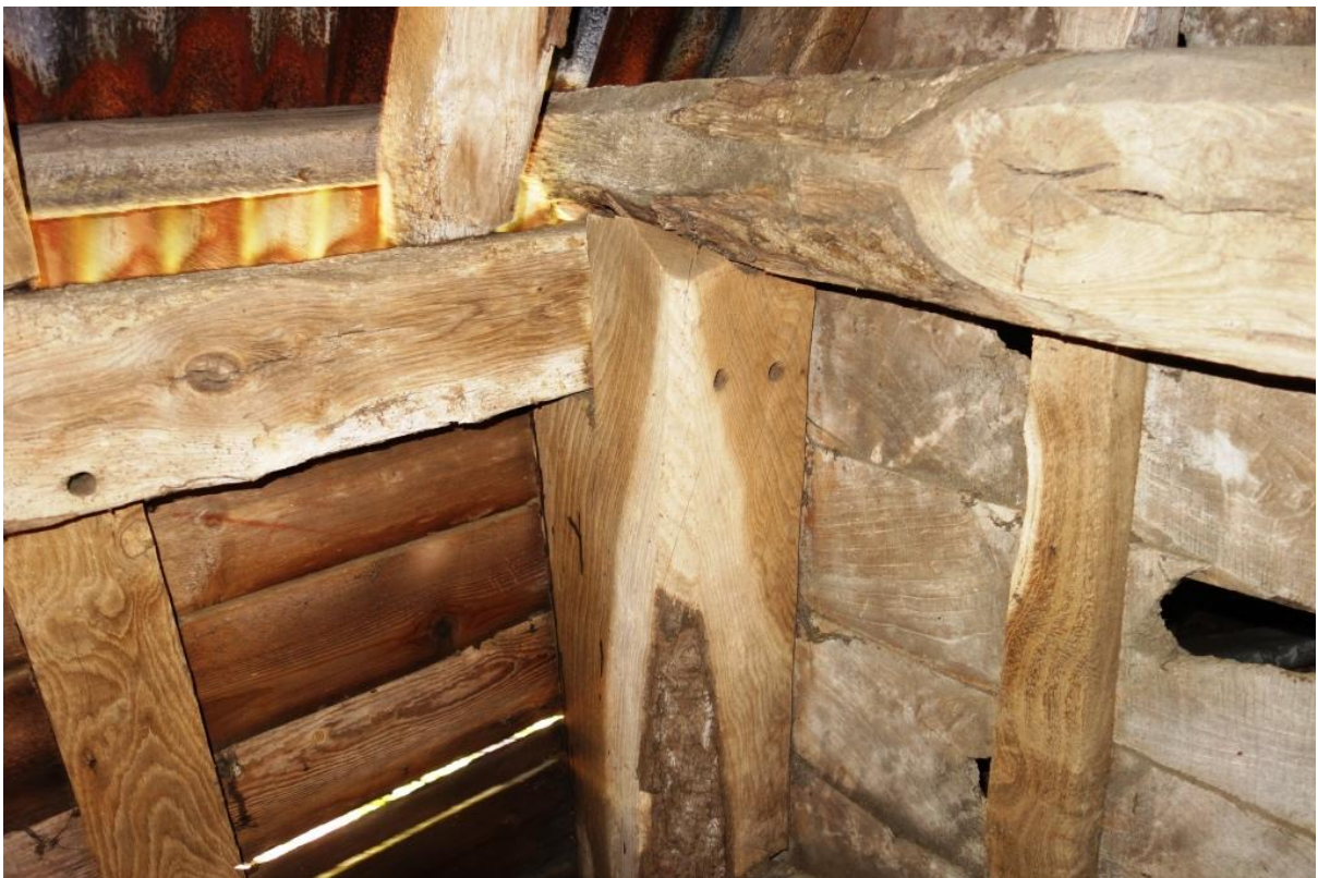
Plate 30. Jowled corner post detail (south-east corner of cow house)
