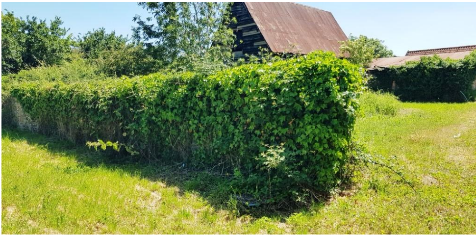
Plate 36. Flint retaining wall to farmyard (c. 19th century)
