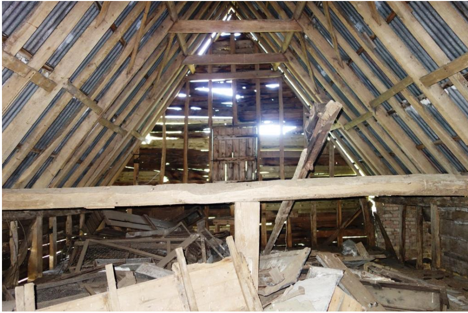
Plate 25. View into hayloft, from the south
