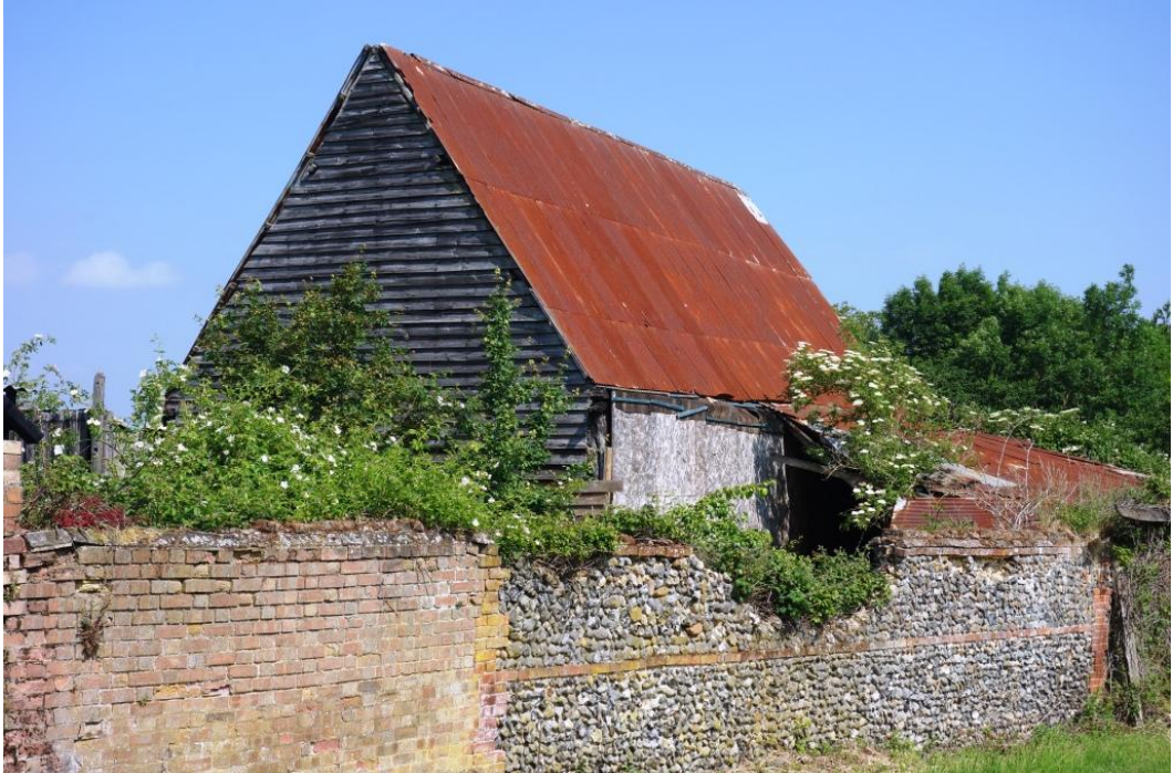
Plate 4. Cow house from the road, and the south-east
