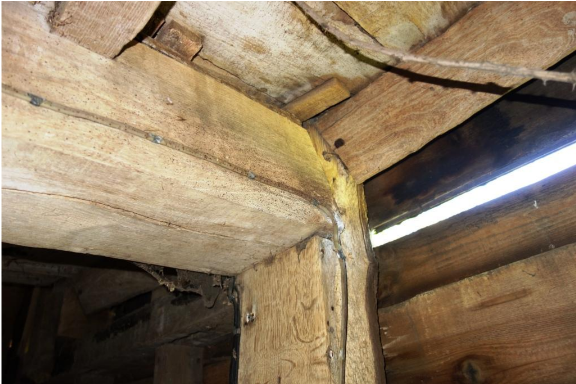
Plate 22. Chamfered beam and stop detail in southern cell
