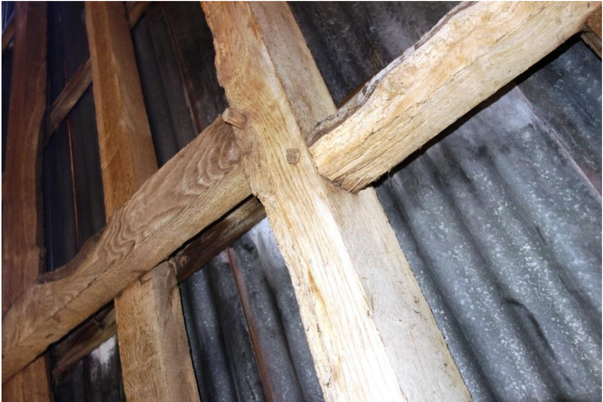
Plate 29. Peg joint detail in roof truss
