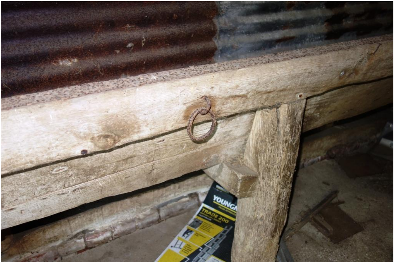
Plate 12. Detail of original feeding trough with tethering ring
