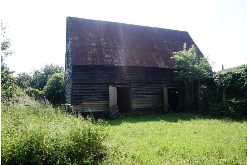
Plate 1. Barn and adjoining range, from the north
