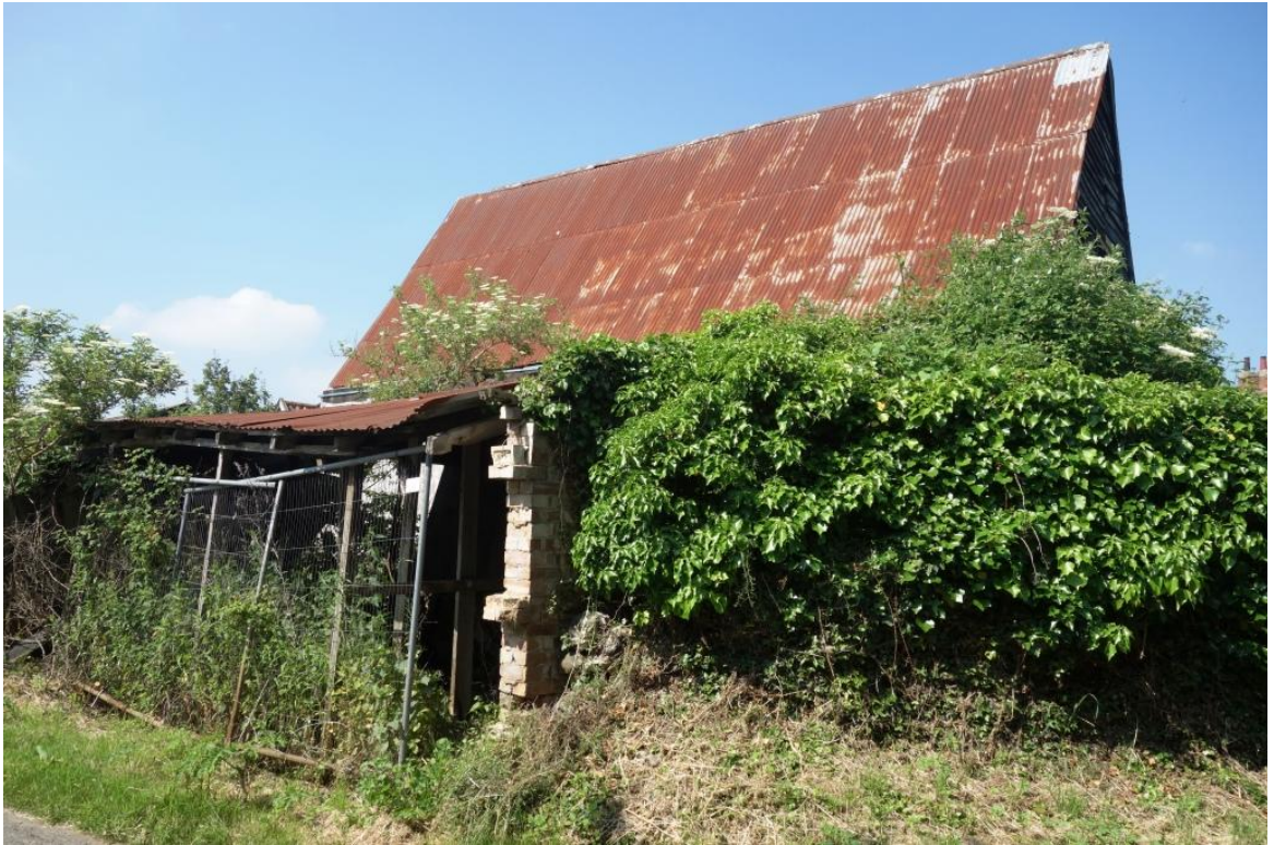
Plate 5. Cow house, from the north-east
