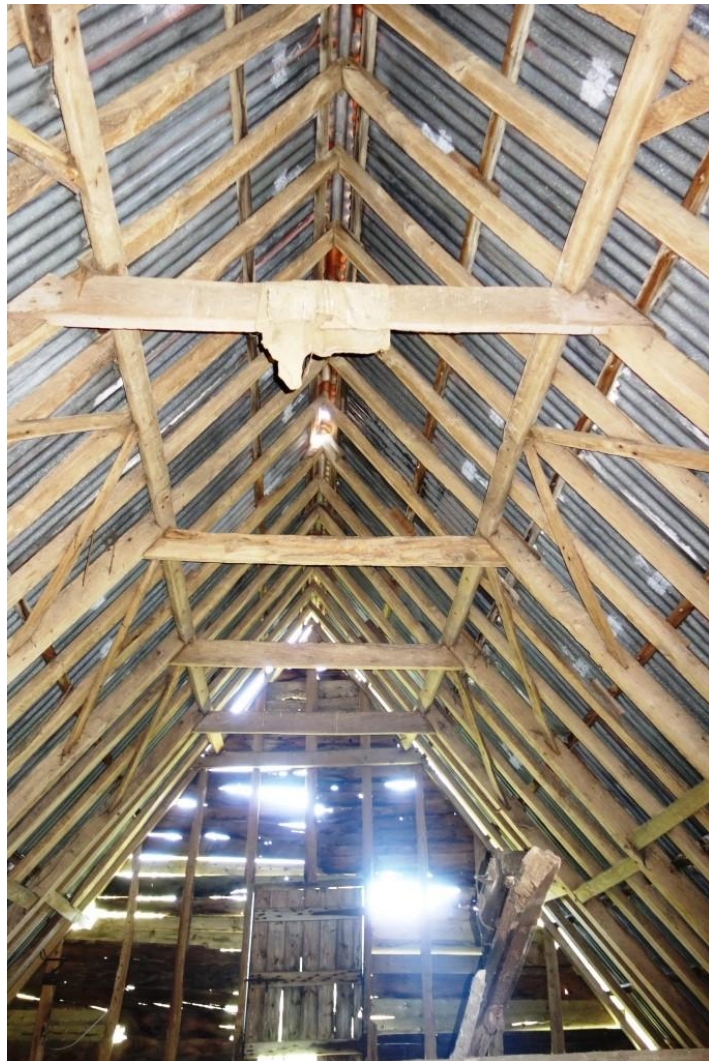
Plate 26. Roof truss detail, from the south
