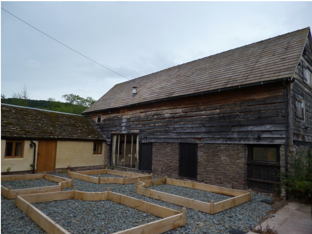
Figure 3a/b: Exterior views of the still standing cross-wing of the now lost hall (top) and the parallel barn range to its west (bottom)
