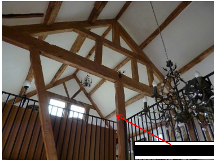
Figure 6e: Annotated photograph of the barn trusses to locate sampled timbers (see Table 1)
