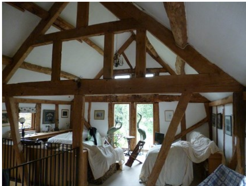
Figure 5a/b: Interior views of the barn range, looking west to east (trusses 2 and 3) (top) and east to west (trusses 4 and 5) (bottom)
