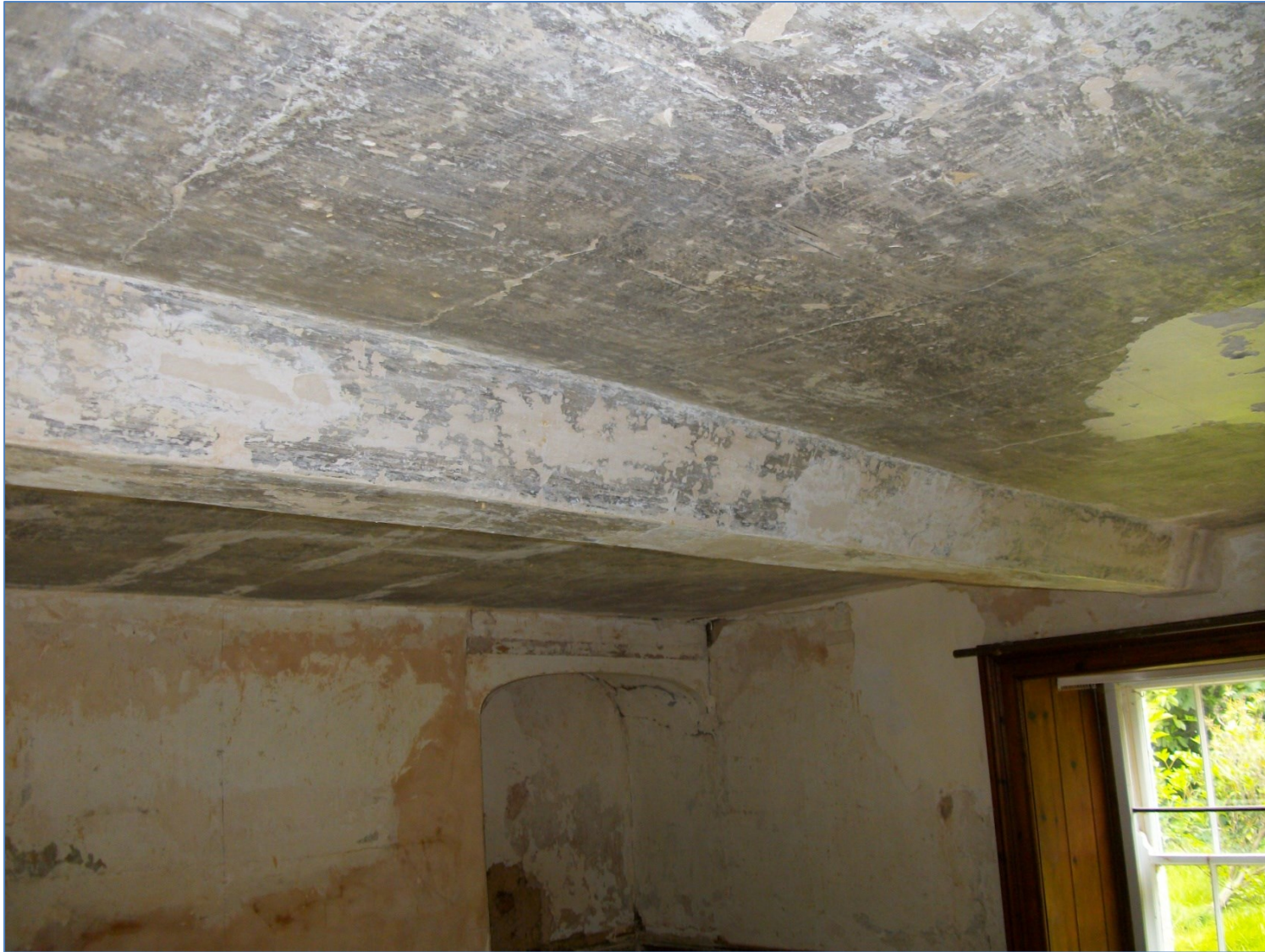
Figure 7: South range; ground-floor ceiling beam (southern one)
