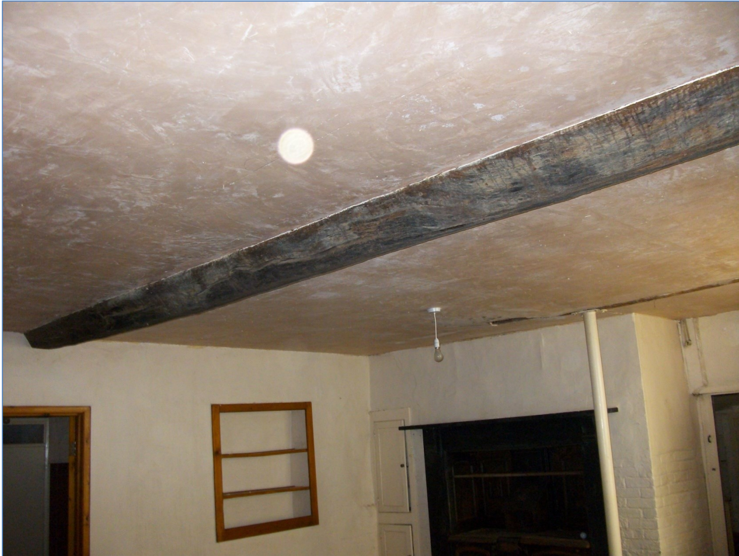
Figure 9: North range; ground-floor ceiling beam
