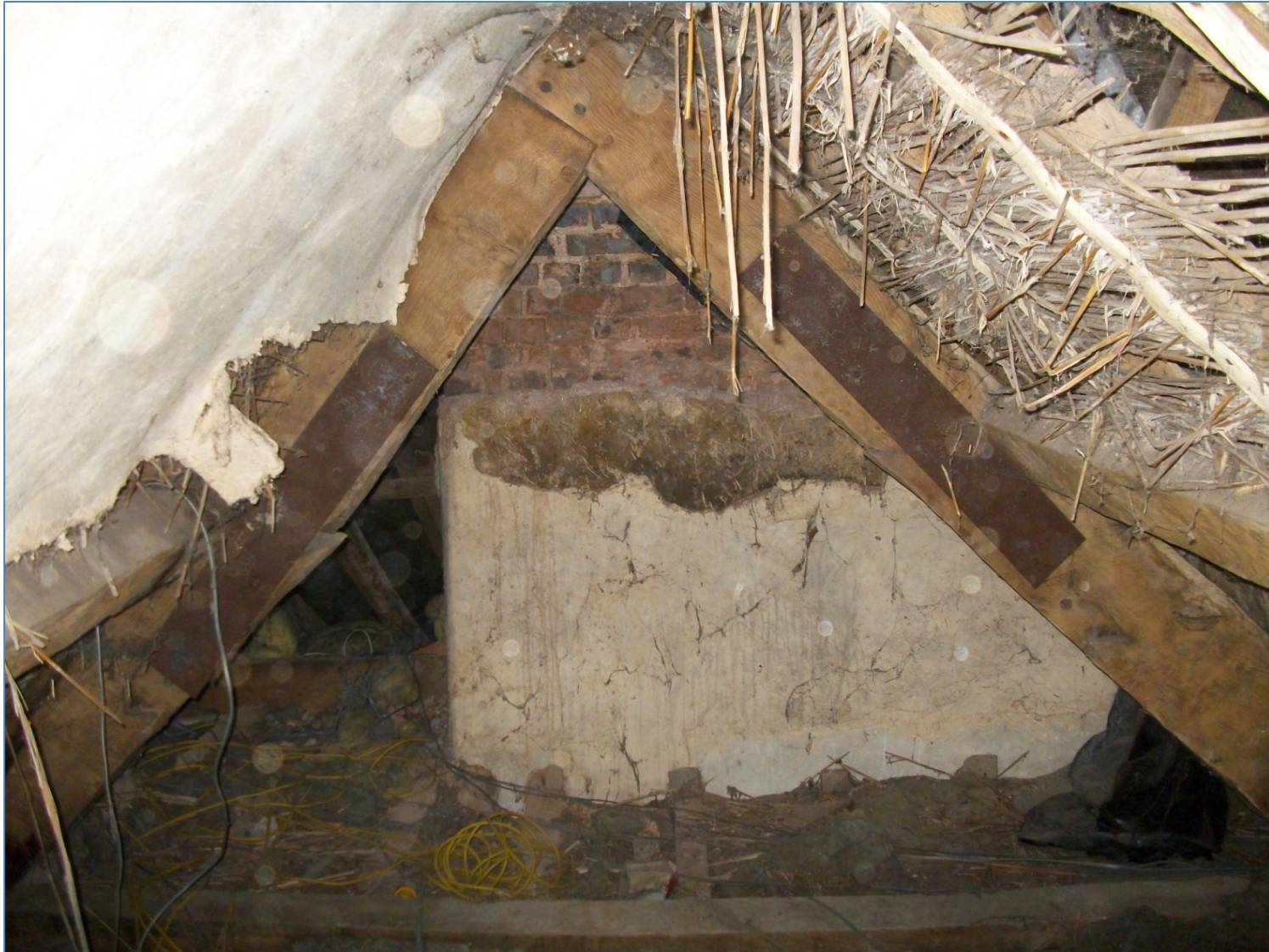
Figure 4: Main range roof, truss 4 (east face)
