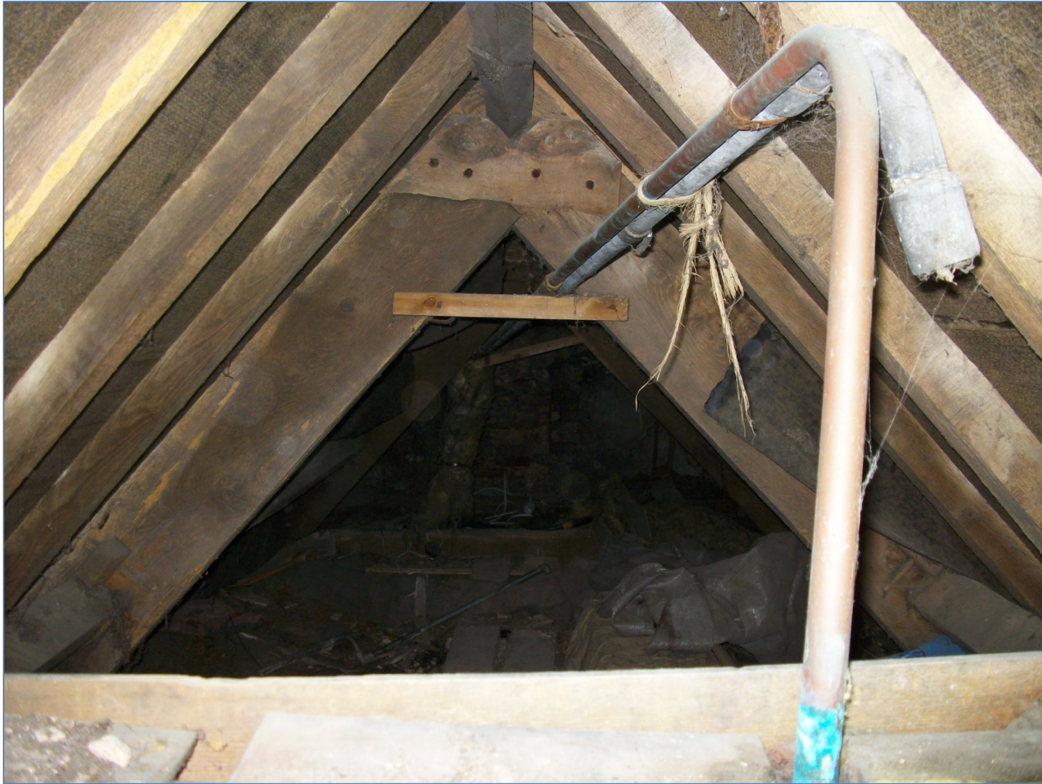
Figure 8: North range roof, truss 8 (south face)
