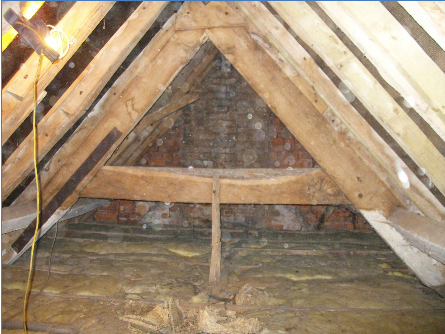
Figure 5: South range roof, truss 6 (north face)
