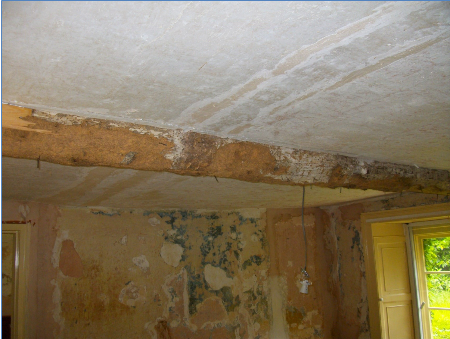
Figure 6: South range; ground-floor ceiling beam (northern one)
