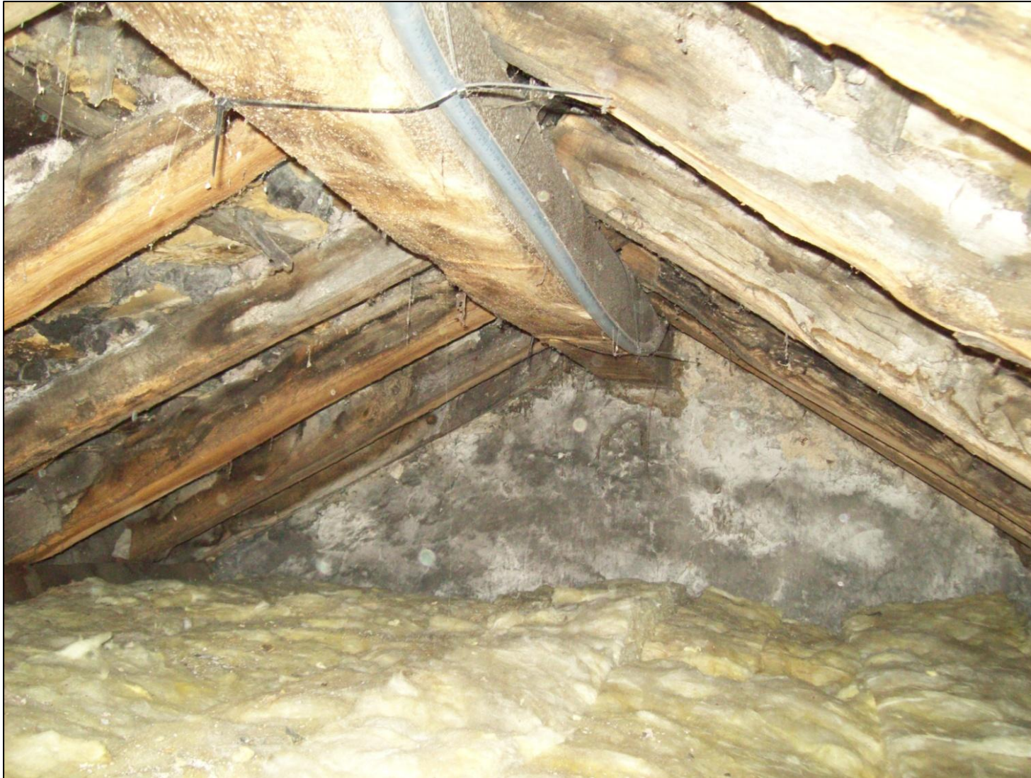
Figure 2: The House; bay 4, photograph taken from the south
