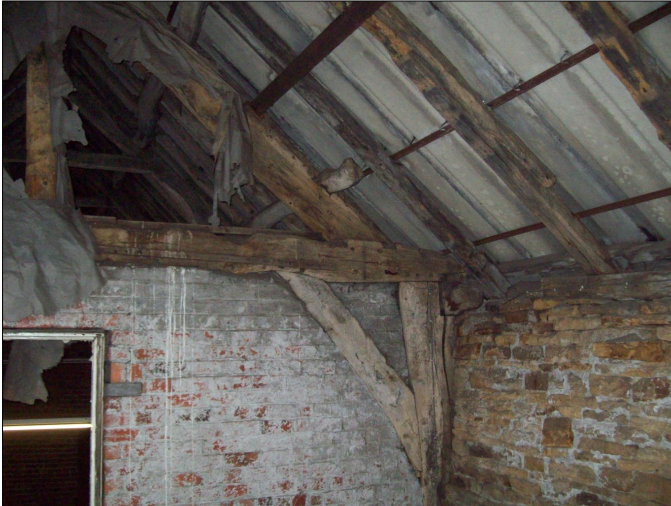
Figure 5: The Barn; truss 6, photograph taken from the north
