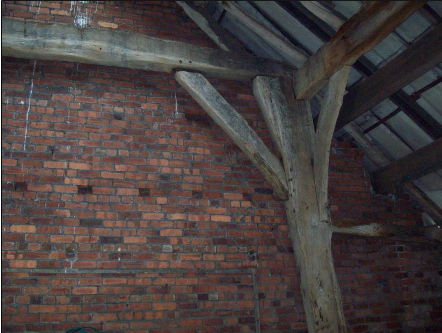
Figure 4: The Barn; east aisle post of truss 3
