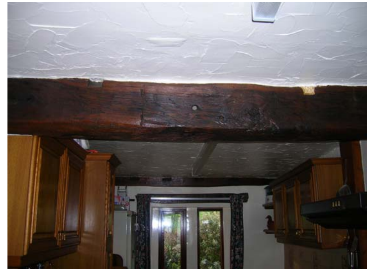
4b above: view of the ceiling beam in the kitchen
