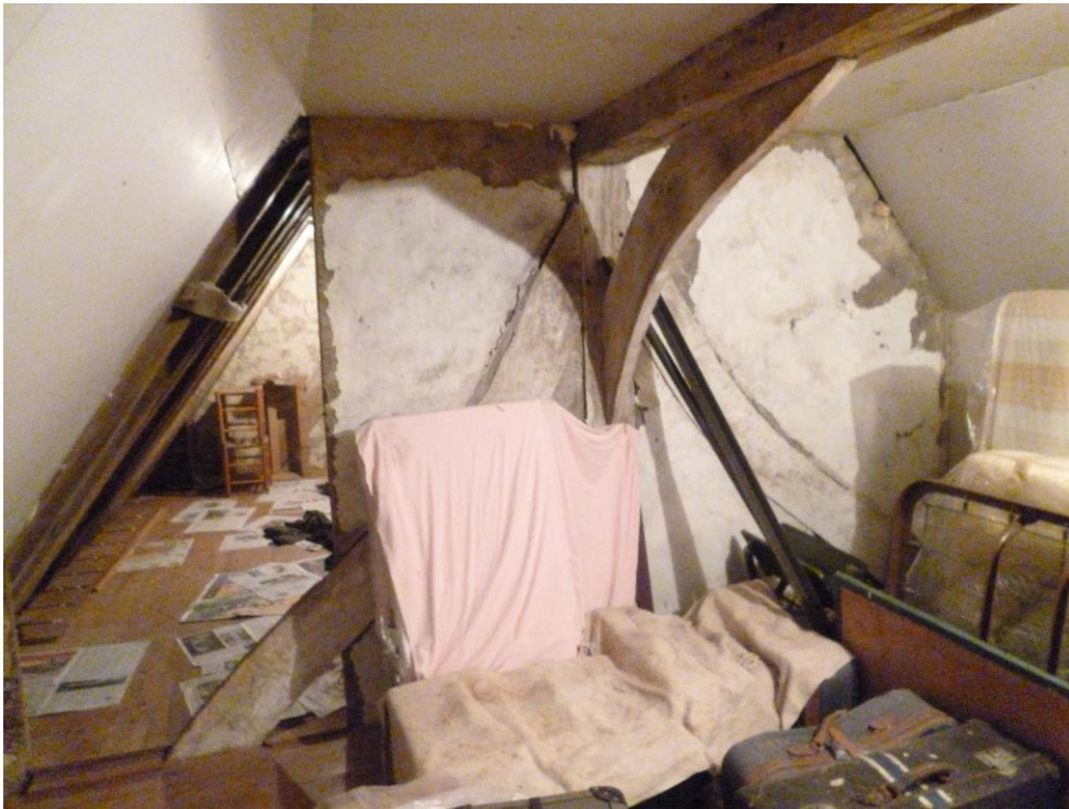
Figure 2a (top): View of the west face of truss 1
