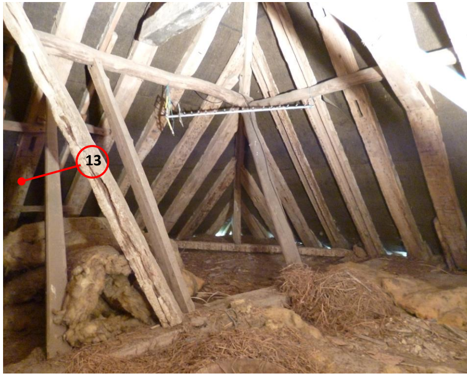
Figure 4d: Photograph of the west hip end to show sampled timber
