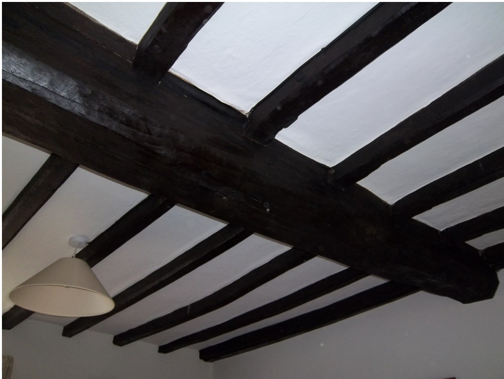
Figure 5: The main bridging beam of the ground floor ceiling to the lounge, cored as sample MKV-A04
