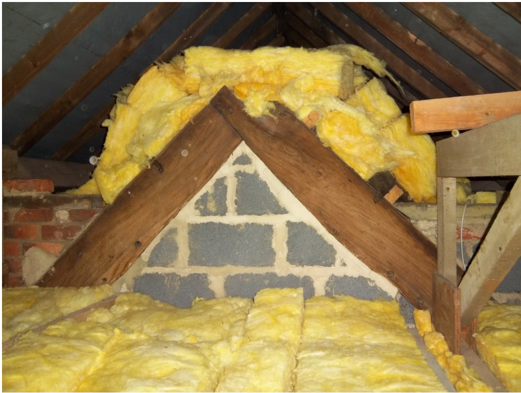
Figure 4: View of the apex of the remaining truss showing that it does not support the roof
