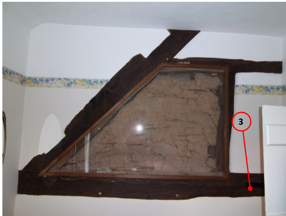
Figure 2a/b: Views of the single remaining truss (top) and the panel of wattle and daub in-fill (bottom). The sampled timbers are also shown
