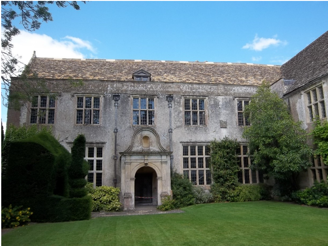
Figure 2a/b: Views of the east range and its southern extension (top), and the south range (bottom)
