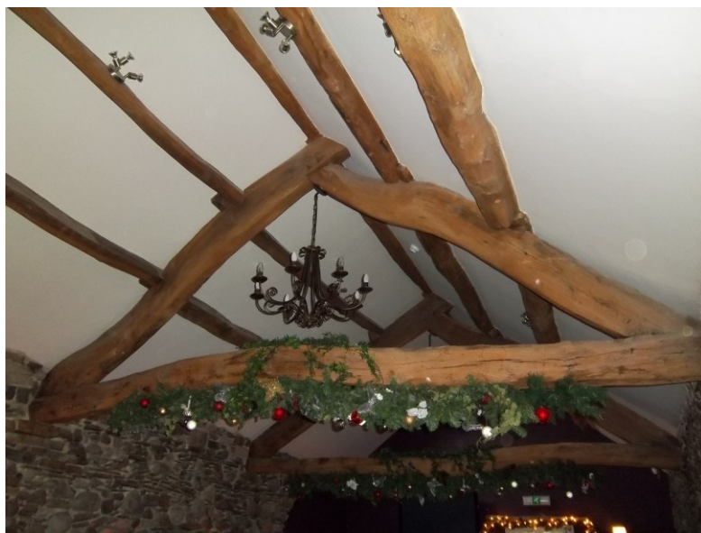
Figure 2a-c: Views of the roof trusses: building 1 (top), 2 (middle) and 3 (bottom)
