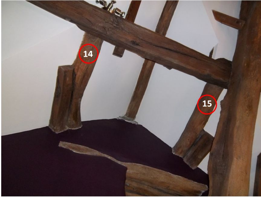
Figure 4d: View of the timbers in the roof between buildings 1 and 2
