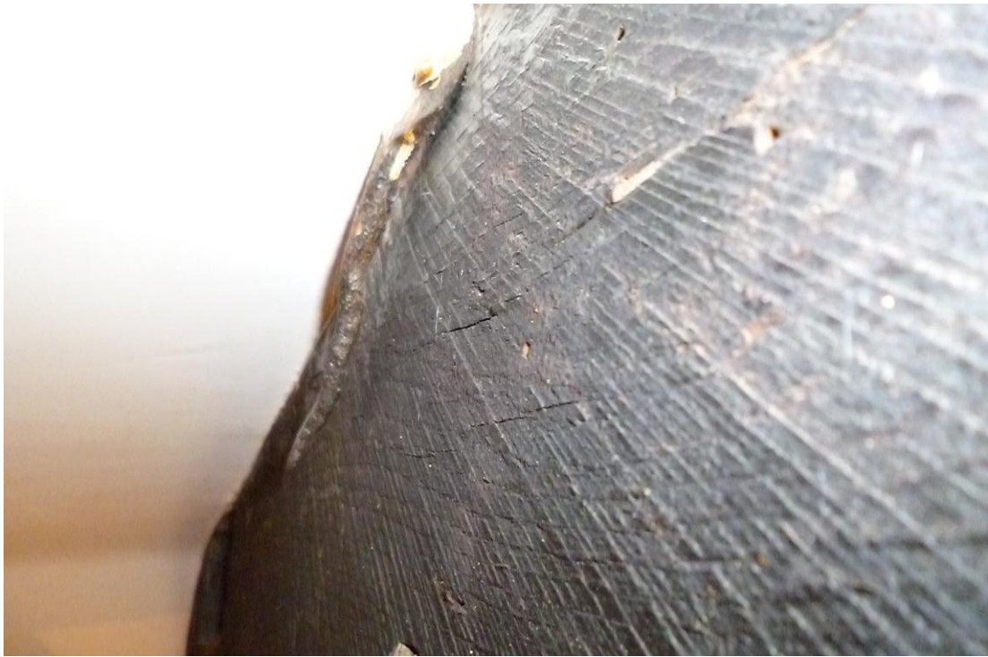
Figure 4c: Saw marks to the face of one timber forming parallel lines
