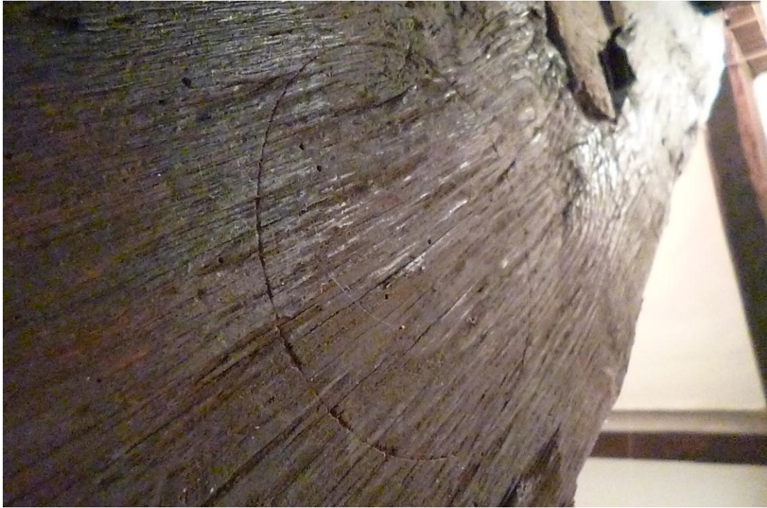
Figure 4e: Circular 'compass' mark to timber, possibly the beginnings of a decorative 'florets' inscription, and as it might have looked, completed, below
