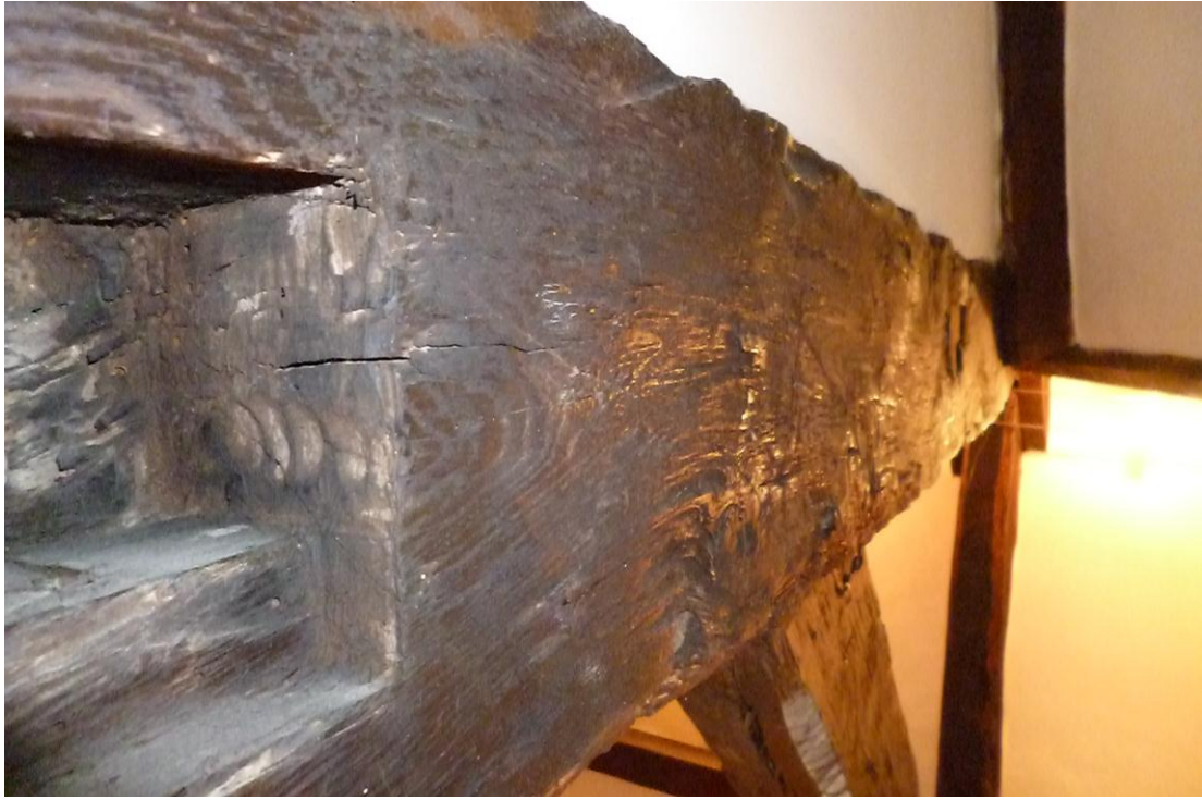
Figure 4d: Adze marks to the face of timber forming characteristic 'scallop'
