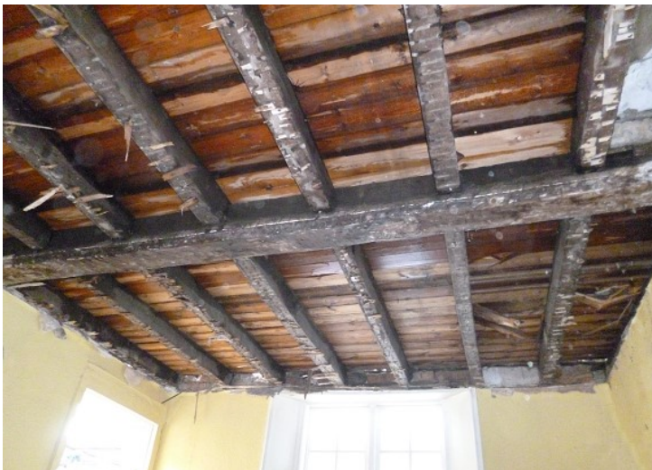
Figure 3a-c: Views of the fragmentary remains of the timbers and the ground floor ceiling frame
