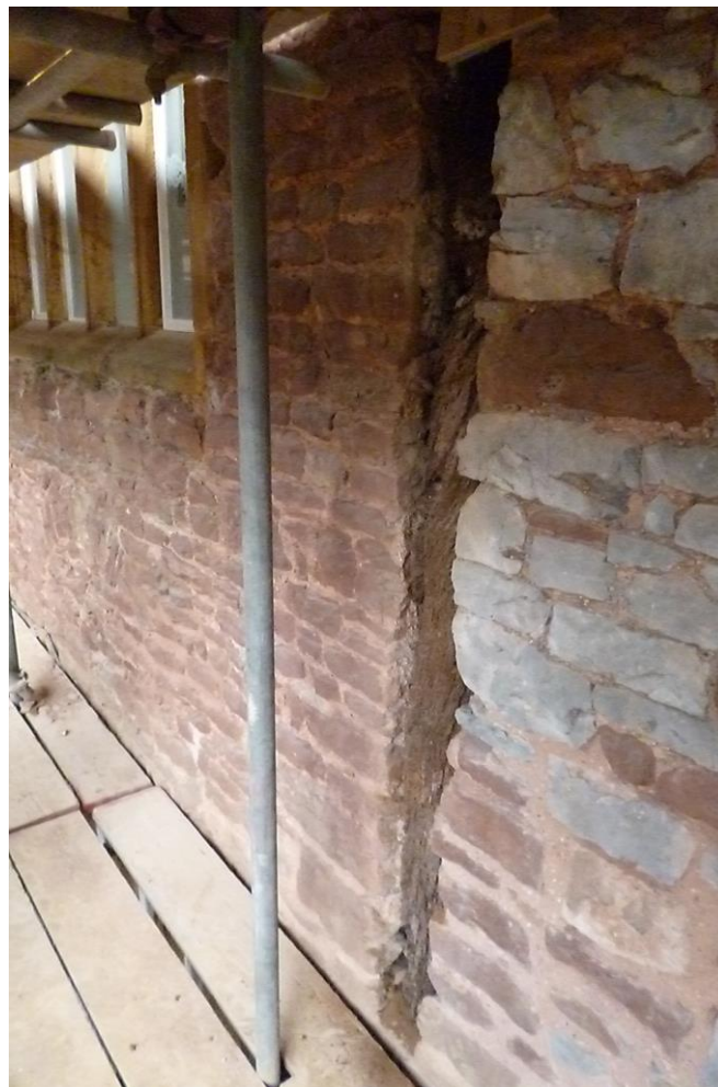
Figure 3d/e: Views of a truss of the sampled south range roof (top) and a post buried in the south wall of the north range (bottom)
