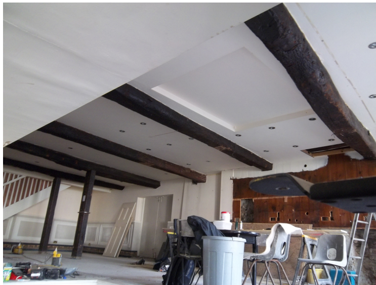
Figure 4d/e: View of the ground-floor pine ceiling beams to 2 Bridge Street (top), sampled as BID-P25–P27 and the ground-floor ceiling beams to 5 Bridge Street (bottom), sampled as BID-A20–A24
