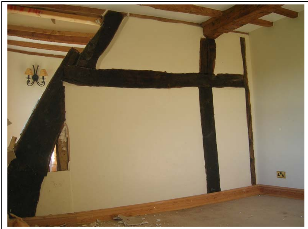
Figure 3a/b: View of the single remaining cruck truss; top, from the east, below, from the north-west
