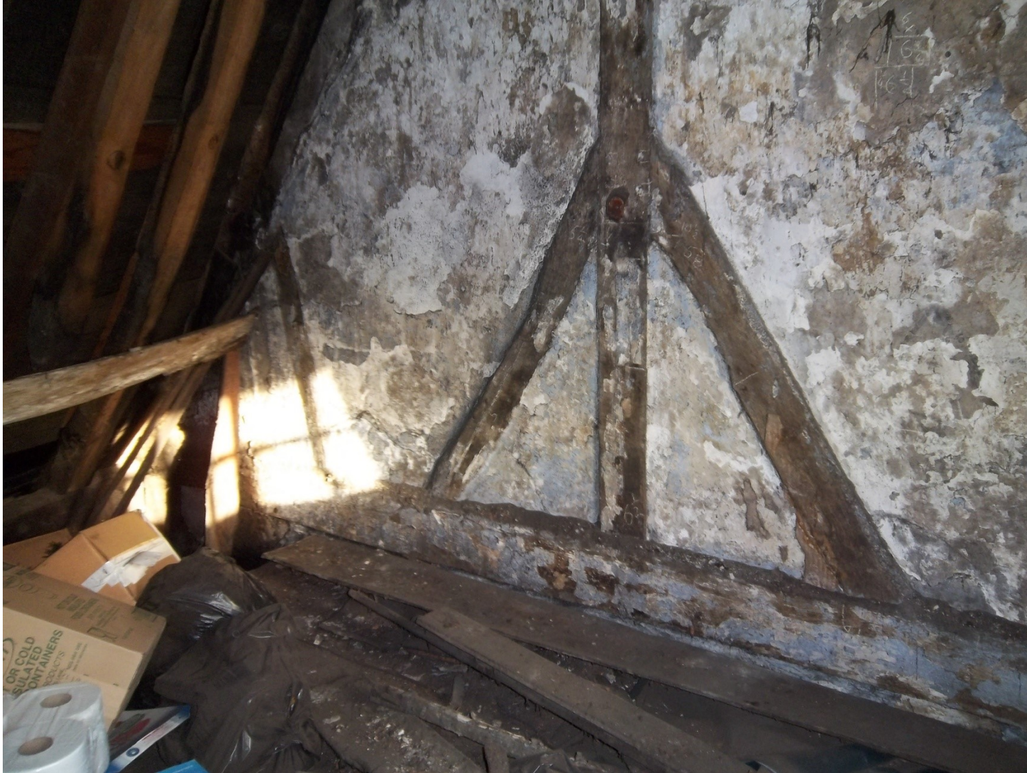
Figure 5: Truss 3 (north face)
