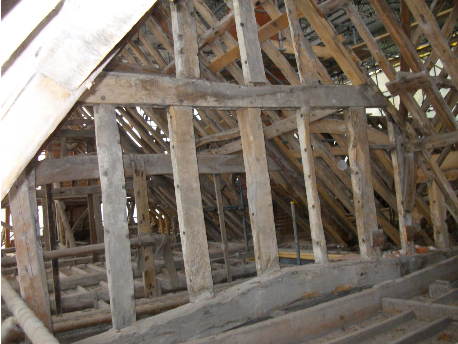
Figure 6: Main range roof; truss 1 (photograph taken from the north)
