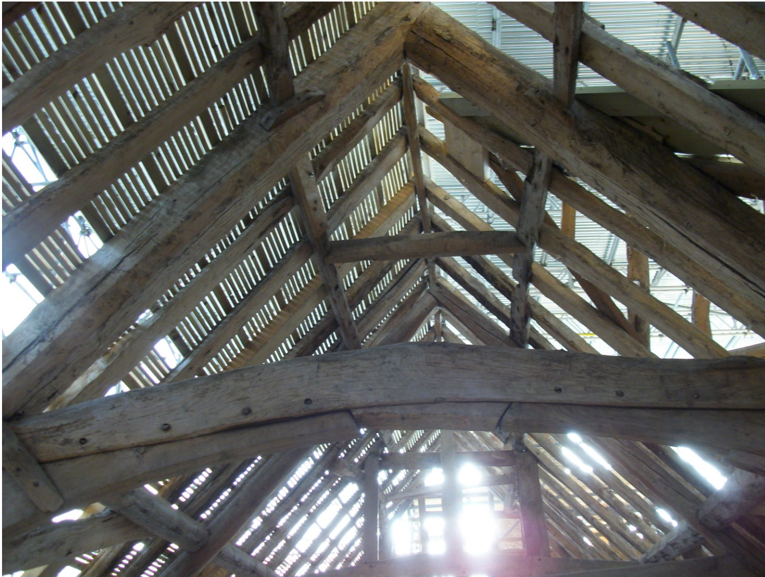
Figure 7: Main range roof; truss 3 (photograph taken from the south)
