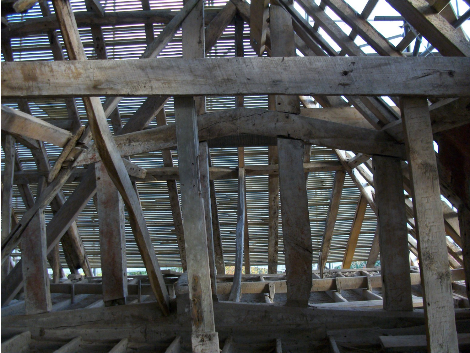
Figure 10: Cross-wing; truss 6 in the background (photograph taken from the west)
