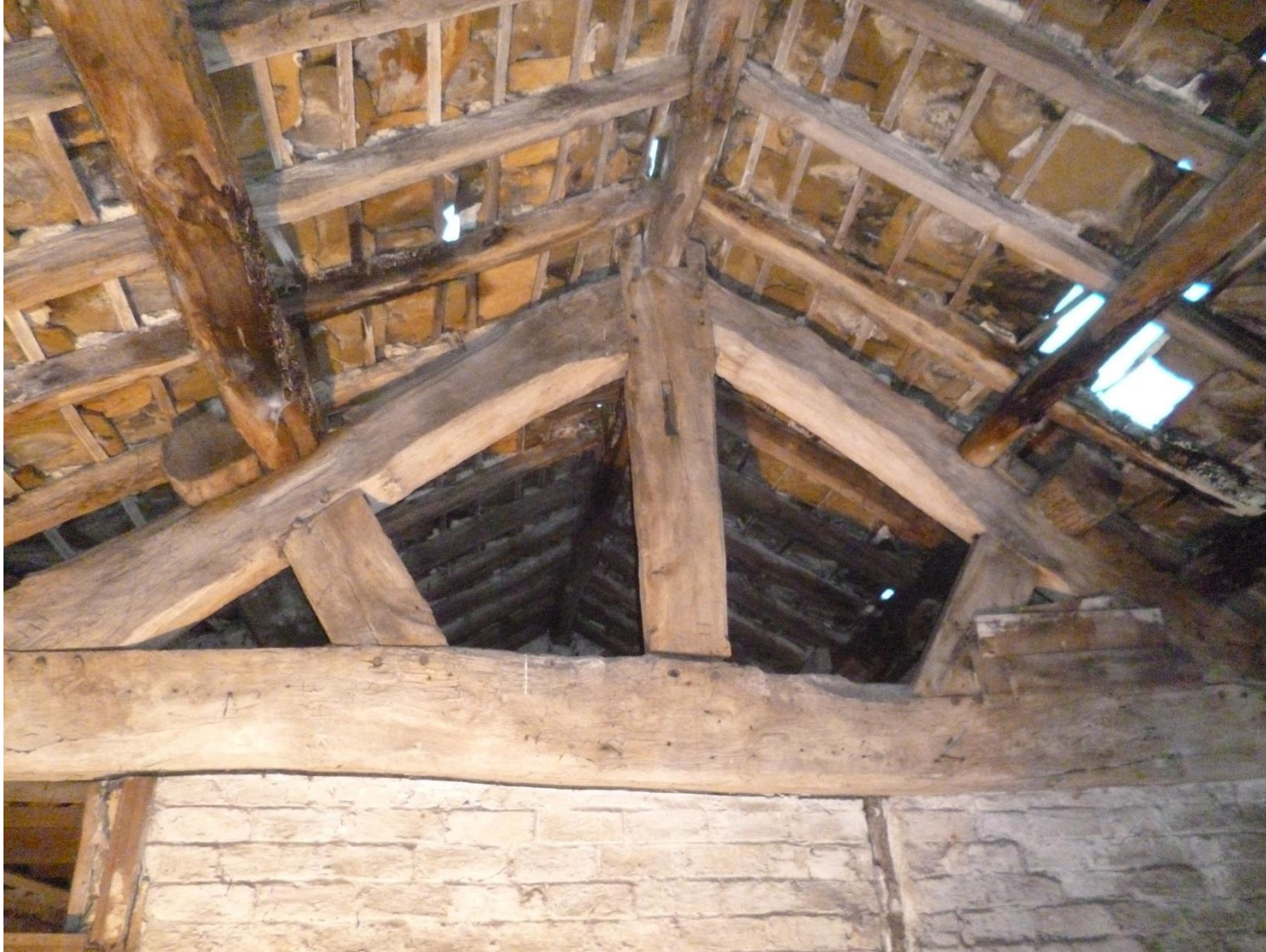
Figure 6: Former farmhouse, truss 2 (photograph taken from the west)
