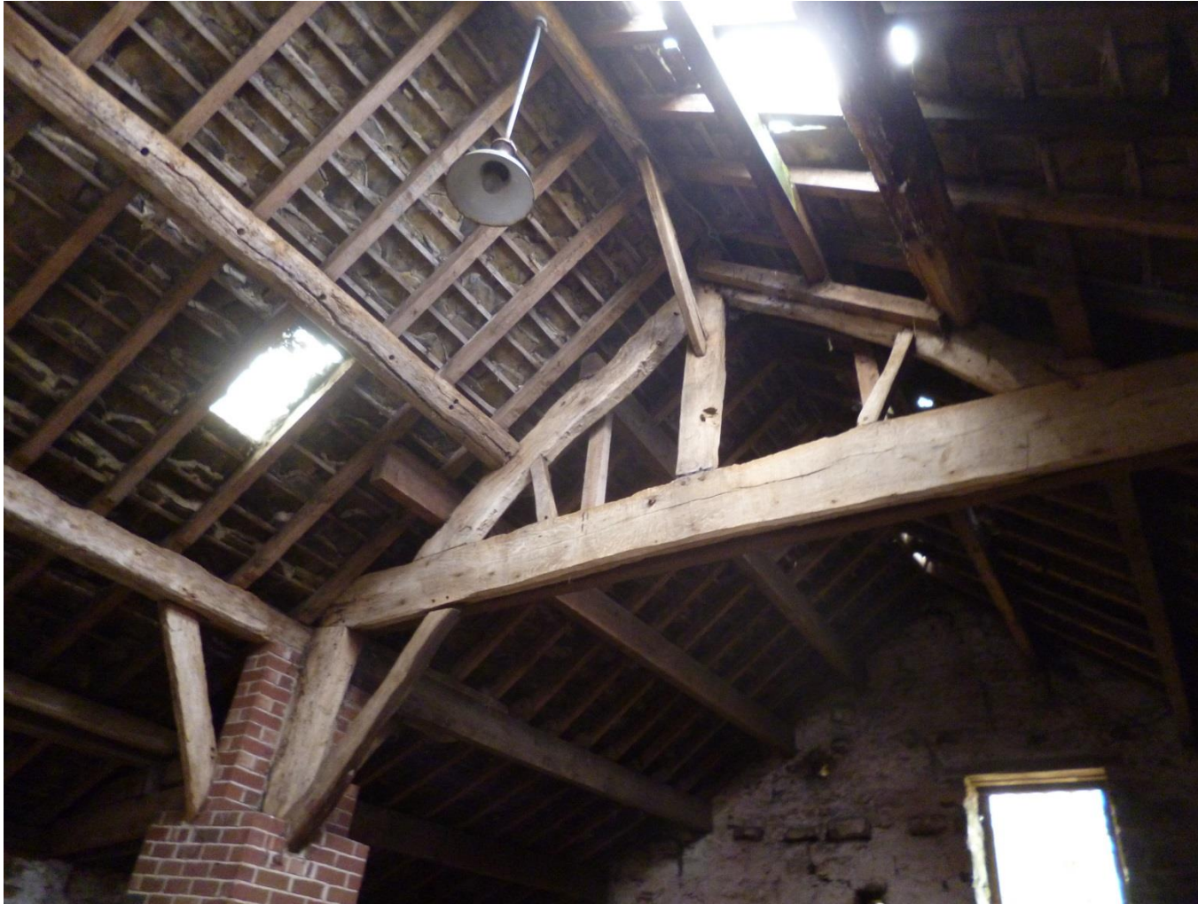
Figure 8: The barn, truss 1, photograph taken from the south
