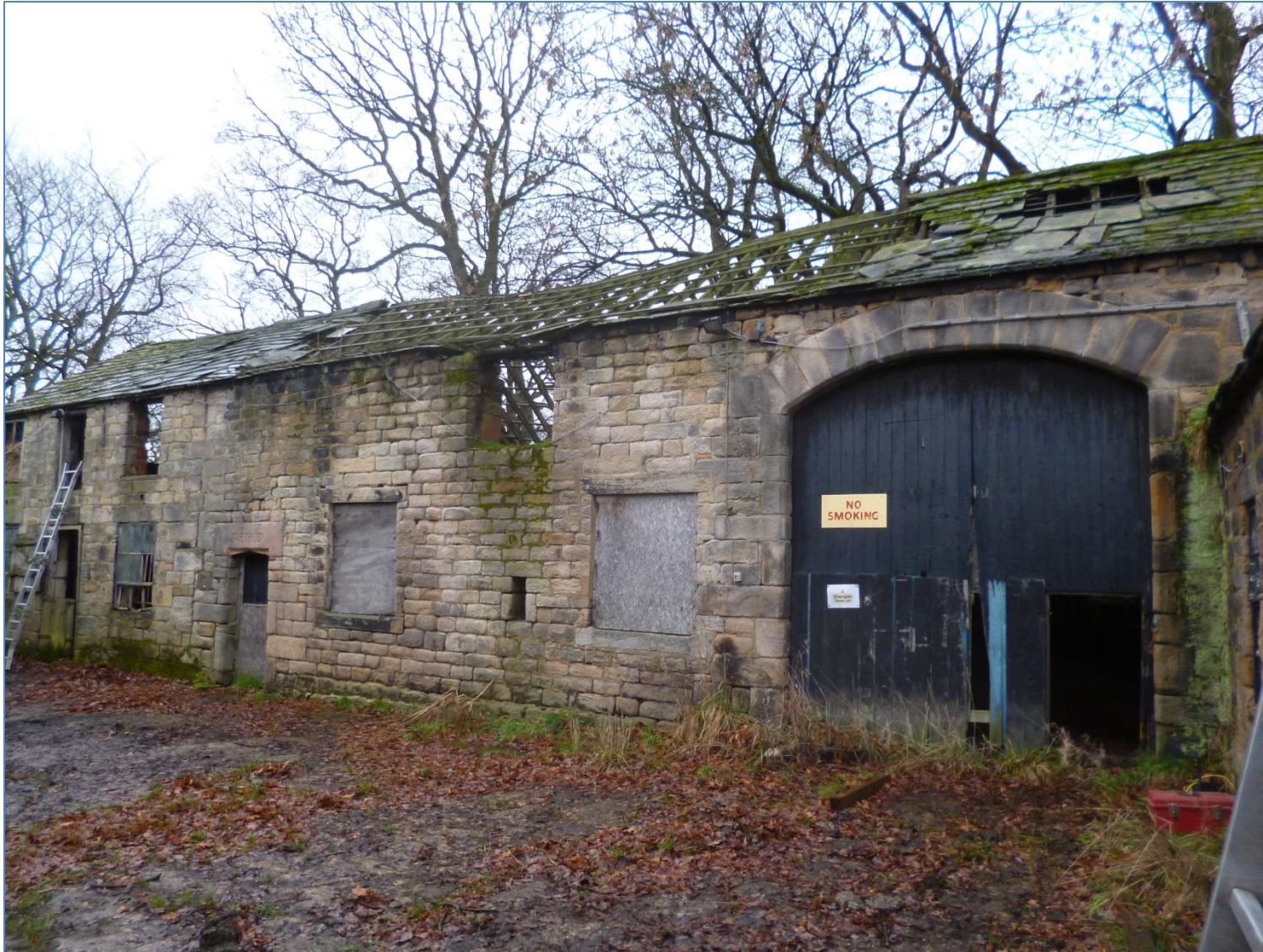
Figure 7: The barn, photograph taken from the east
