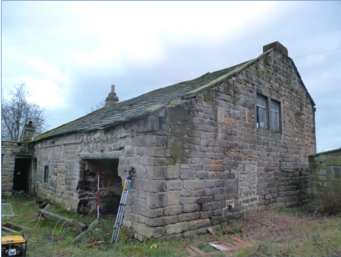
Figure 5: The rear of the former farmhouse, photograph taken from the north-west
