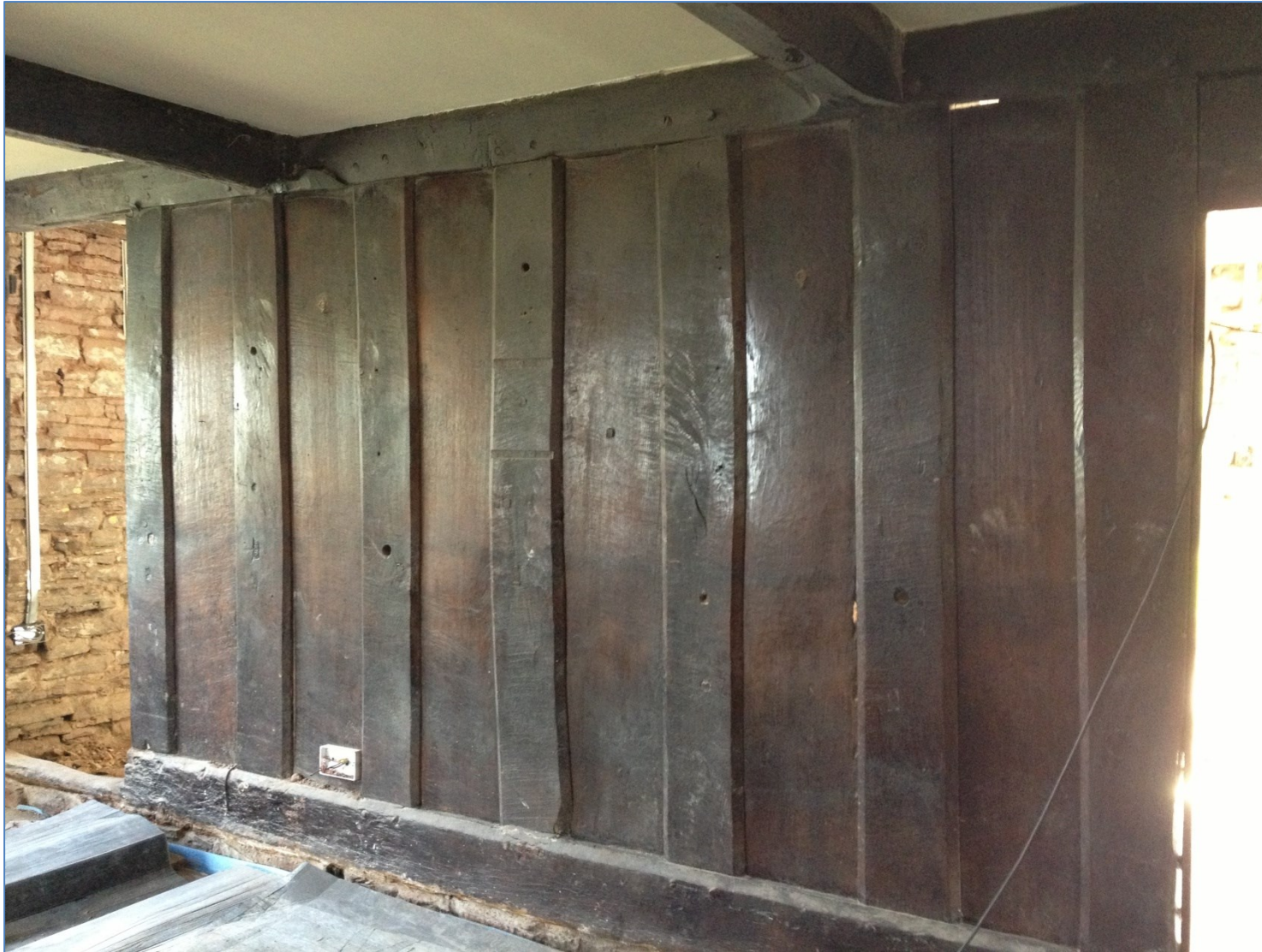
Figure 4: Plank and muntin screen
