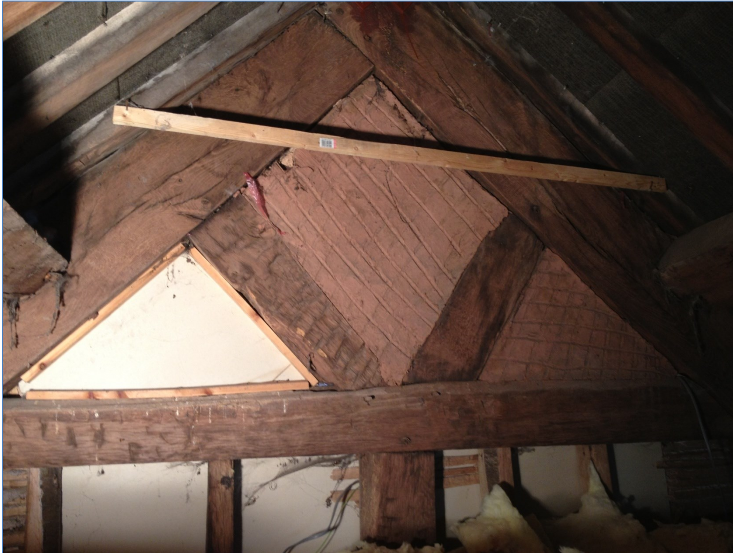
Figure 6: Truss 2 (photograph taken from the north)
