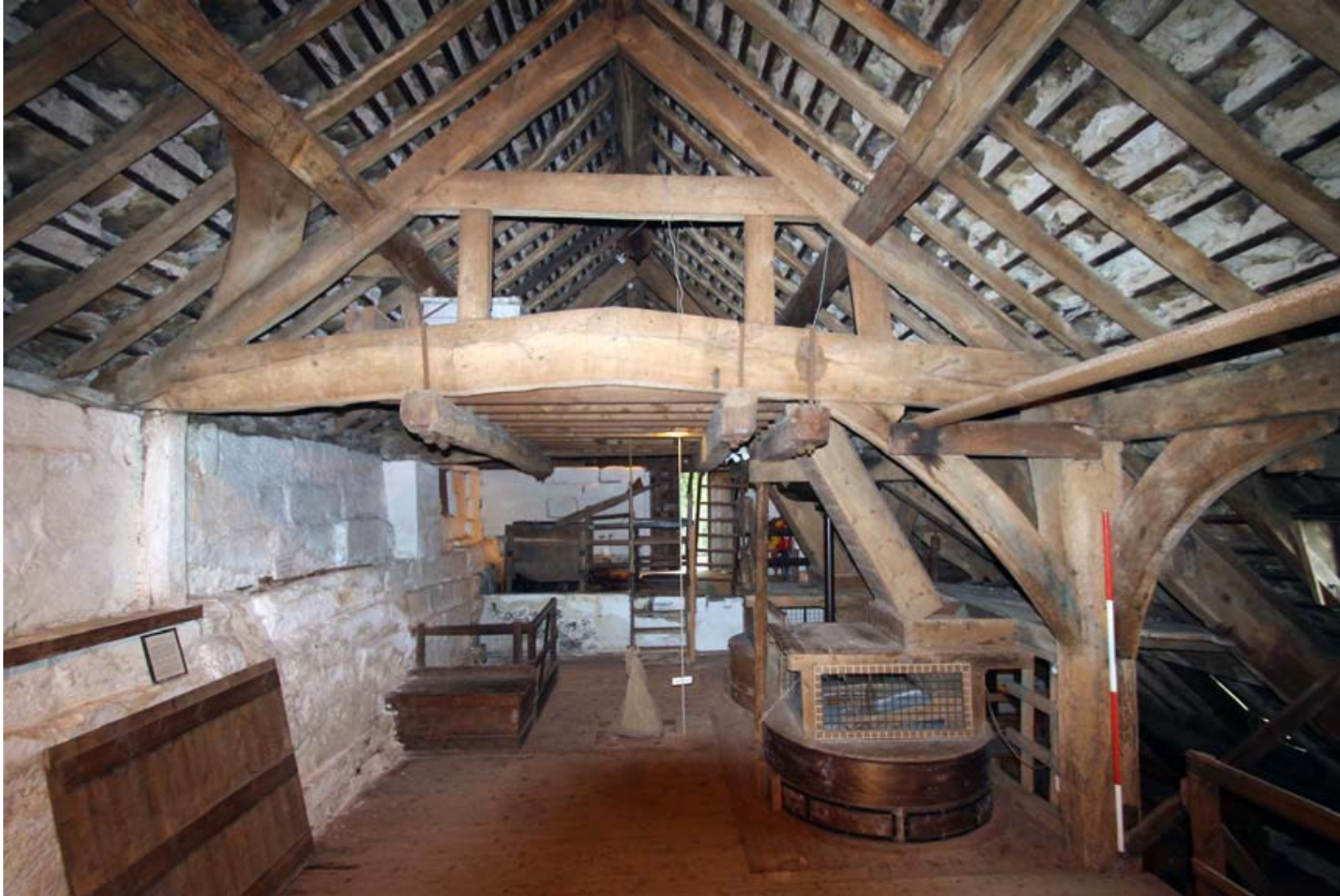
Figure 5: Upper mill, upper /roof level, viewed from north (Matrix Archaeology)
