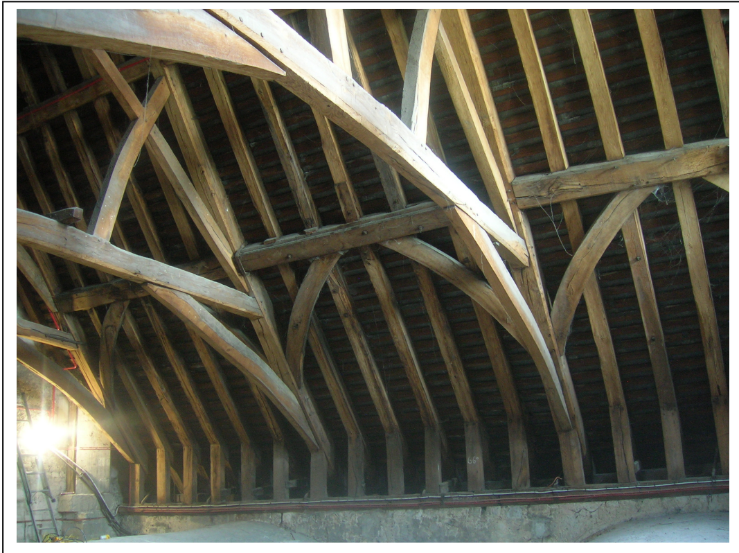
Figure 4a/b: Views of the roof to the north-west transept
