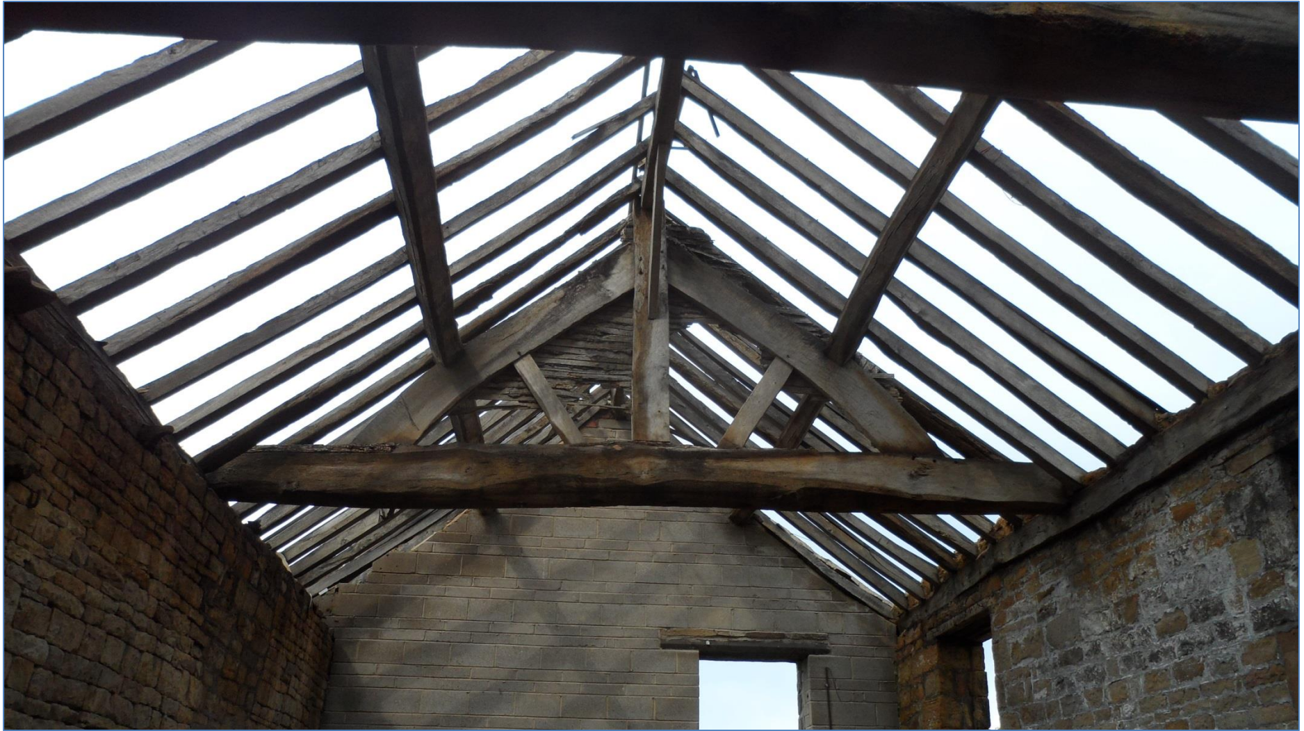
Figure 7: The mistal, truss 1, photograph taken from the south-west
