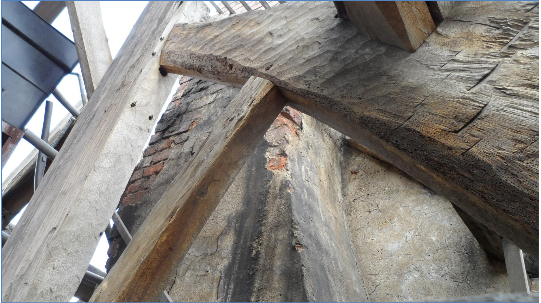
Figure 8: The cottage, east principal rafter of truss 6 with adze marks
