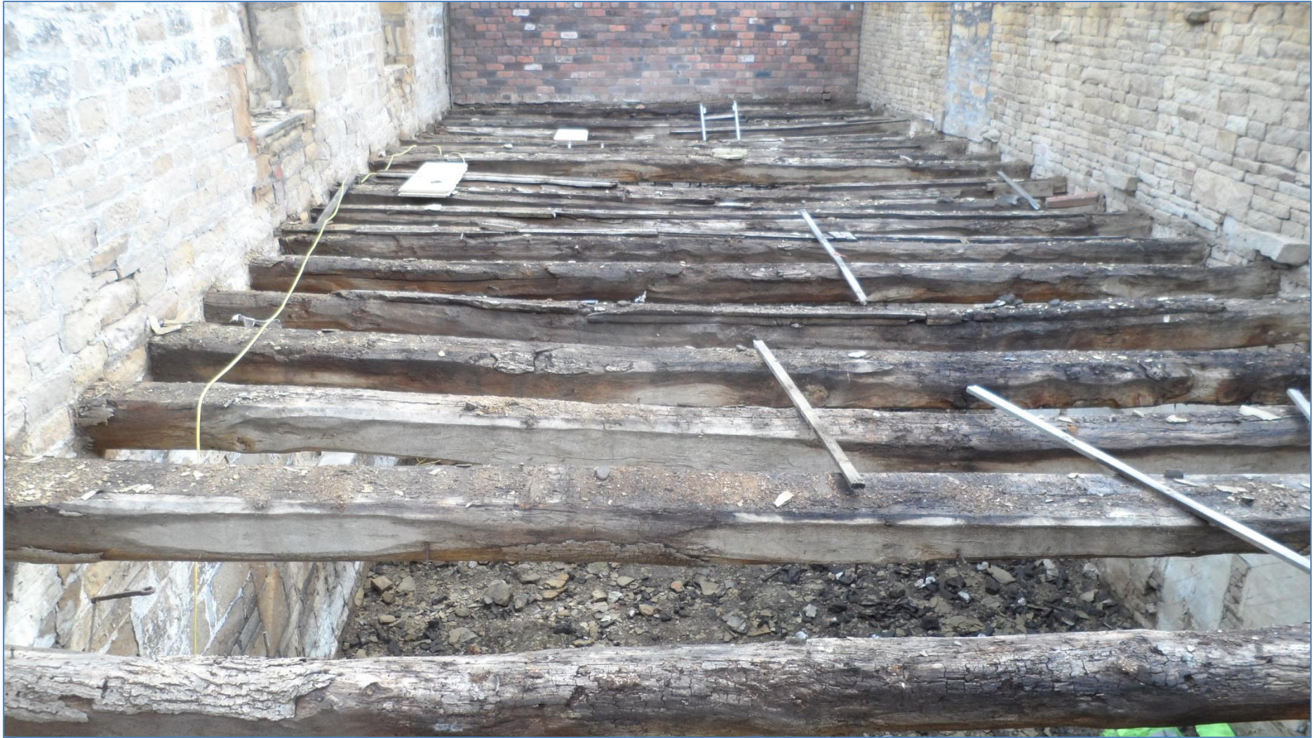
Figure 9: The mistal, first-floor frame, photograph taken from the north-east
