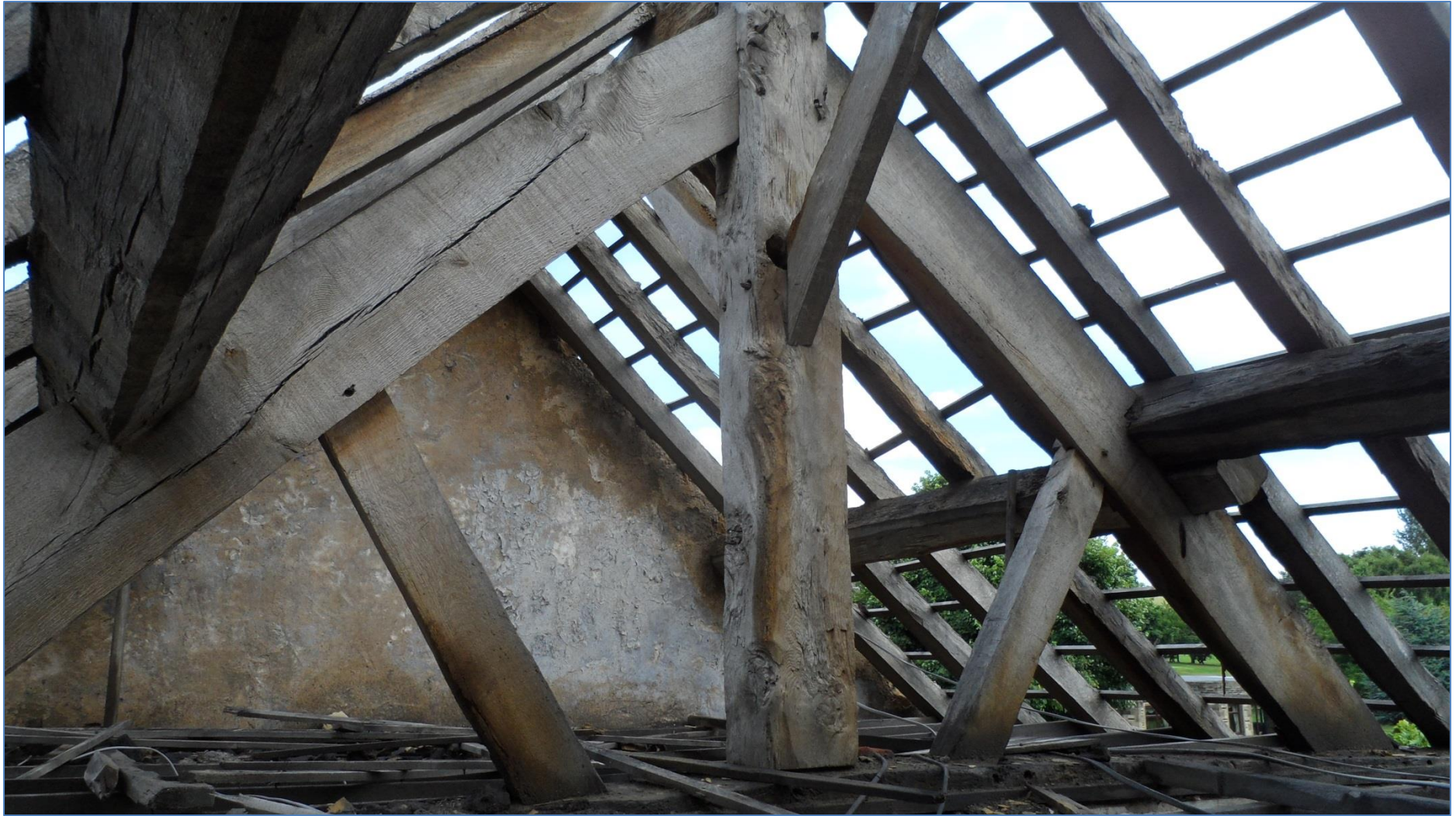
Figure 6: The cottage, truss 5, photograph taken from the south-west
