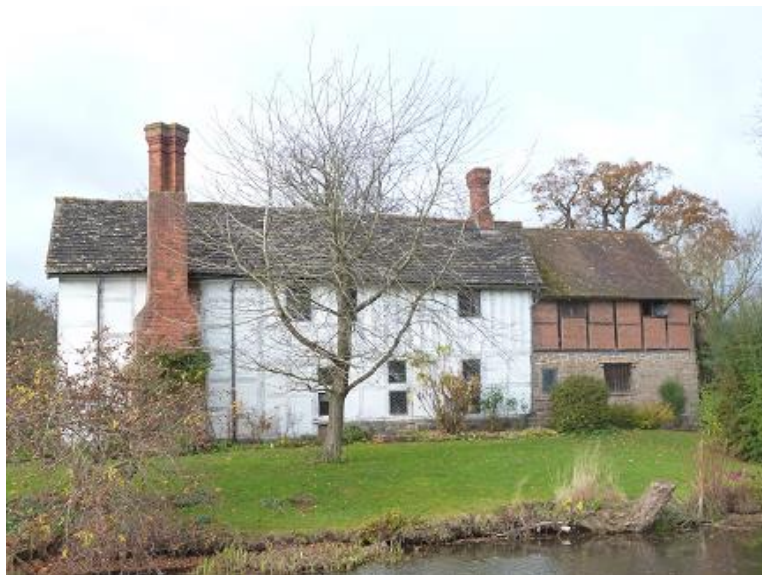
Figure 2a–c: Views of base cruck open hall (top), exterior from south showing hall and south end of cross-wing (middle) and from the east showing cross-wing and extension (bottom)
