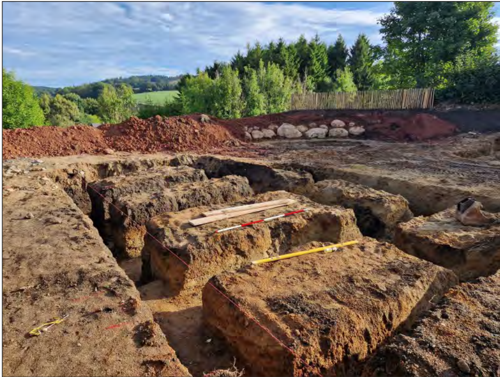
Pl. 6 General view of foundations at northern end of site showing increasing depth of topsoil (1001). 2m scale. Looking northeast.
