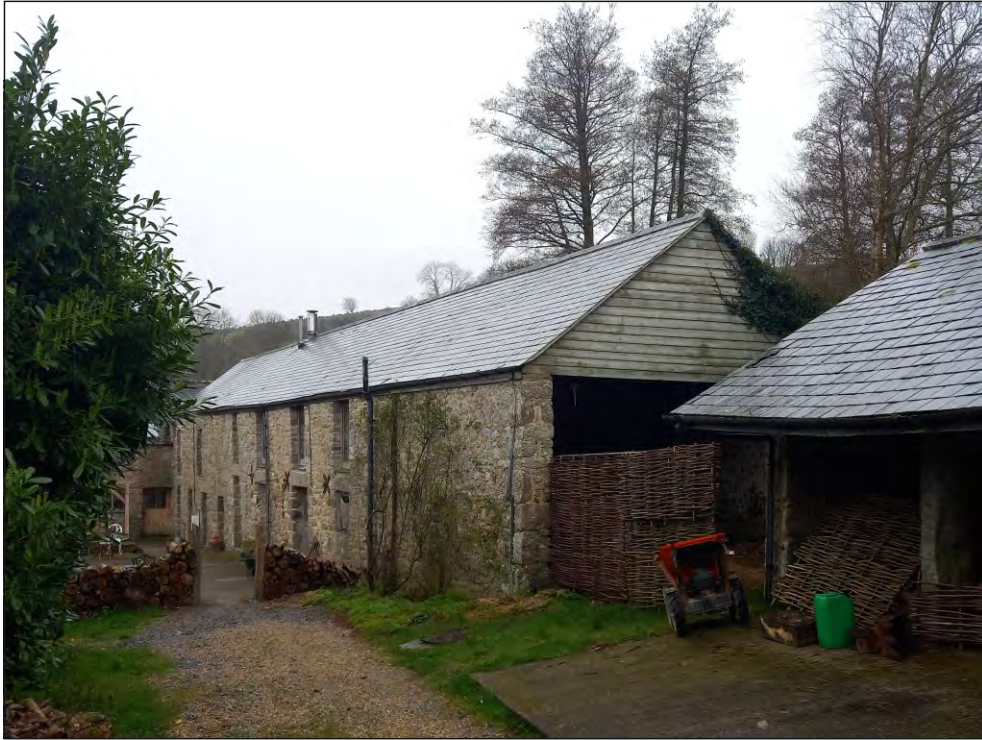
Pl. 1 General view of Southcombe Barn. Looking southwest.
