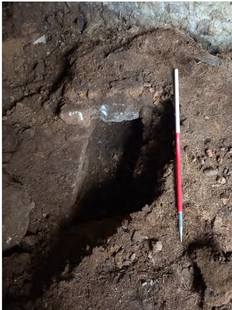
Pl. 2 General view of drain 102. 1m scale. Looking west.
