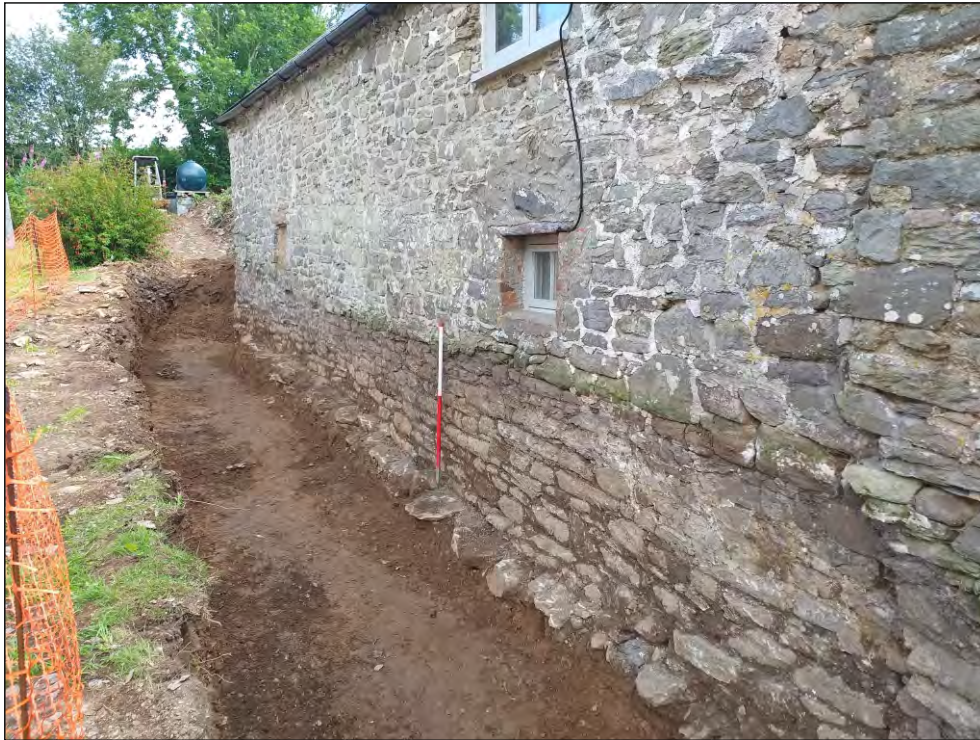
Pl. 3 General view of shallow stone rubble foundation (106) of Church Cottage. 2m scale. Looking east.
