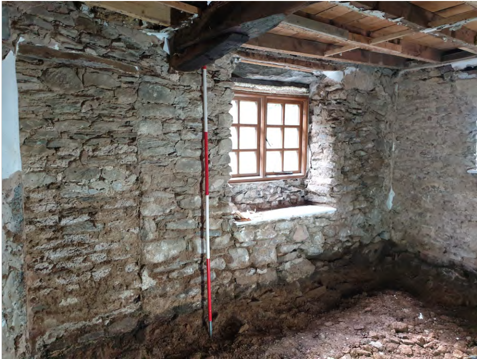
Pl. 7 General view of living-room showing beam supported with wooden shoe following rebuilding of southeast corner of building in the late 19th century. 2m scale. Looking south.
