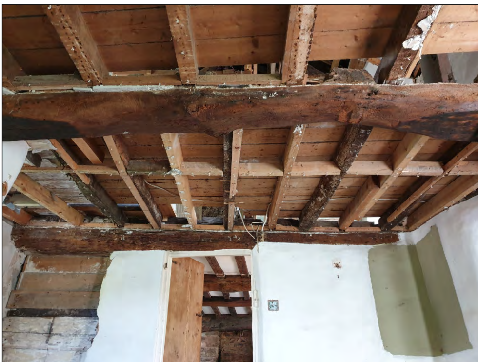
Pl. 10 General view of beam. Looking northeast.
