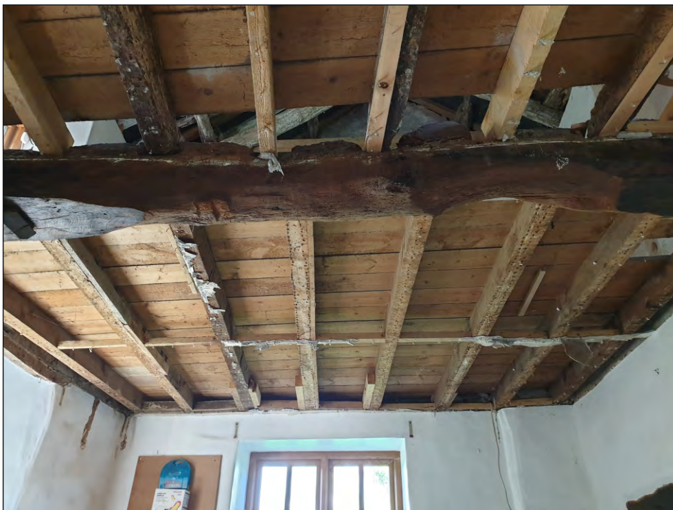
Pl. 9 General view of beam. Looking southwest.
