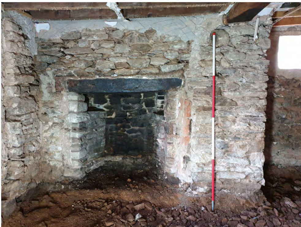
Pl. 12 General view of lateral fireplace showing late 19th century narrowing of opening. 2m scale. Looking northwest.
