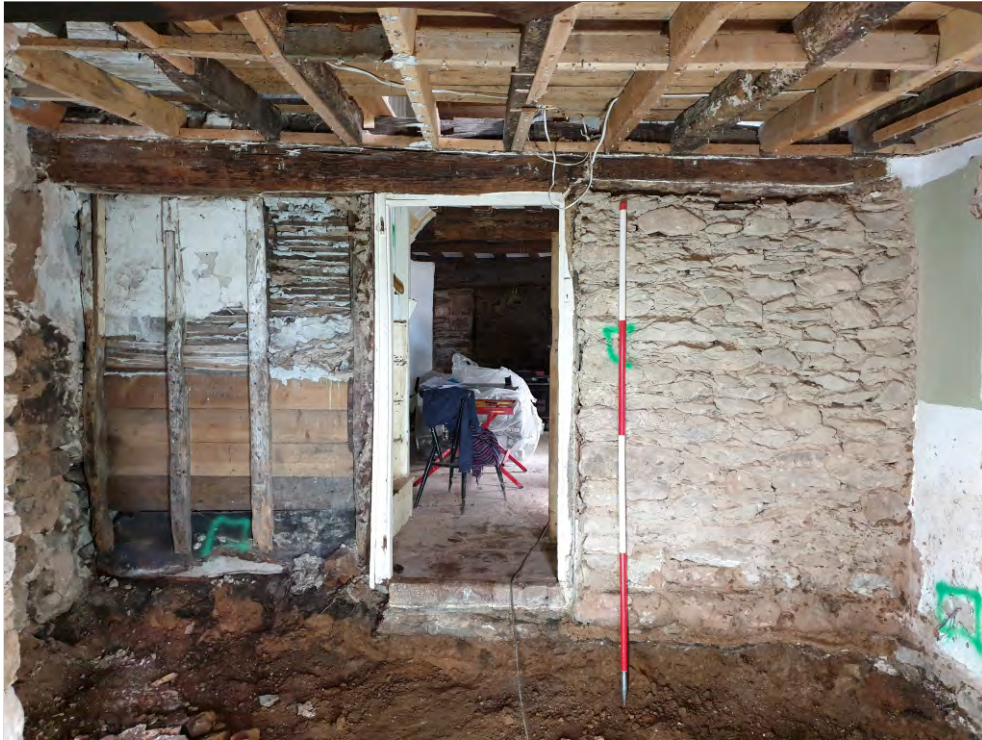
Pl. 11 General view of passage screen. 2m scale. Looking northeast.
