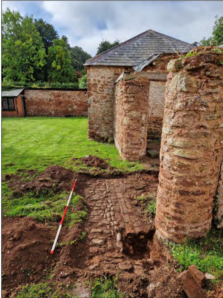
Pl. 25 General view of Trench 1 showing cobbled yard surface (103), brick drain (102) and cobbled surface (101). 2m scale. Looking southwest.
