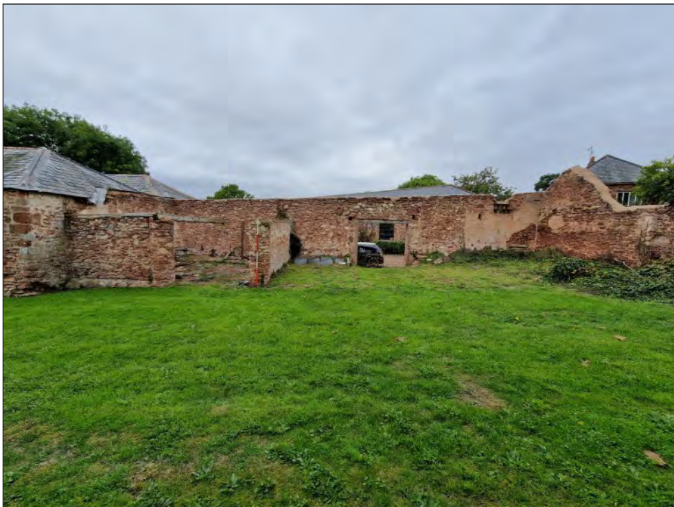
Pl. 6 General view of the linhay on the western edge of the stock yard. 2m scale. Looking west.
