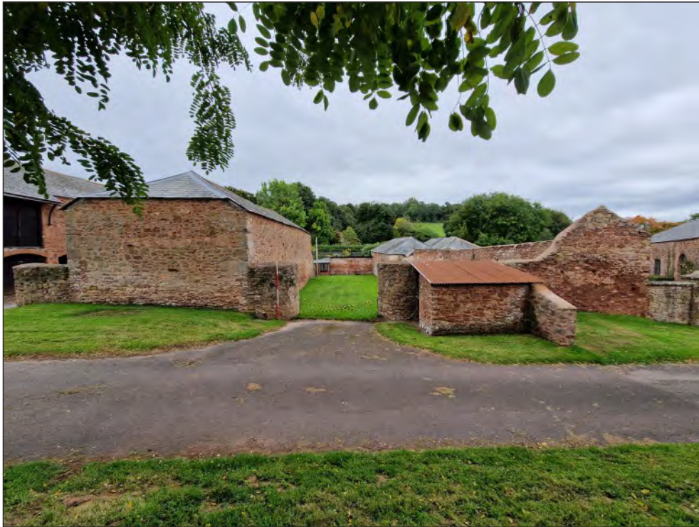
Pl. 5 General view of the stock yard with the linhay to the right. 2m scale. Looking southwest.
