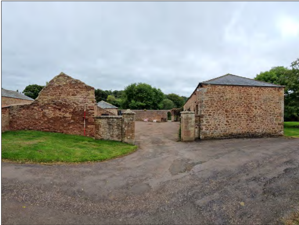
Pl. 17 General view of the stable yard showing the linhay (left), coach house (centre background) and stable (right). 2m scale. Looking southwest.
