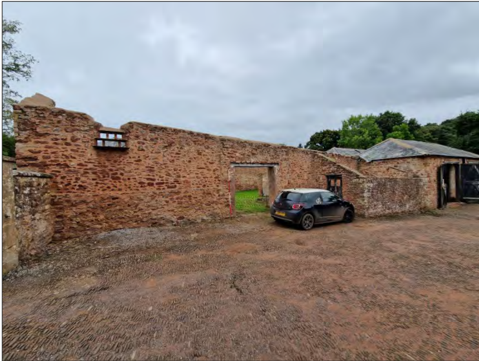
Pl. 19 General view of the linhay and coach house. 2m scale. Looking southeast.
