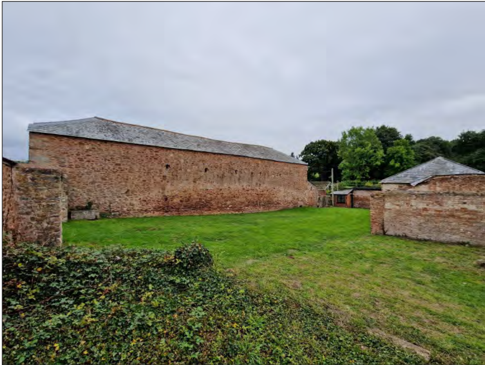
Pl. 15 General view of the stock yard showing the stables, the pig buildings (centre right) and the coach house (right). 2m scale. Looking southeast.
