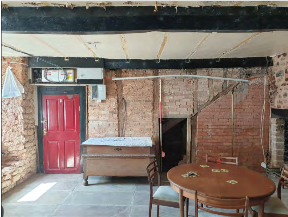
Pl. 7 General view of northwestern timber studwork late 18 th - or early 19 th -century partition showing position of former medieval partition (centre) and blocked doorway (right). 2m scale. Looking northwest.
