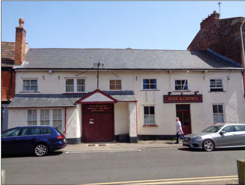
Pl. 1 General view of the south range of the Rose and Crown. Looking northeast.
