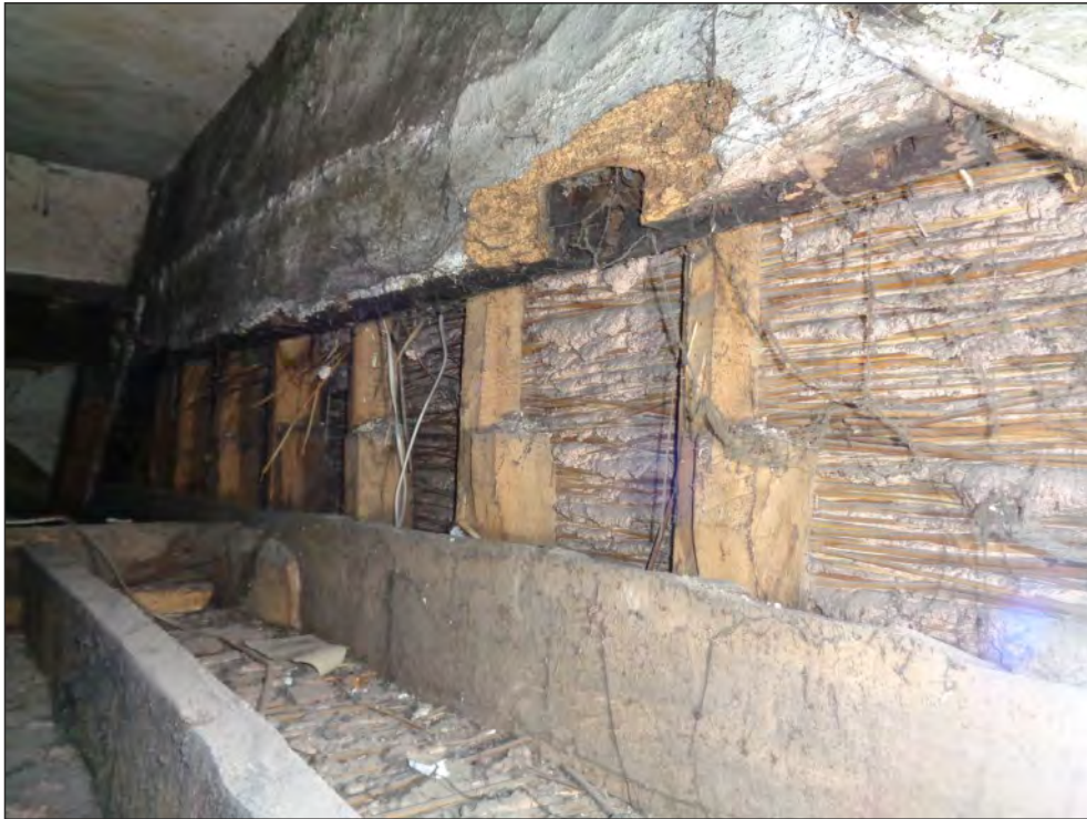
Pl. 23 Close-up of the eastern elevation of the partition between the former hall and inner room showing smoke staining. Looking west.
