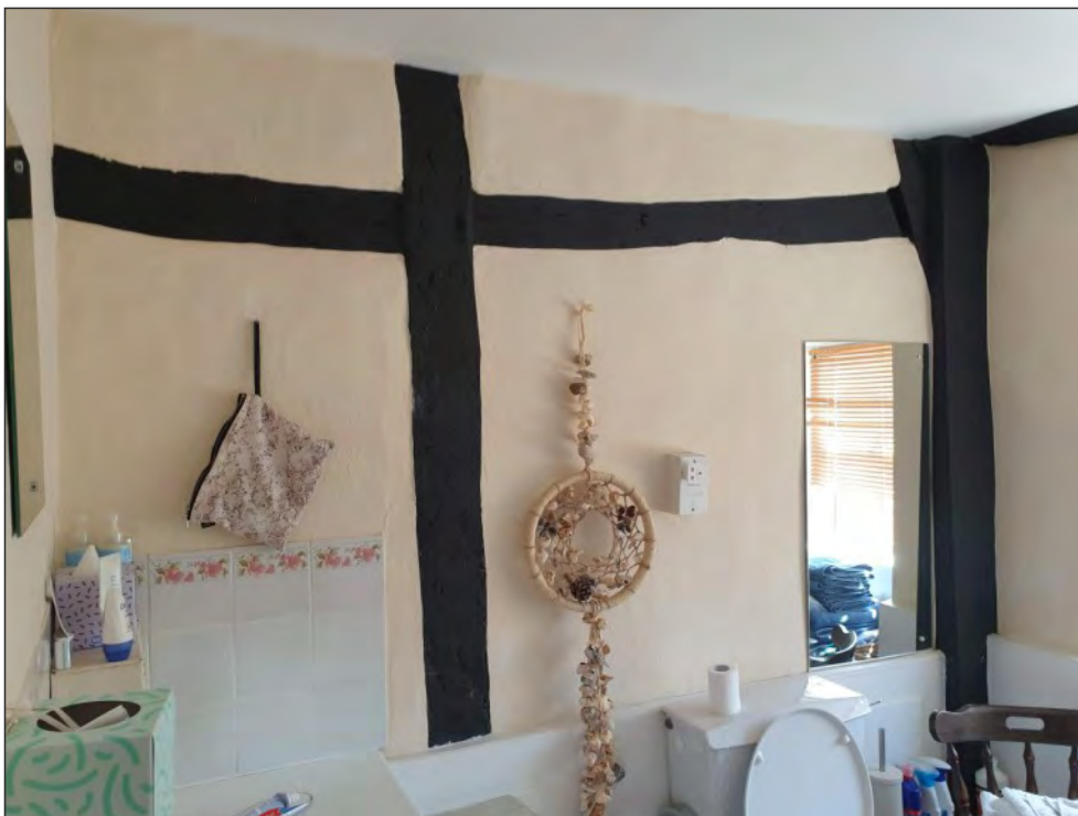
Pl. 15 General view of the full height timber and plaster partition on the east side of room F19. Looking south.
