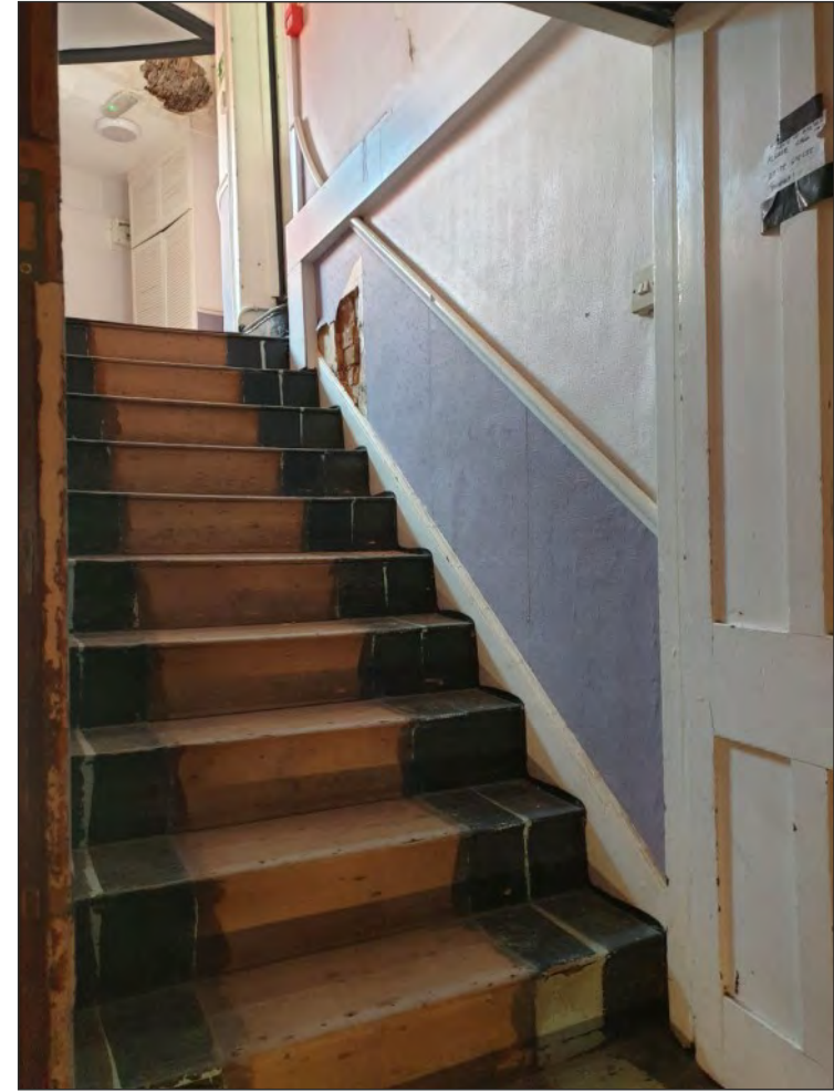
Pl. 6 General view of the main staircase. Looking northeast.
