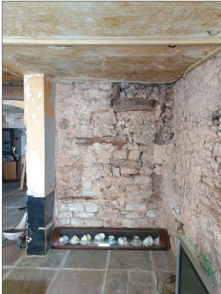
Pl. 14 General view of two small window embrasures rising with a former corner stair. Looking northeast.
