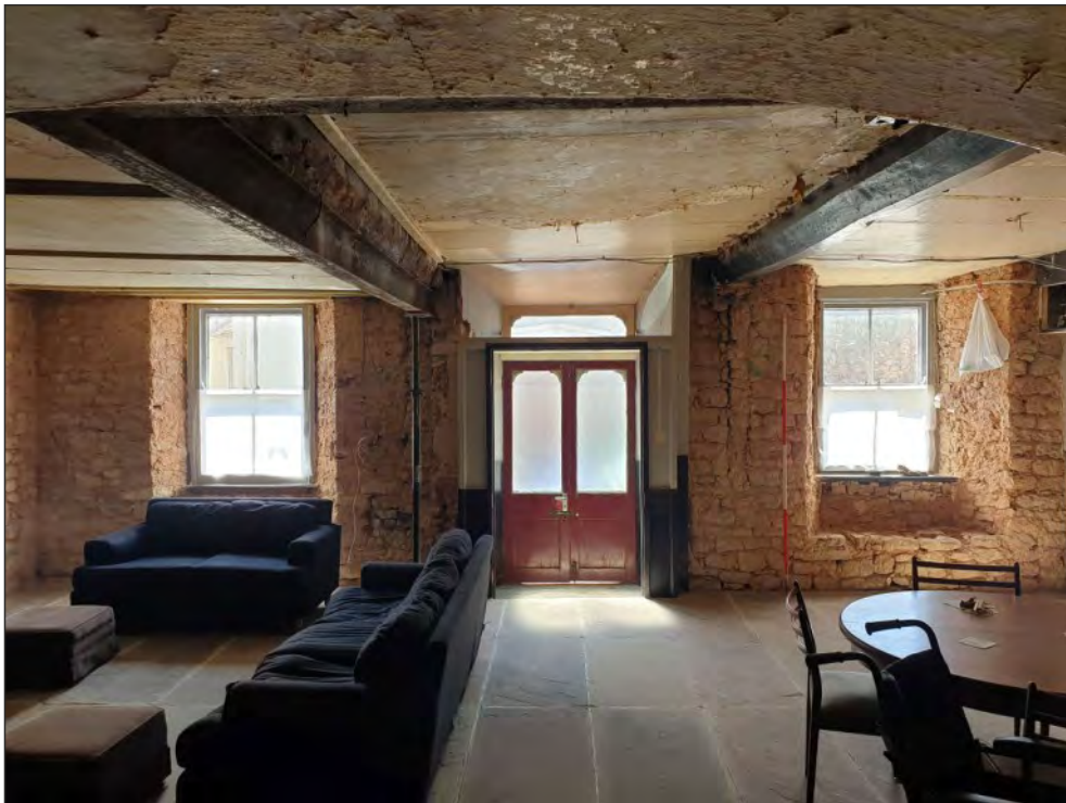
Pl. 12 General view of the south elevation of room G01 showing the remains of the infilled cruck chases. 2m scale. Looking south.
