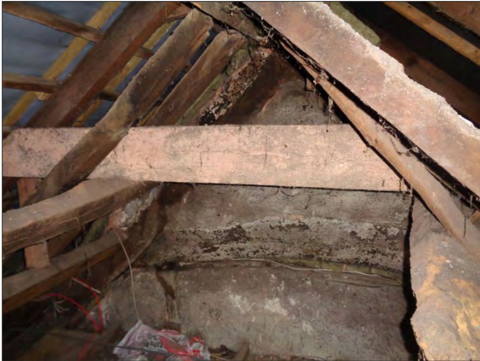
Pl. 17 Close-up of high-level cranked collar without arch bracing. Looking southeast.
