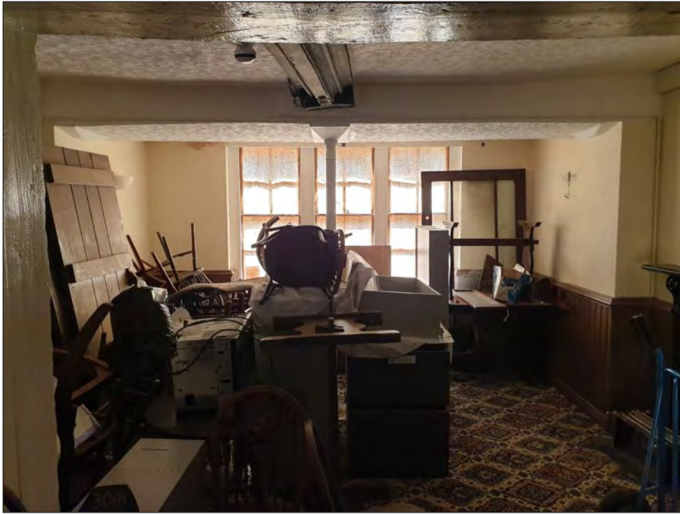
Pl. 11 General view of row of three cast-iron columns with wide bay window in the background. Looking southwest.
