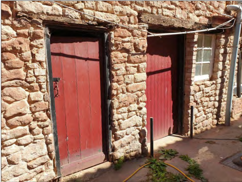
Pl. 27 General view of extension with a pair of doorways under relatively slight timber lintels. Looking southeast.
