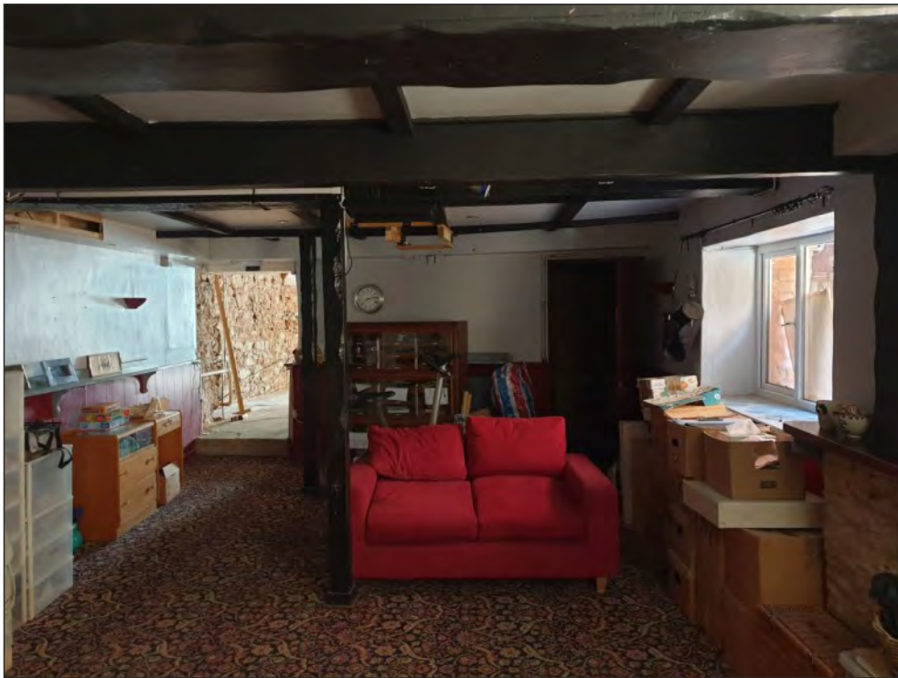
Pl. 30 General view of the rear bar with its faux-rustic boarding and supported by carefully gnarled 'olde worlde' posts reflecting the popular style of pub décor in the 1960s and 1970s. Looking southwest.
