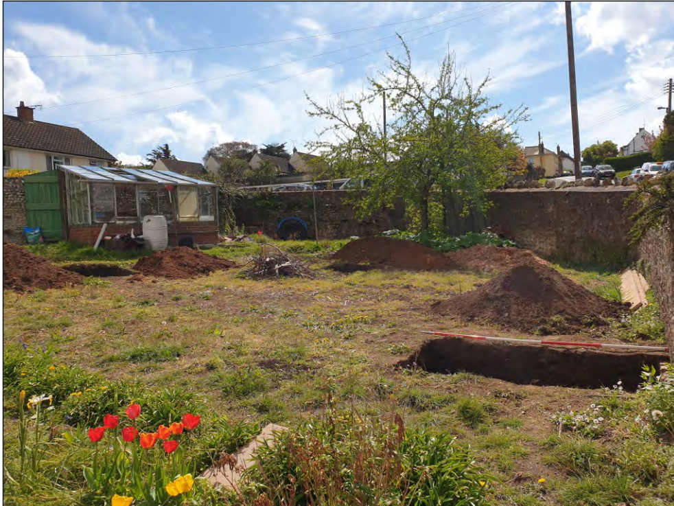
Pl. 1 General view of the proposed site showing Trenches 1-3. 2m scale. Looking southeast.
