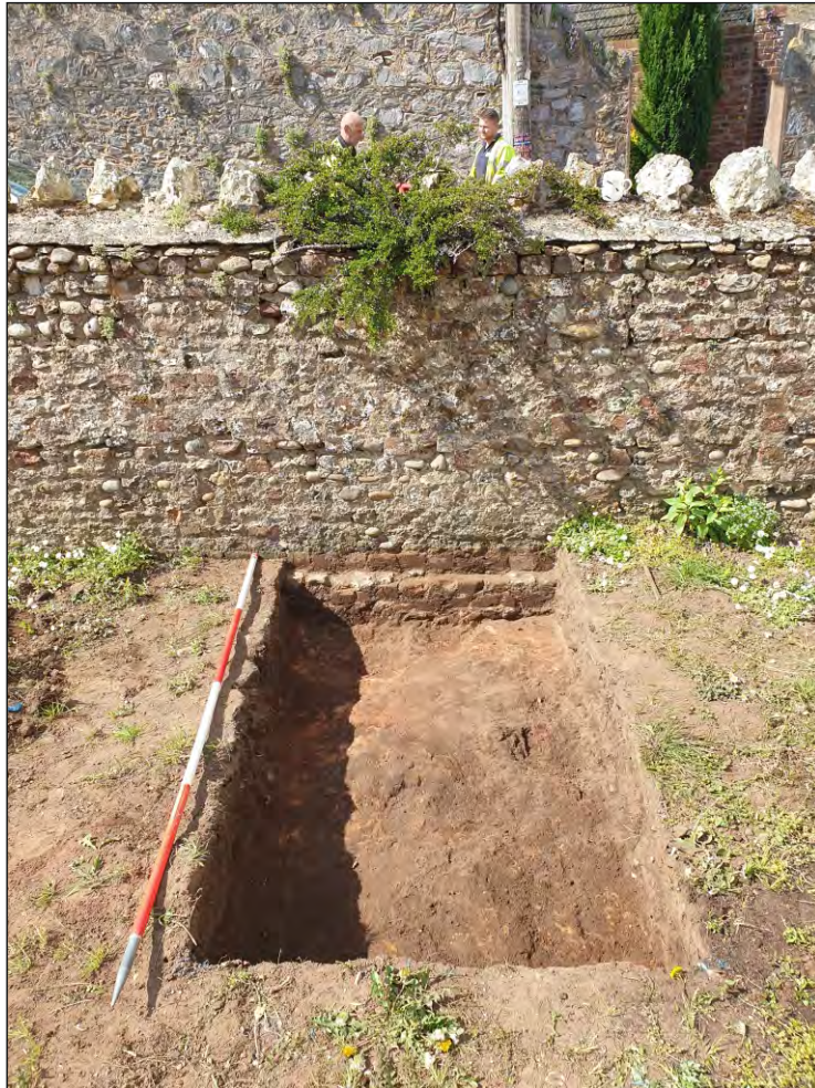
Pl. 3 General view of Trench 1 showing foundation of garden wall (102) above natural subsoil (101). 2m scale. Looking west.
