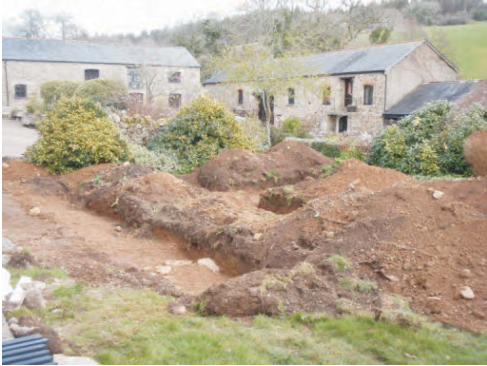
Pl 1 General view of trenching in area of Shippon. Looking northeast.
