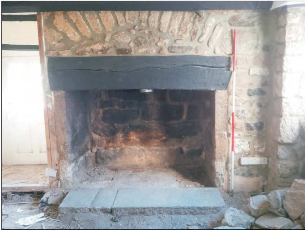
Pl. 7 General view of fireplace, Hall. 2m scale. Looking east.
