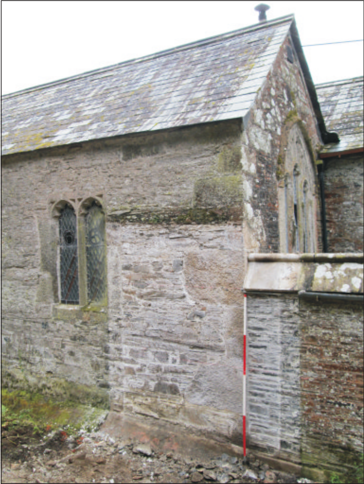
Pl. 4 General view of exposed church fabric. 2m scale. Looking southeast.
