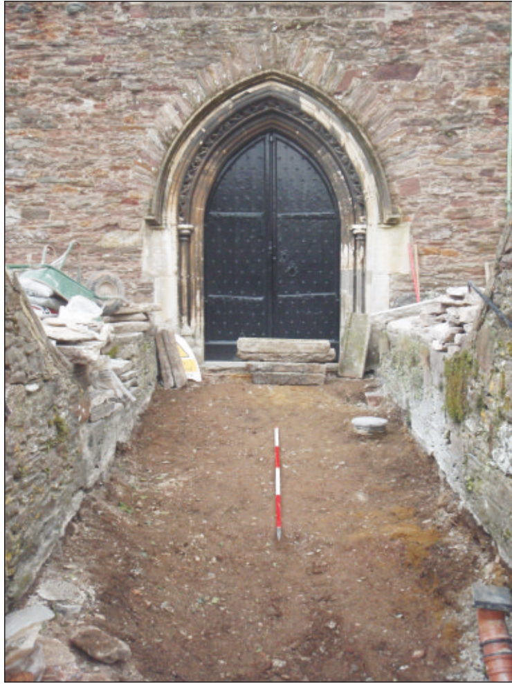
Pl. 1 General view of access ramp area. 2m scale. Looking east.
