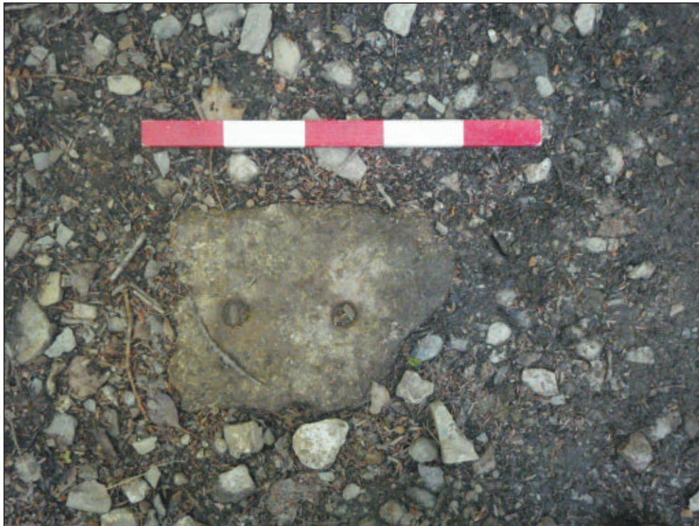
Pl. 2 Close-up of granite set showing boltholes. 0.5m scale. Looking south.
