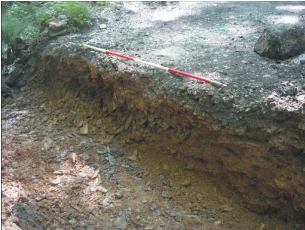
Pl. 3 Section through Plymouth-Dartmoor Railway. 2m scale. Looking southeast.
