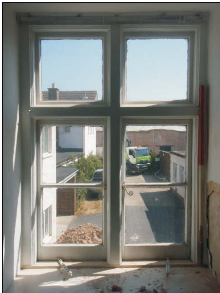
Pl. 15 General view of first floor cross windows. 1m scale. Looking northeast.
