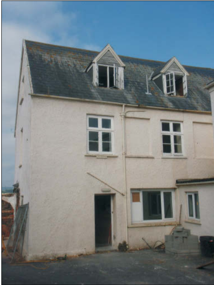
Pl. 5 General view of rear range showing C18th first floor cross windows and later blocking. Looking southwest.
