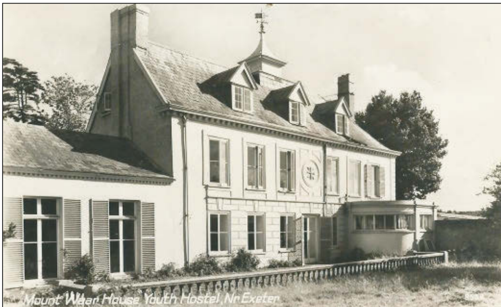
Fig. 8 Postcard showing original chimney stacks at either end of the principal range and bell tower.
