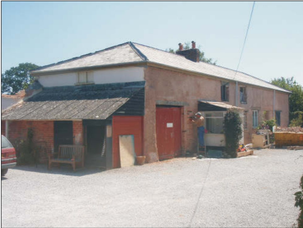
Pl. 19 General view of manager's cottage. Looking east.
