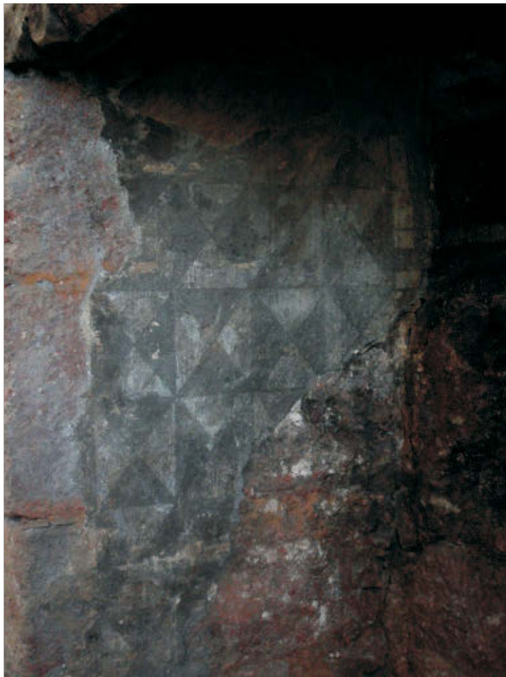
Pl. 12 Close-up of jamb showing diagonally quartered near squares. Looking south.
