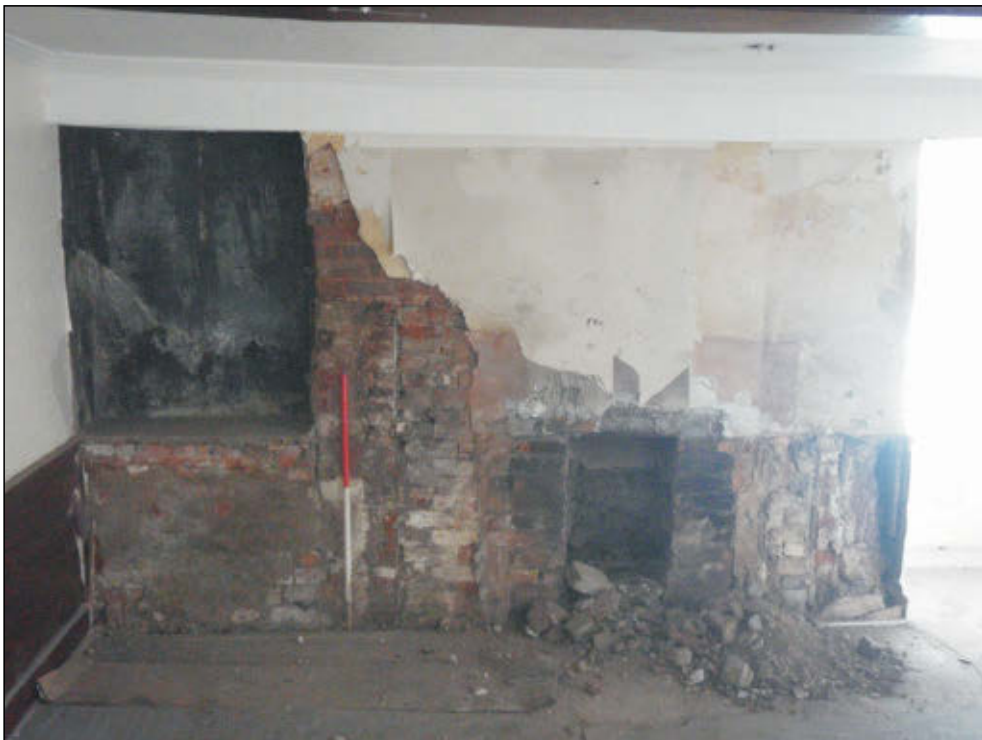
Pl. 8 General view of ground floor fireplace showing successive alterations. 1m scale. Looking southwest.
