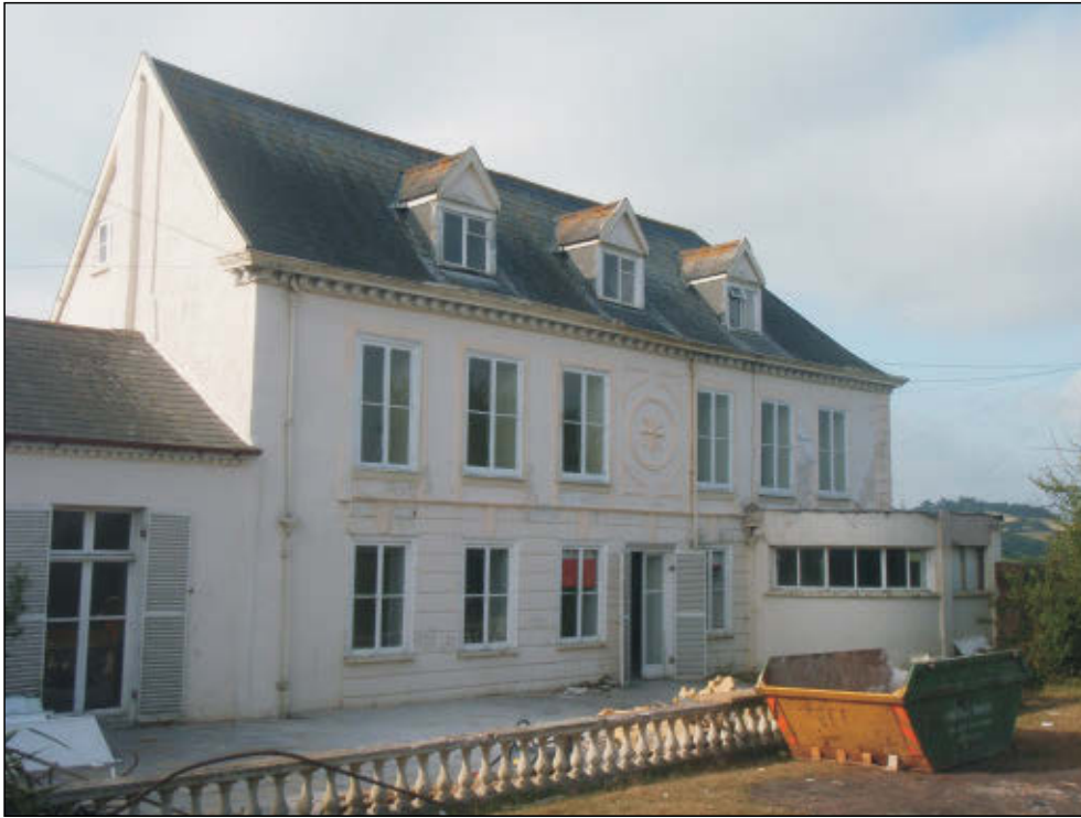
Pl. 1 General view of main building facade showing C18th stucco decoration. Looking south.
