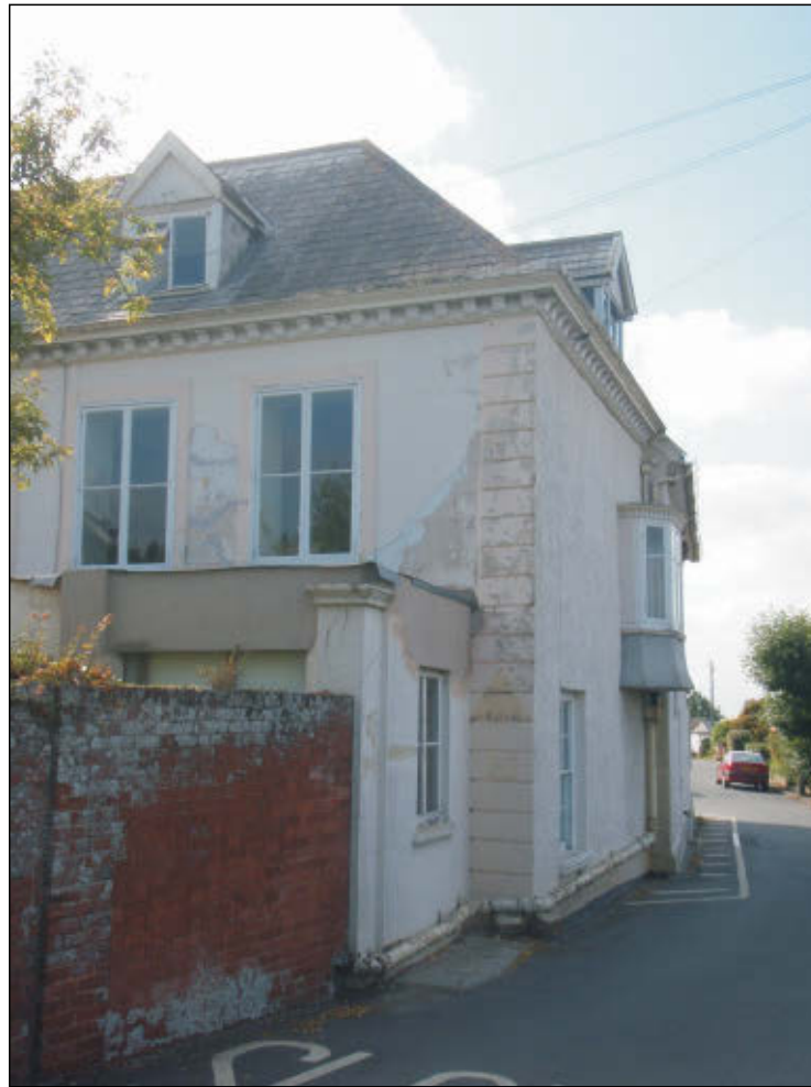
Pl. 2 Side view showing early C20th porch and C19th oriel window. Looking southeast.
