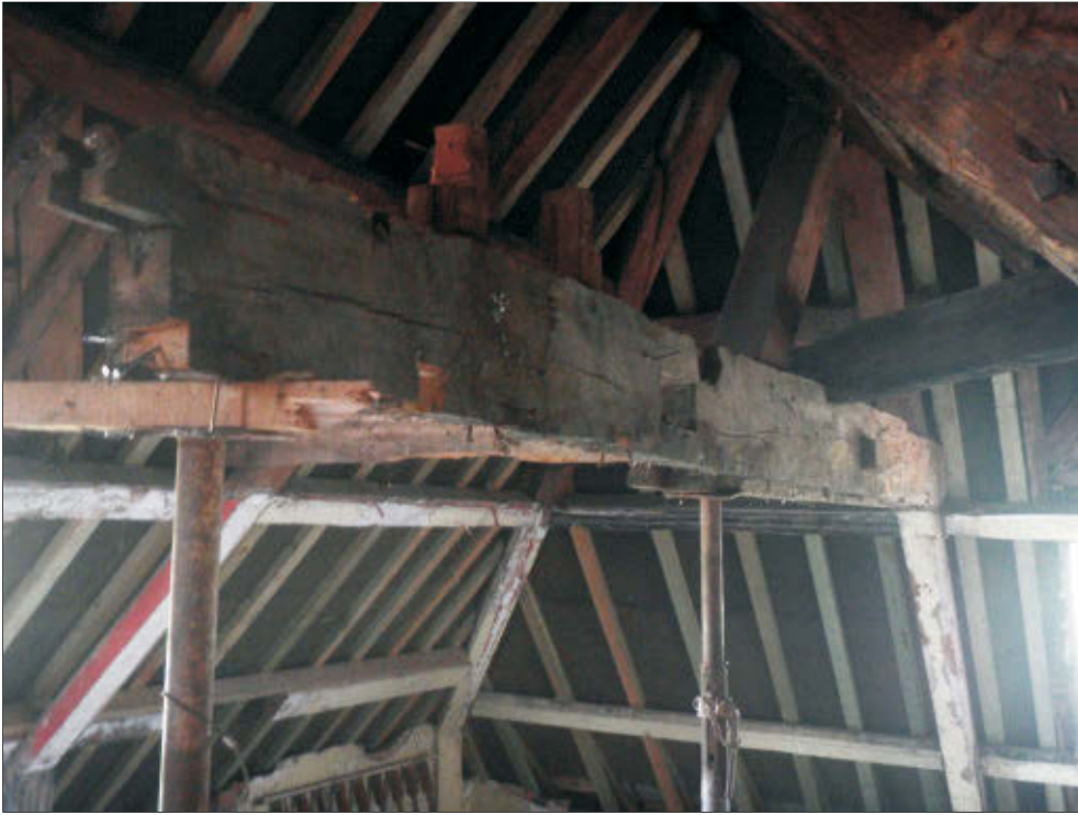
Pl. 17 General view of re-used jointed cruck truss. Looking south.
