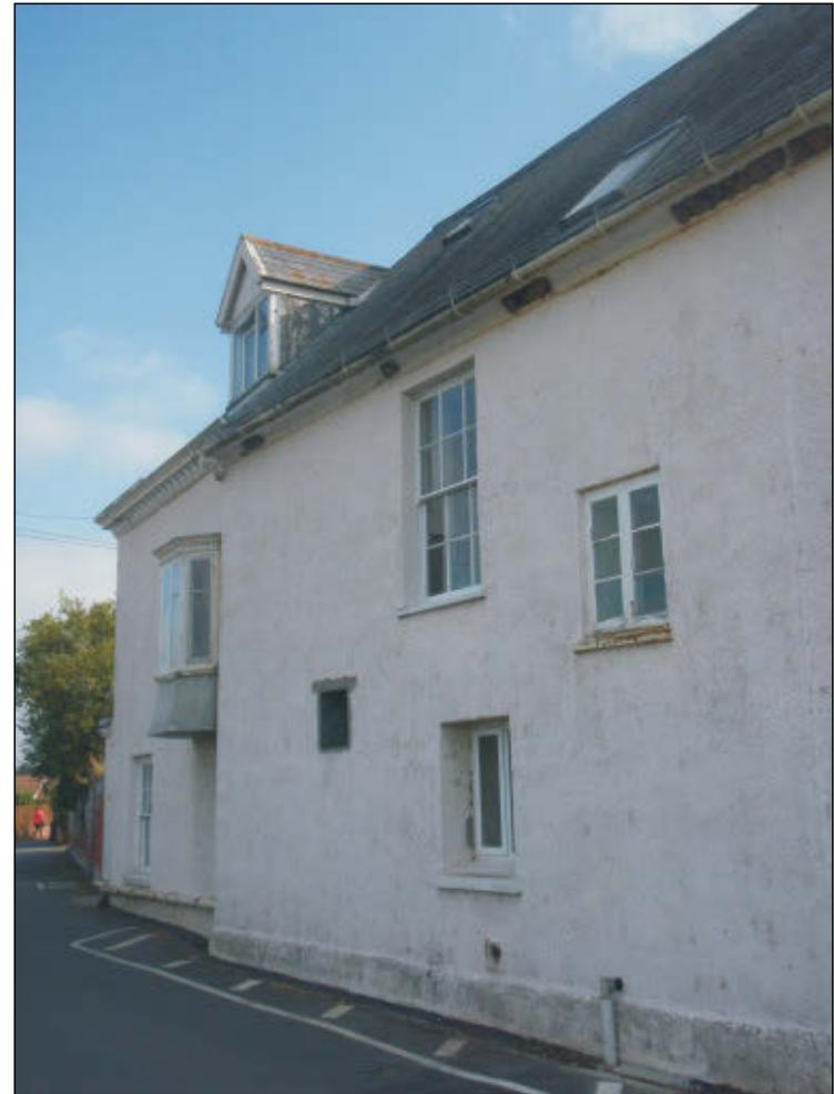
Pl. 4 Side view showing C18th-C20th windows. Looking north.
