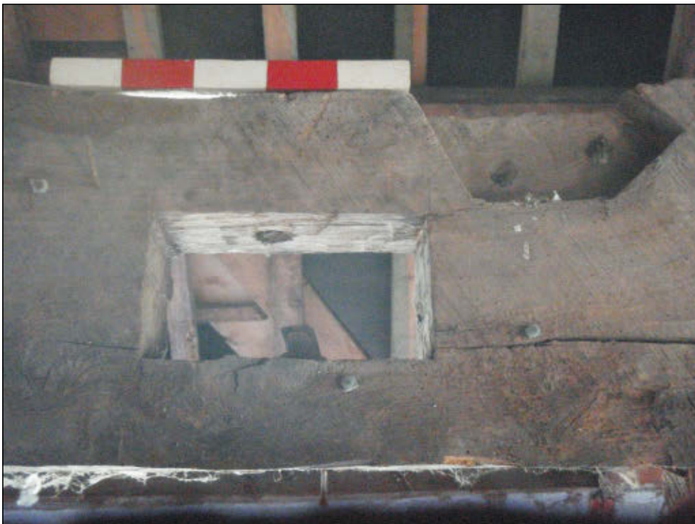
Pl. 18 Close-up of lap joint and purlin hole. 0.25m scale. Looking southwest.
