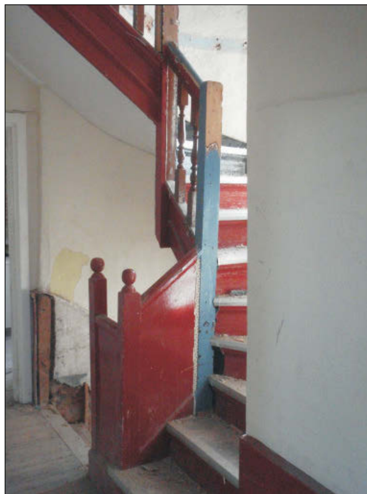
Pl. 16 General view of staircase leading to second floor. Looking east.
