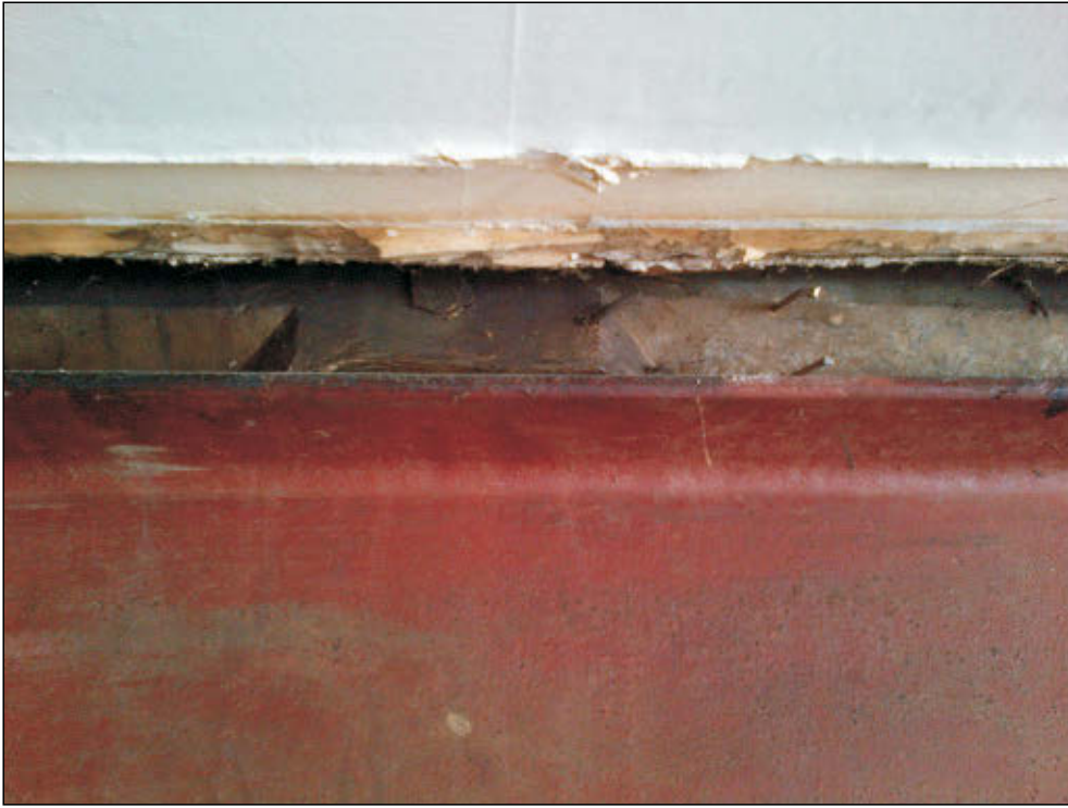
Pl. 7 Close-up view of ground floor head rail for plank and muntin screen. Looking southwest.
