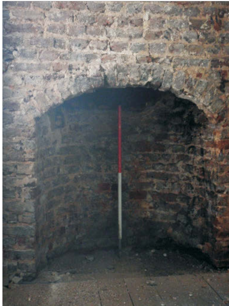
Pl. 14 Close-up of fireplace in Room F11 showing curved back and arch. 1m scale. Looking east.
