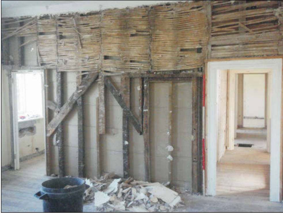
Pl. 13 General view of first floor C18th partition with blocked C19th doorway in foreground. 2m scale. Looking northeast.
