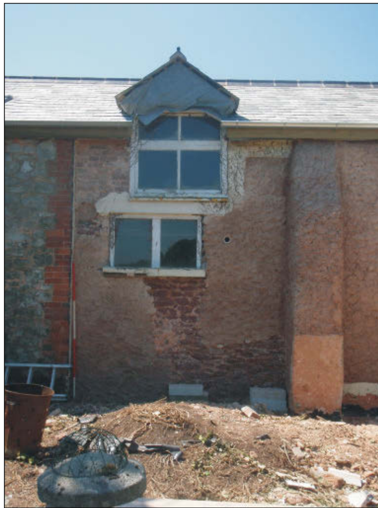
Pl. 20 General view of blocked-up barn door and C19th hayloft window. 2m scale. Looking southwest.
