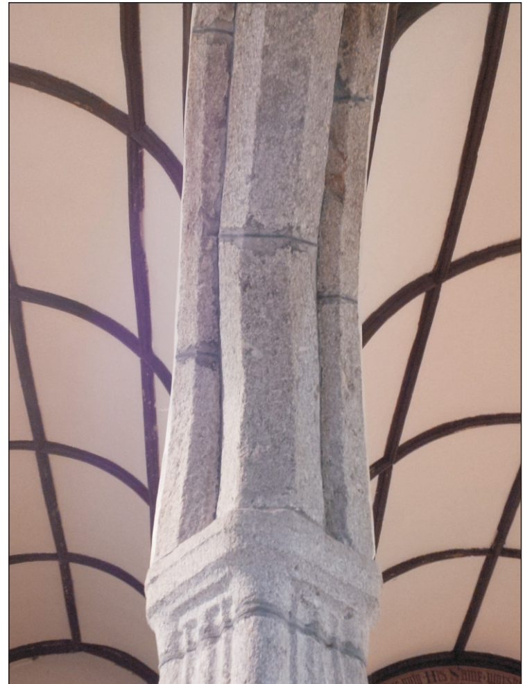
Pl. 10 Arcade: Close-up of west bay arch. Looking east.
