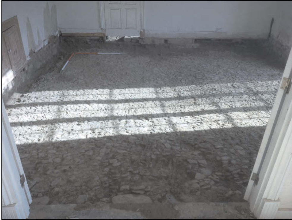
Pl. 1 General view of cobbled floor (101) in sitting room. 1m and 1m scales. Looking northeast.
