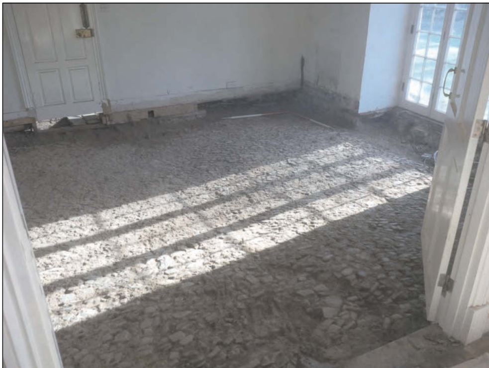
Pl. 2 General view of cobbled floor (101) in sitting room. 1m and 1m scale. Looking east.
